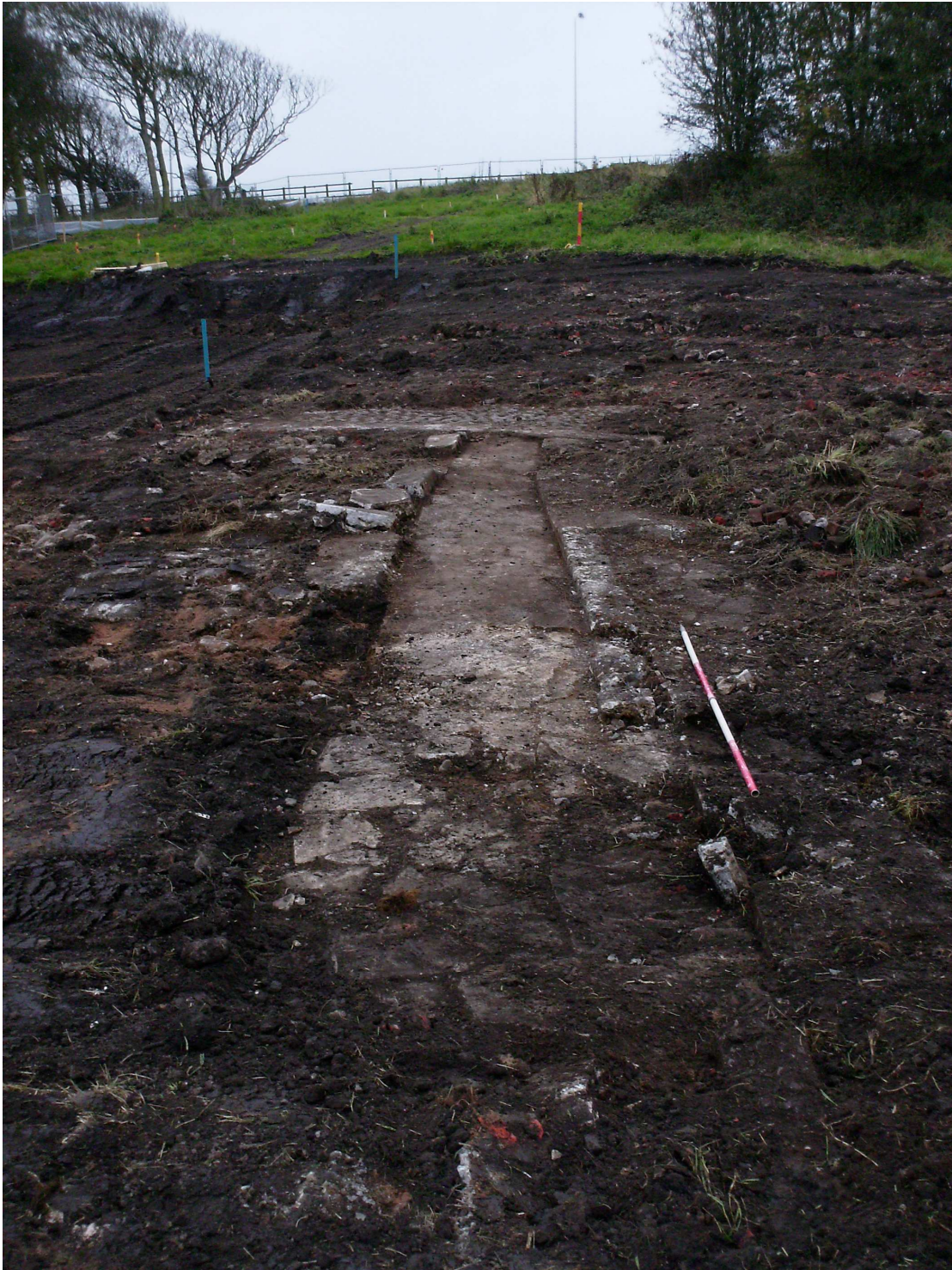
Plate 5: Concrete sluice 2004 , looking south
