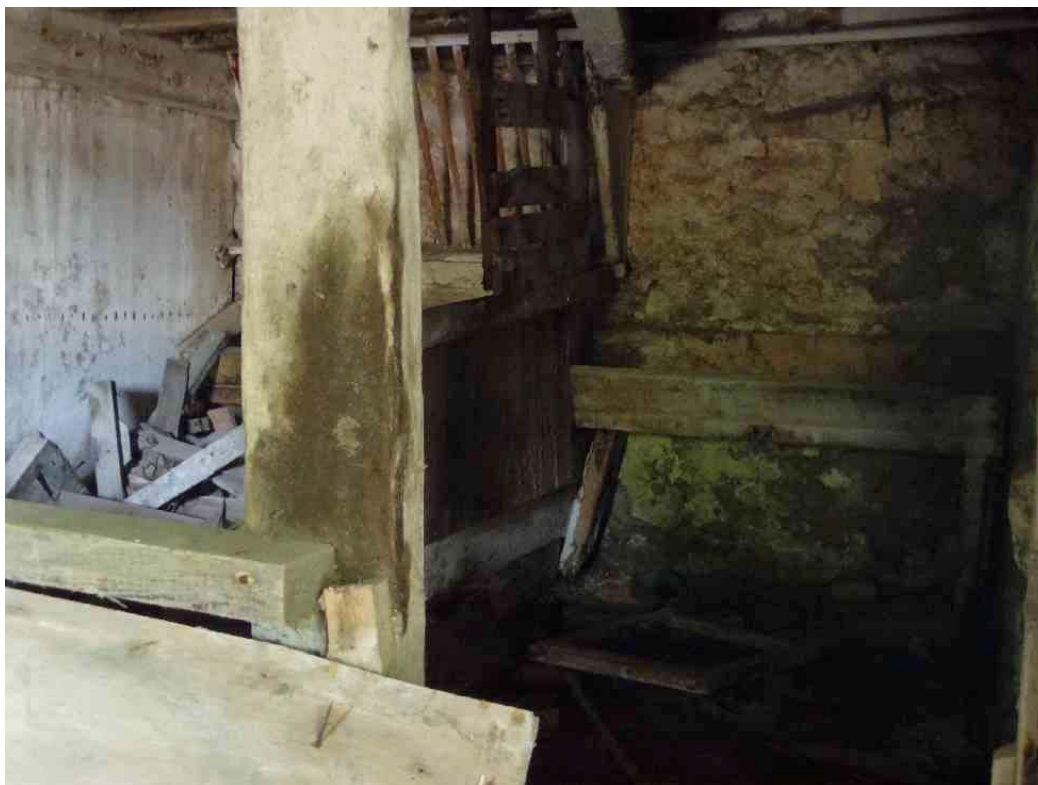
Plate 9: Detail of stables with manger on ground floor
