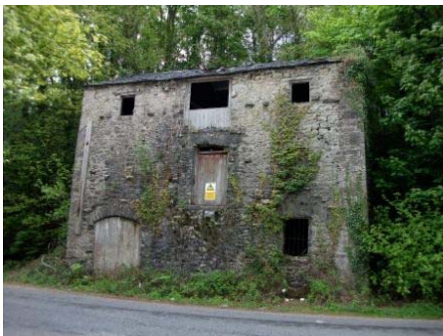
Plate 4: The front (north-west) elevation of the warehouse (Reproduced with kind permission of the Dallam Tower Estate)
