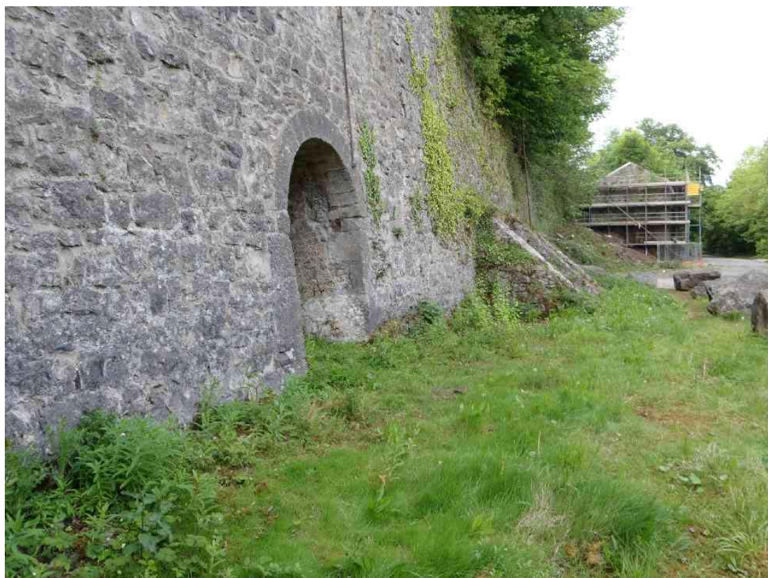
Plate 2: The warehouse as viewed from the limekilns
