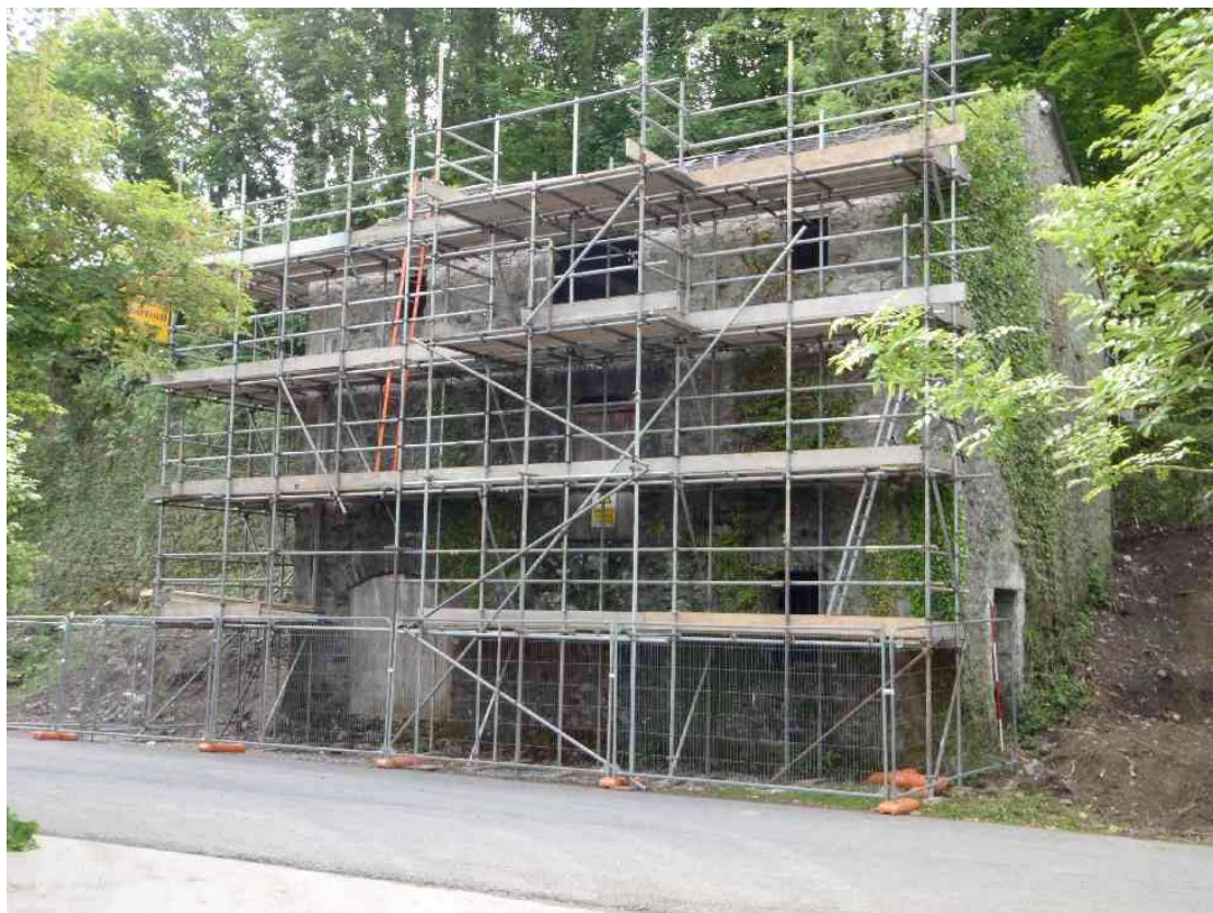
Plate 3: Scaffolding surrounded the warehouse on three sides at the time of the building investigation
