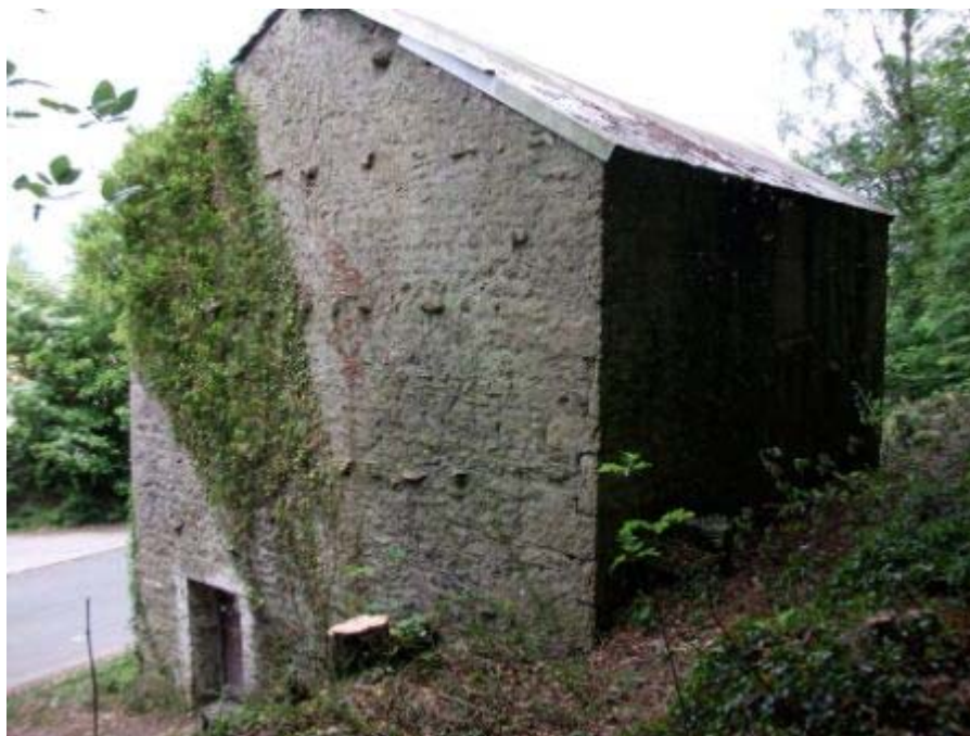
Plate 6: Detail of the through-stones in the south-west elevation (Reproduced with kind permission of the Dallam Tower Estate)
