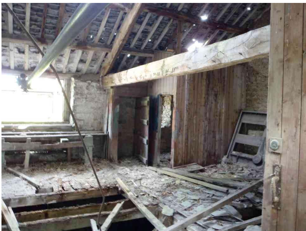
Plate 10: Office partition on second floor, with cupboard and workbench under window
