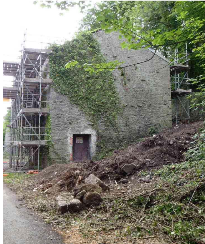
Plate 5: The south-west gable of the warehouse
