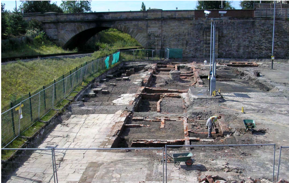
Plate 22: View along the foundations of buildings on the 'Up' Platform
