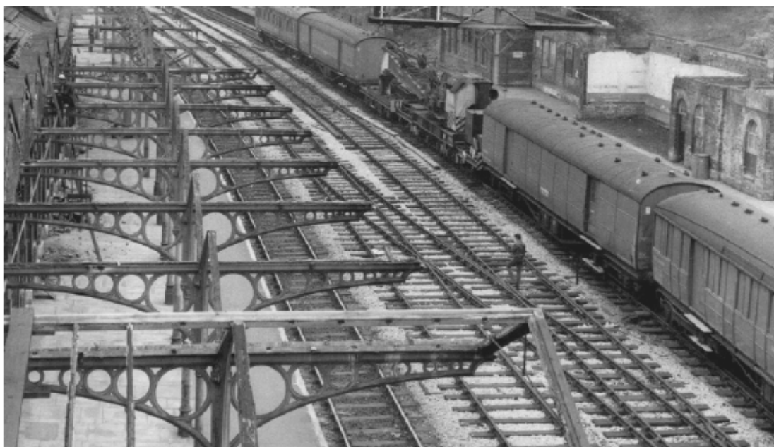
Plate 15: Disassembling the platform canopies on the 'Up' platform in the summer of 1970, by which date the buildings on the 'Down' platform had been partially demolished (Bury Archive Service)
