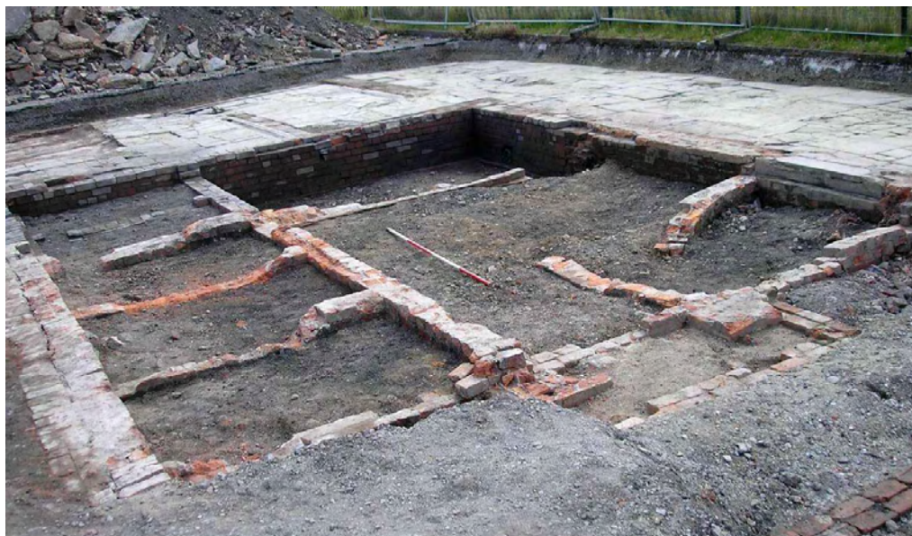
Plate 27: Foundations of the toilet block shown on the 1944 engineering plan
