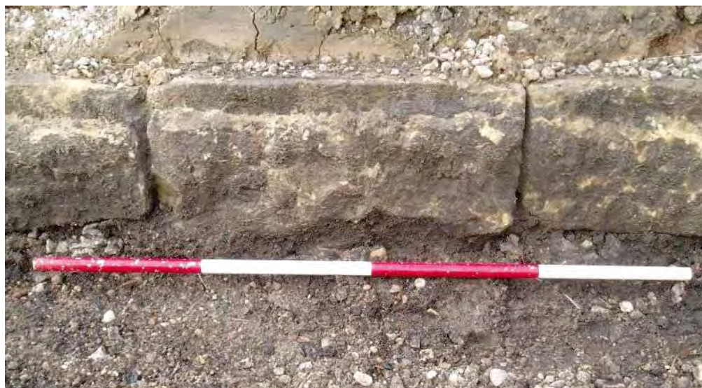
Plate 19: Stone blocks ( I90 ) forming the eastern kerb of the 'Up' platform
