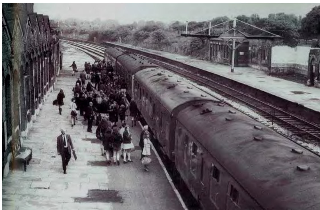
Plate 16: Looking south-east along the 'Up' platform in October 1970, during the station's final week in service. Note the absence of the platform canopies (Bury Archive Service)
