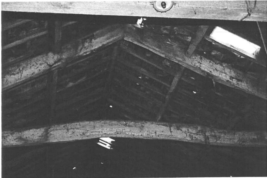
Plate 24: The waney-edged truss within the original phase of the East Barn
