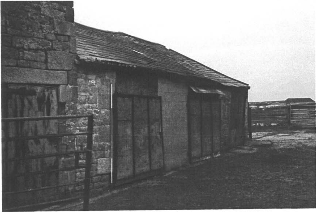
Plate 19: The single-storey extension at the south end of the East Barn
