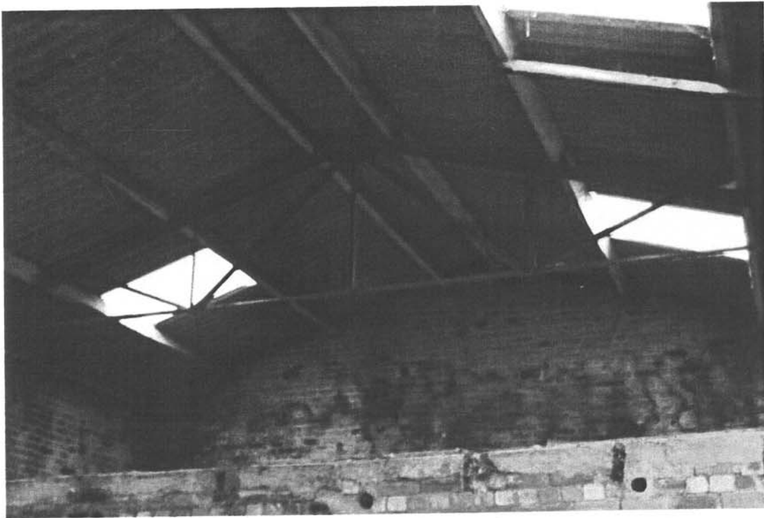
Plate 10: Detail of one of the modern trusses within the North Barn
