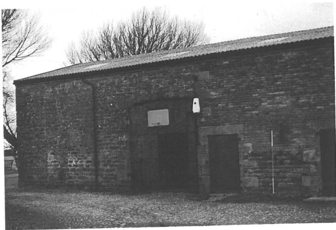
Plate 8: The stone extension to the west of the North Barn
