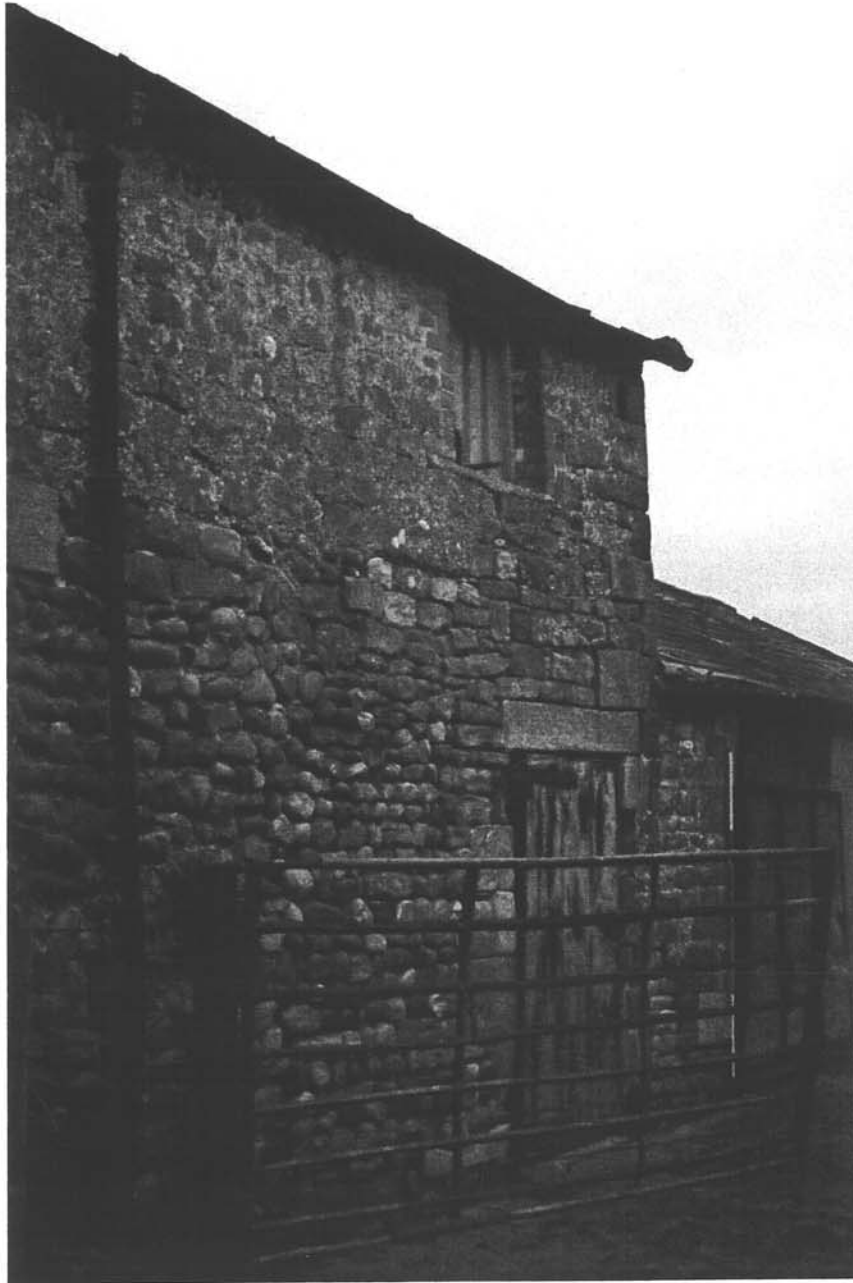
Plate 18: Detail of the west elevation of the East Barn featuring rebuild at the south end of the second phase, with the later single-storey phase in the background
