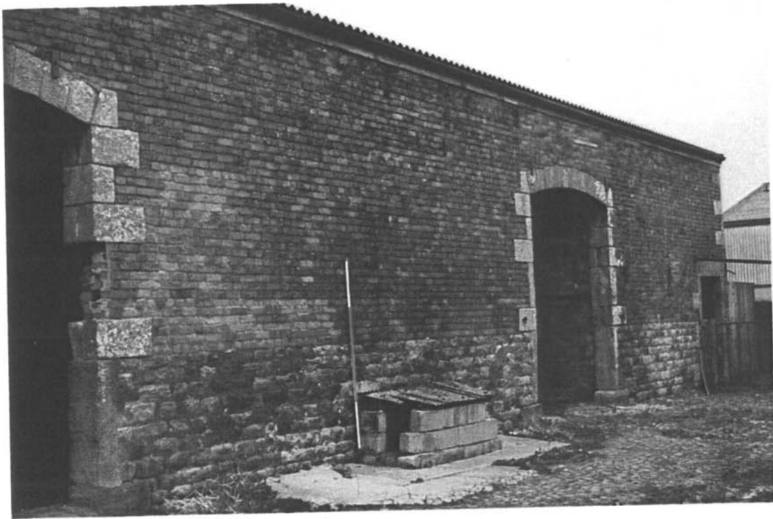
Plate 7: The original stone and brick build on the south elevation of the North Barn
