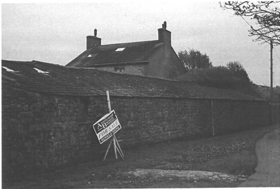
Plate 4: The west elevation of the West Cow Shed
