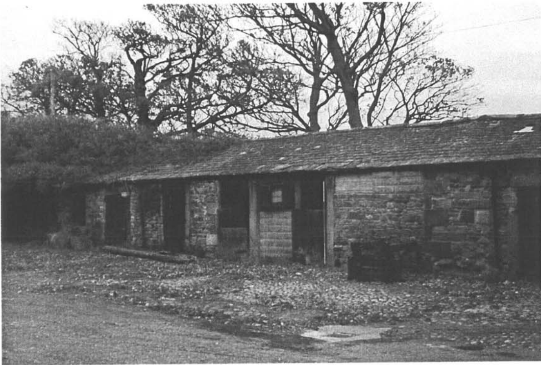
Plate 1: The east elevation of the West Cow Shed facing south-west
