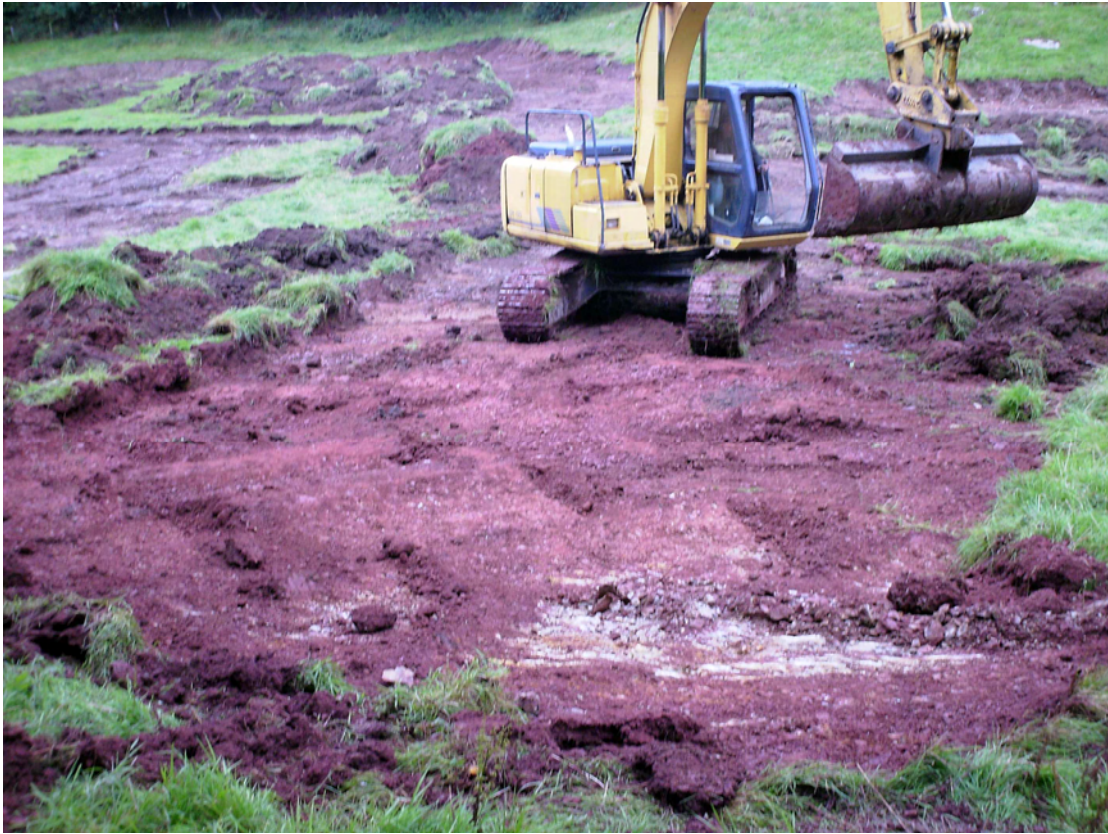
Plate 1: Topsoil stripping of caravan platform; working shot showing intermittent exposure of limestone bedrock
