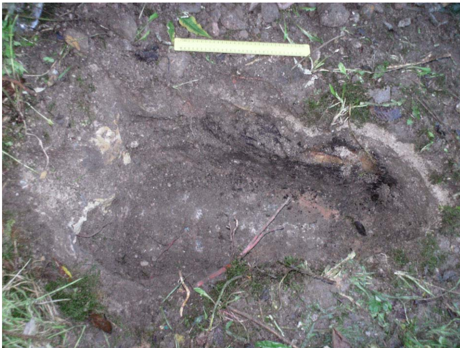
Plate 6: Test Pit 3 showing concrete surface 302 (0.3m scale)
