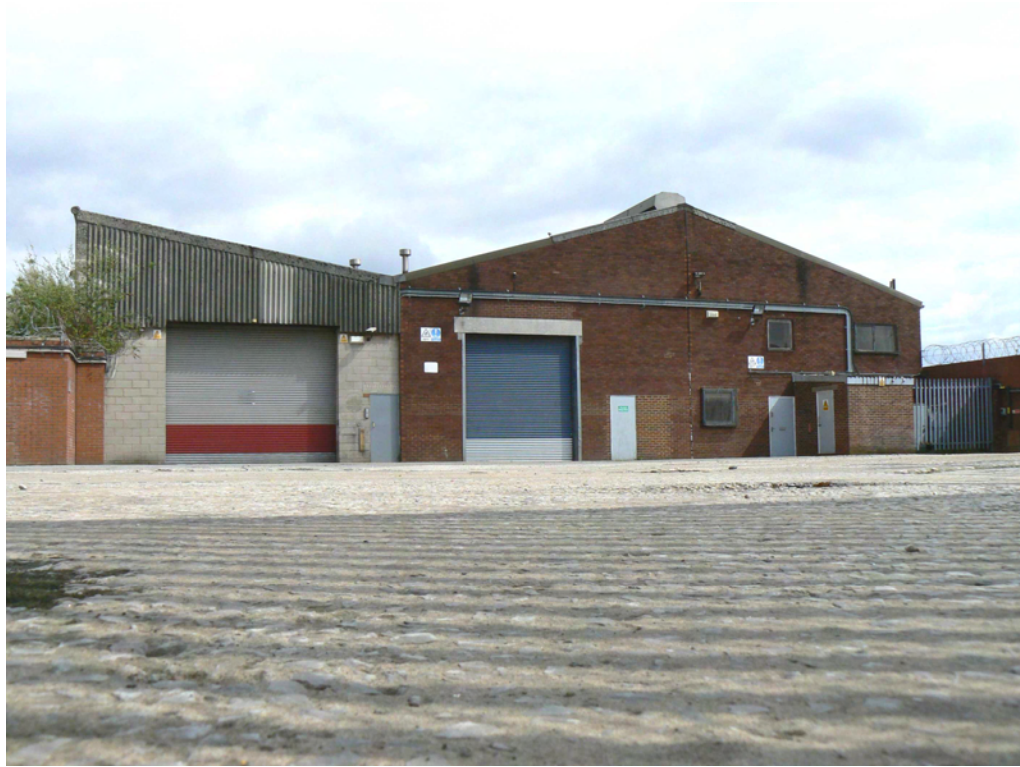
Plate 7: View across the storage yard from the Roger Street entrance
