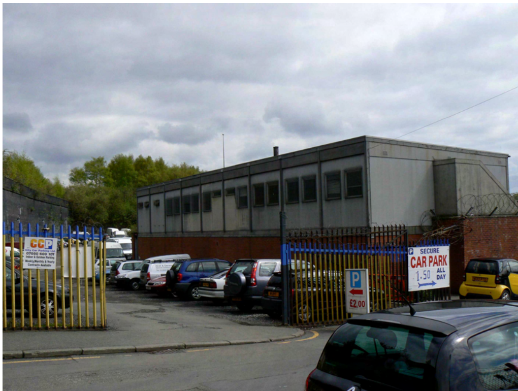
Plate 10: View along Brighton Street, showing temporary office accommodation in the south-western corner of the Scheme Area
