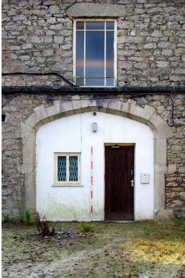
Plate 27: Main doorway, Building 3
