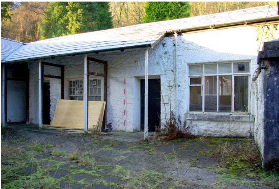
Plate 20: View of the east-facing elevation of Building 2
