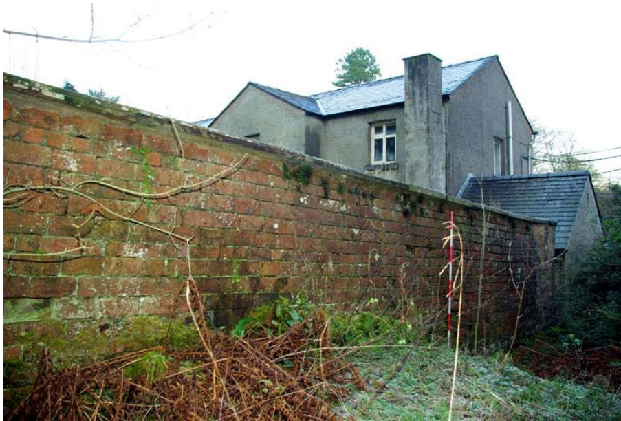
Plate 41: Eastern part of the south boundary wall of the walled garden
