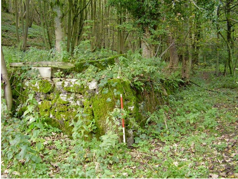
Plate 56: Revetment wall of the terrace looking north
