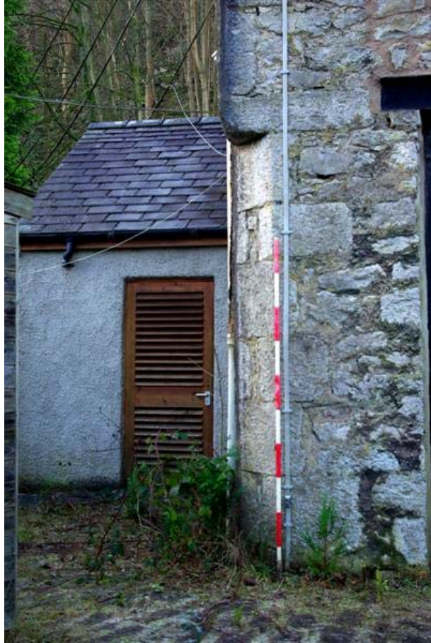
Plate 28: Chamfering at south-east corner of the Building 3
