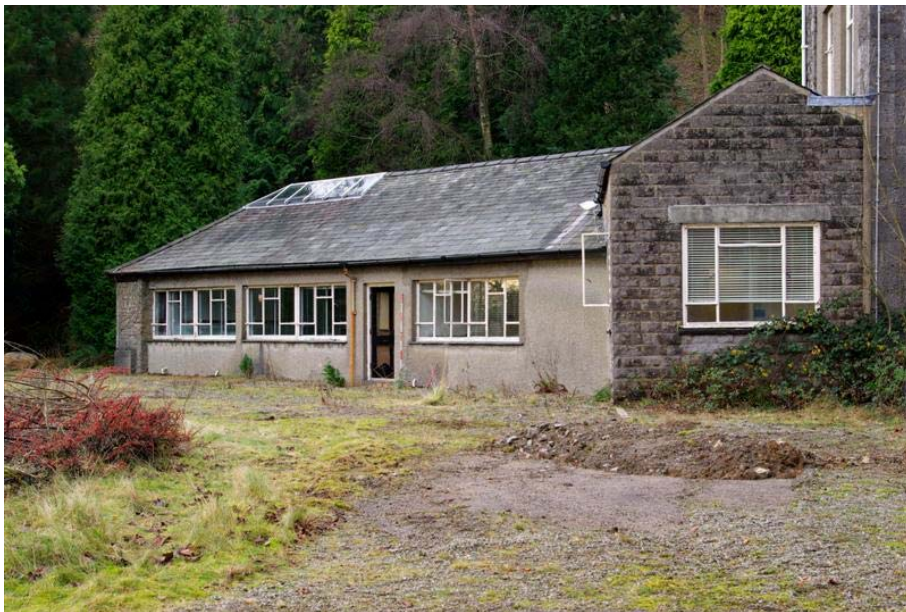
Plate 2: General view of Building 1, facing west
