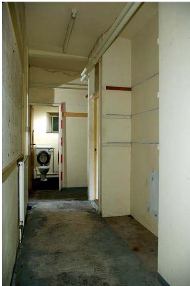
Plate 24: General view of Room B2-10 , facing west
