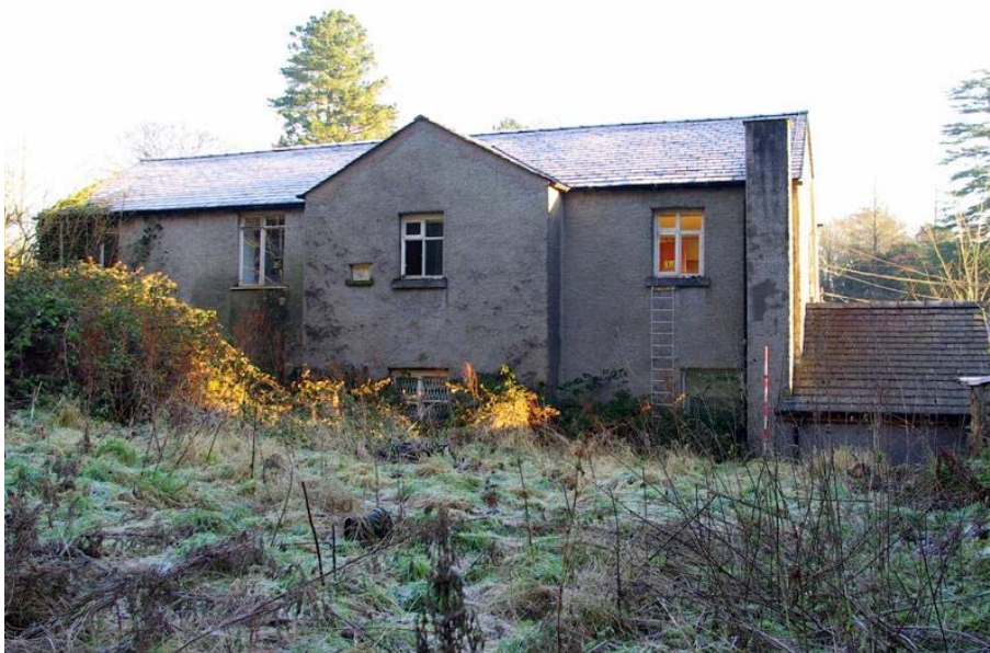
Plate 26: Rear view of Building 3, facing east
