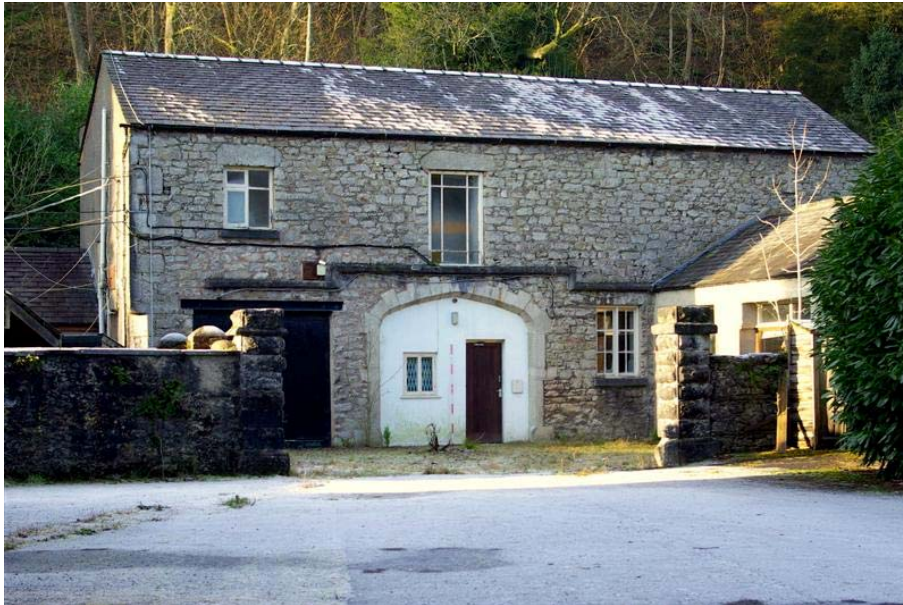
Plate 25: General view of Building 3, facing west
