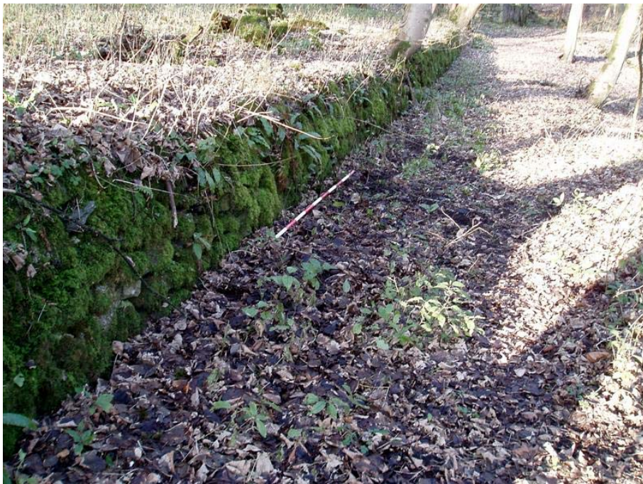
Plate 57: Revetment wall of the terrace looking north
