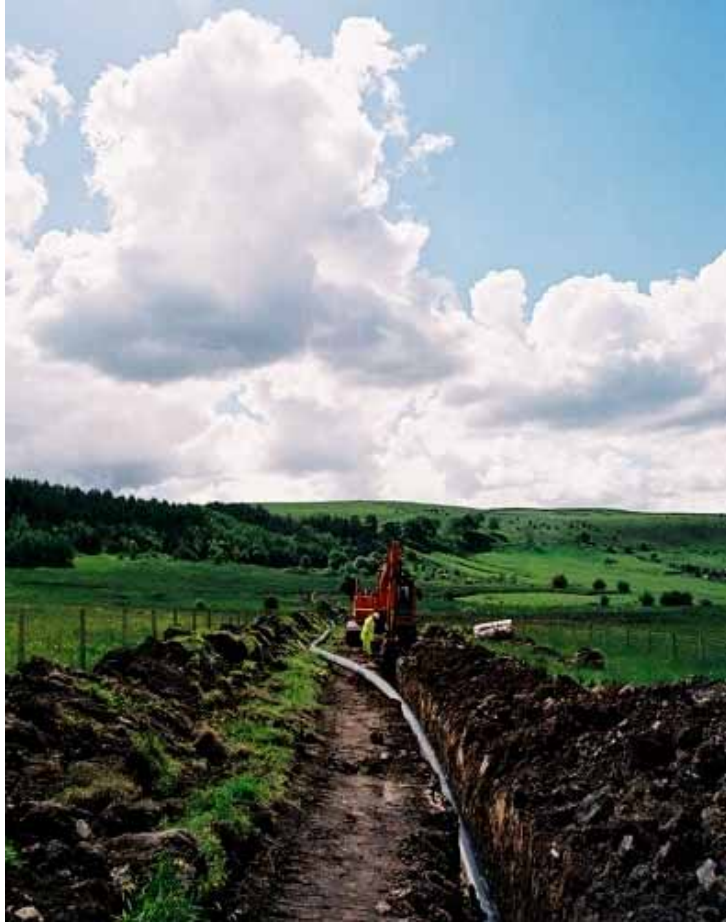
Plate 3: Topsoil stripping within the pipeline easement
