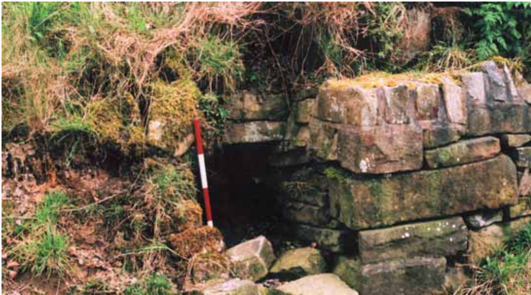
Plate 4: Culvert 161 on Ogden Lane, facing south
