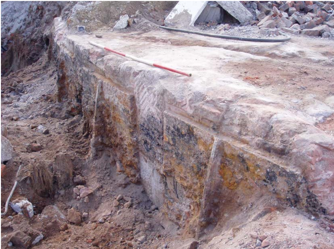
Plate 4: Iron supports for the pier footing (7001), looking south
