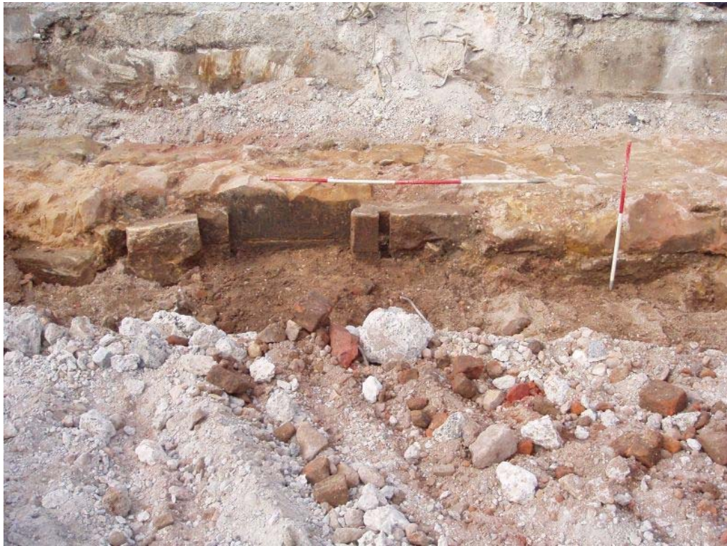
Plate 5: Elevation view of wall 7000 , the rear face of George's Ferry Basin south wall, looking north
