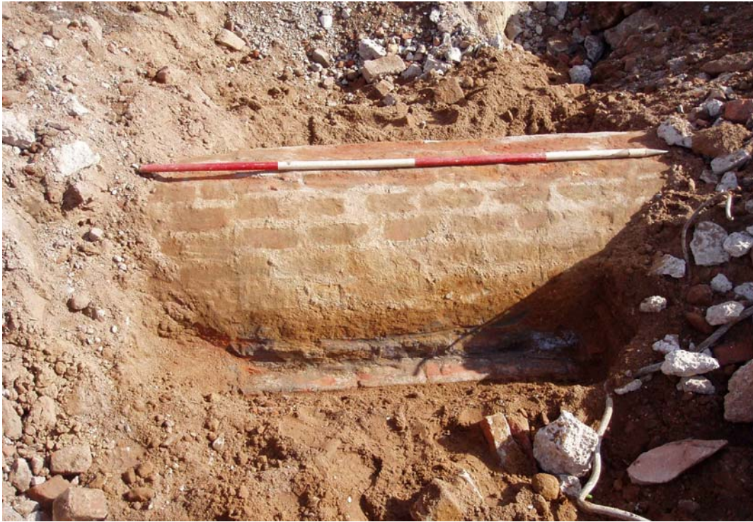
Plate 7: Brick culvert 7005 , looking east
