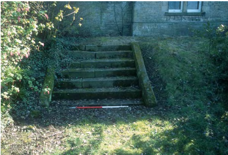
Plate 14: The stone steps between the terraces at the rear of the building
