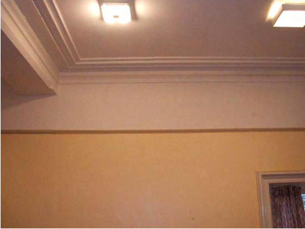
Plate 9: Detail of the chamfered beam and the cornice within Room 2.
