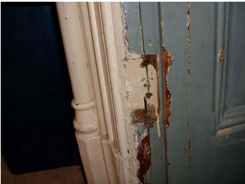
Plate 10: Detail of the architrave adorning the principal doors of the building.
