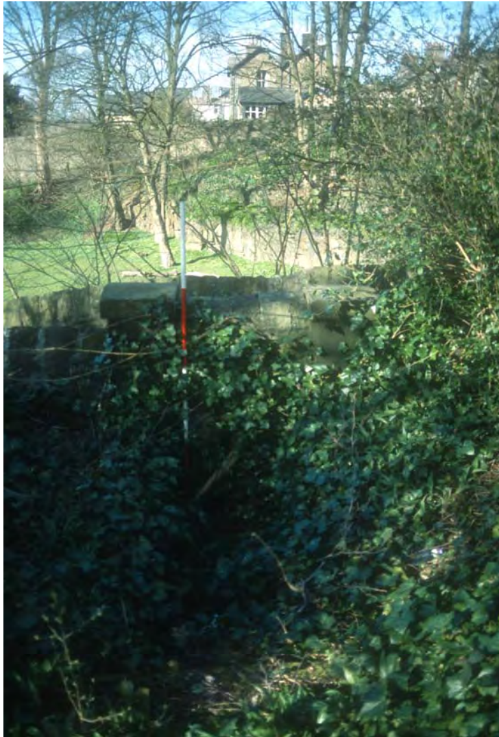
Plate 17: The blocked gate within the north extent of the perimeter wall.
