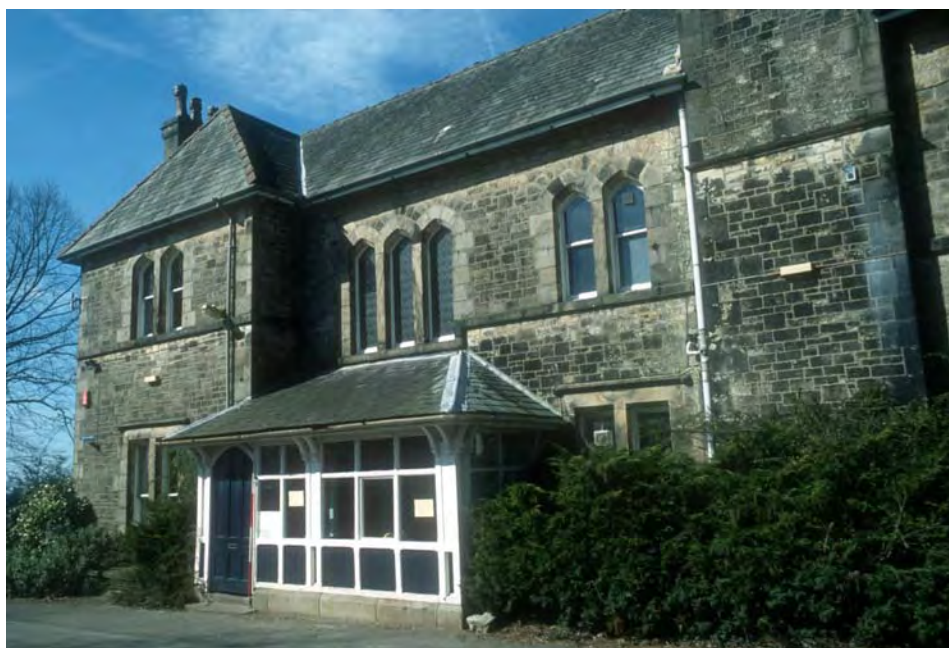
Plate 2: The front (south) elevation of the building from the south-east.
