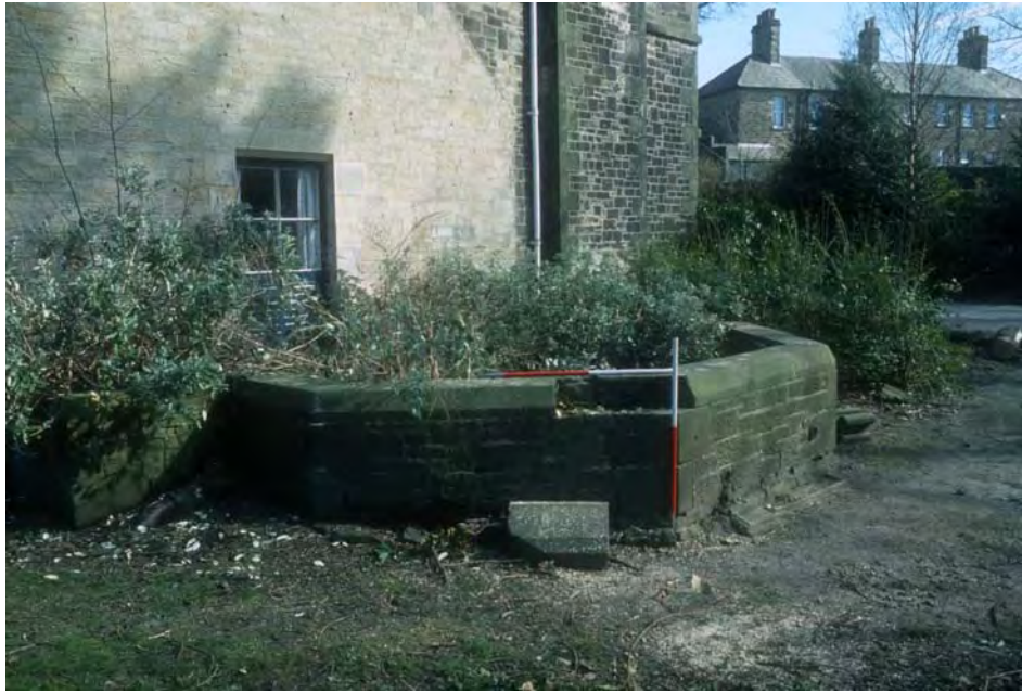
Plate 13: The remains of the Conservatory on the west end of the building
