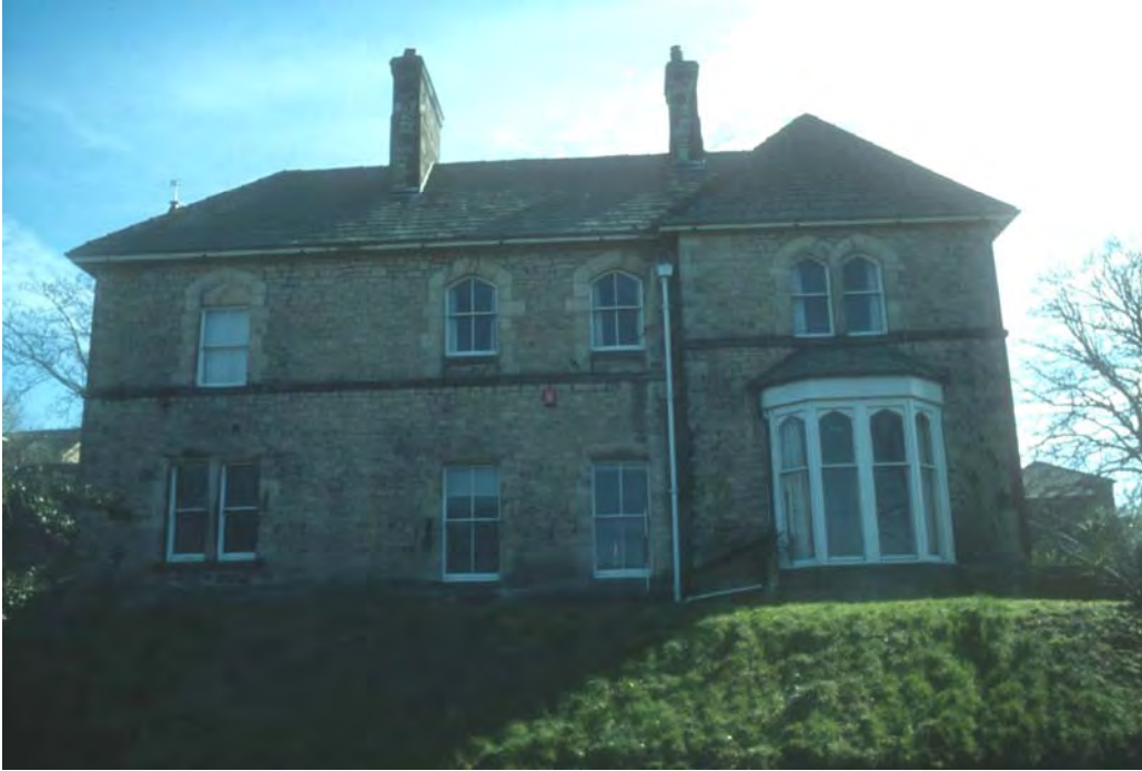
Plate 4: The north elevation.
