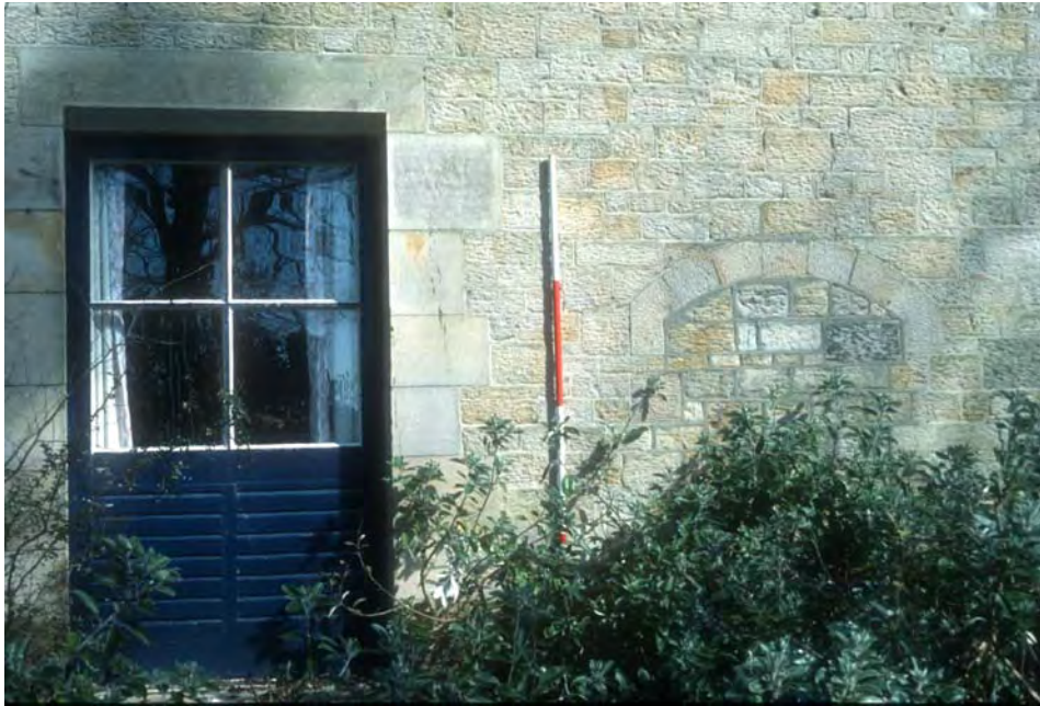
Plate 6: Detail of the converted window and blocked aperture on the west elevation.
