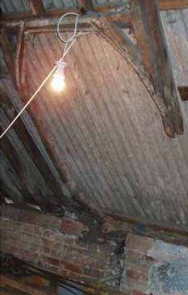
Plate 15: Detail of position of former dormer window, F2, Outbuilding 1 (supplied by clients architect)
