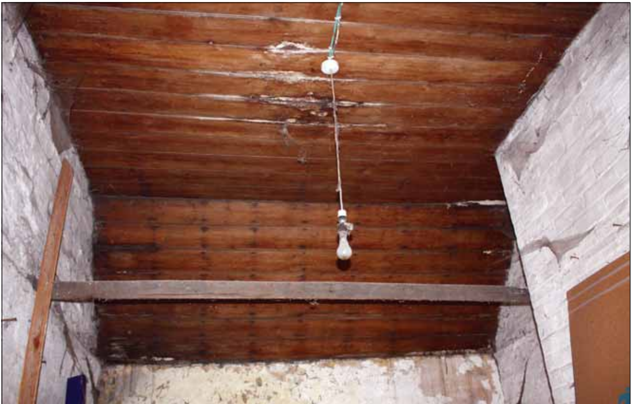
Plate 20: Detail of boarded ceiling, G5, Outbuilding 2
