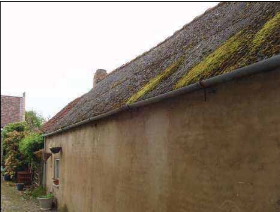
Plate 10: North-facing elevation of Outbuildings 1 and 2 (supplied by clients architect)
