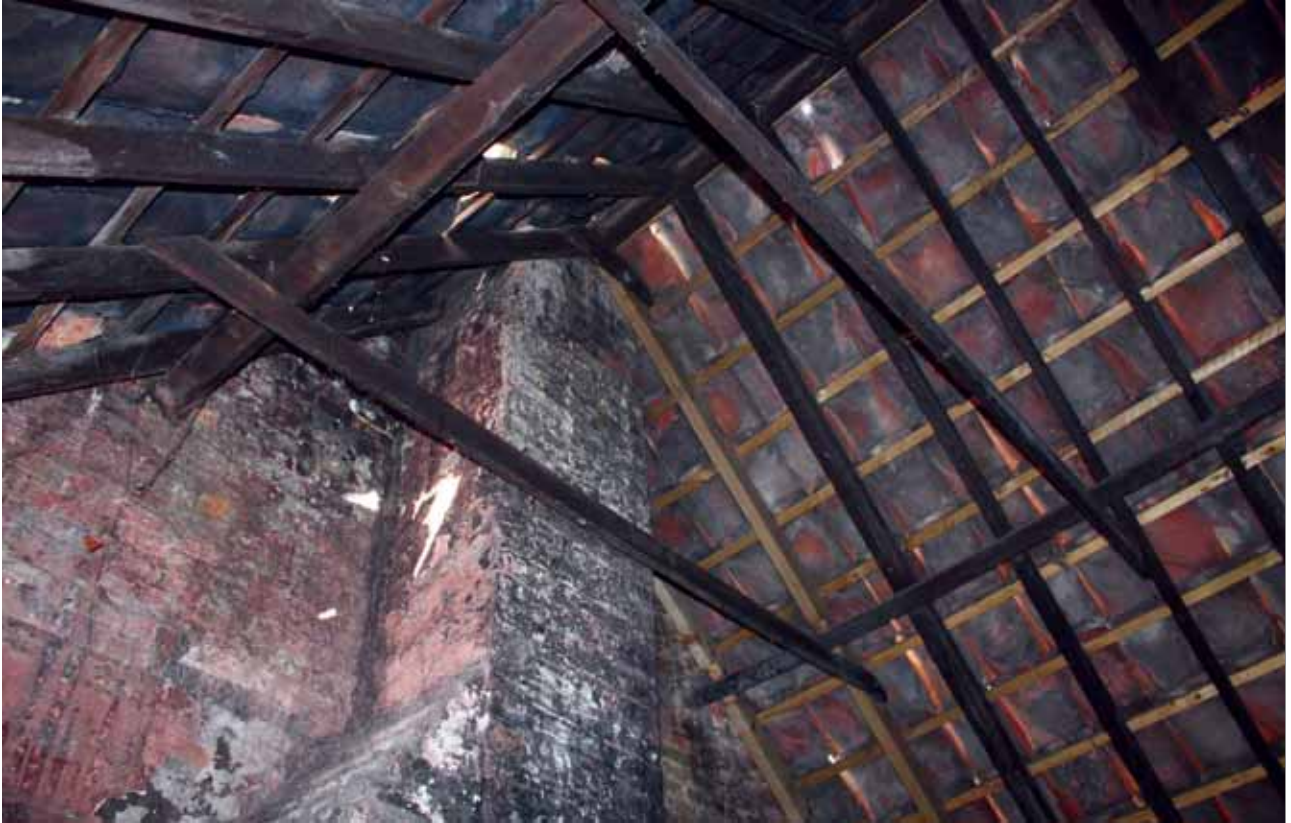
Plate 17: Detail of roof structure showing evidence of burning, G4, Outbuilding 2
