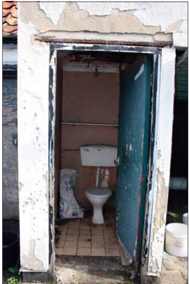
Plate 24: Outside toilet (G7), Outbuilding
