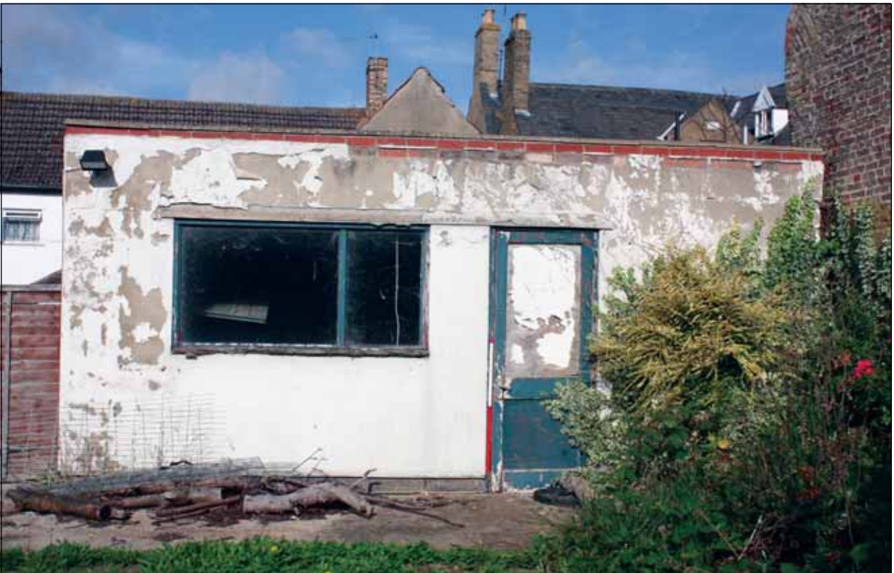
Plate 8: Outbuilding 2, east-facing elevation
