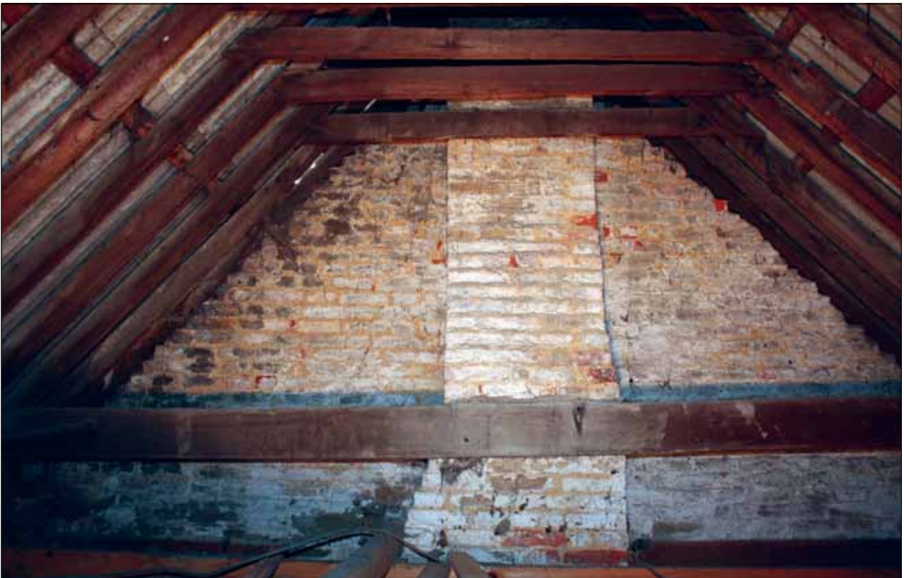
Plate 14: Detail of roof structure, chimney-breast and wall, F2, Outbuilding 1
