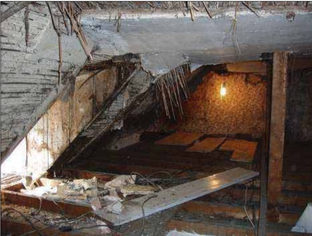
Plate 13: General view, F1, Outbuilding 1 (supplied by clients architect)
