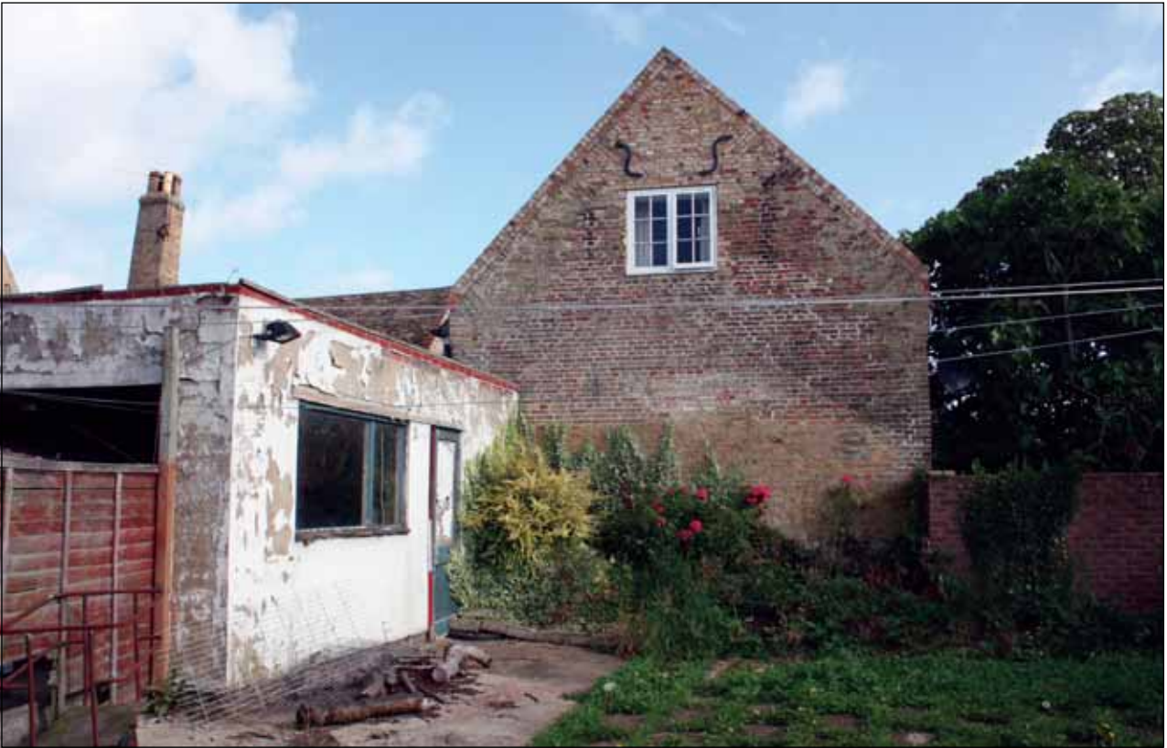
Plate 9: Detail of “ghostline” of former outbuilding on south-facing elevation of outbuilding at 110 High Street
