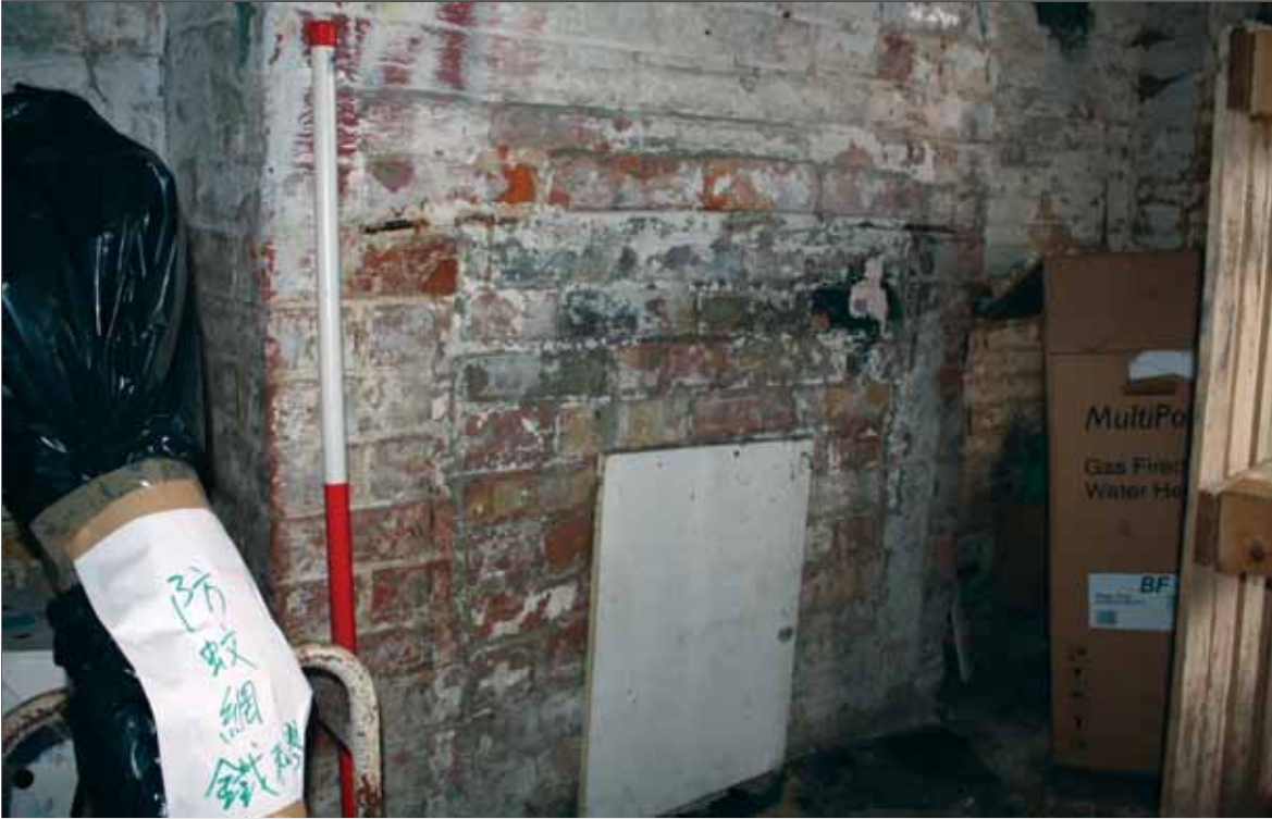
Plate 21: Detail of blocked-up fireplace, G5, Outbuilding 2
