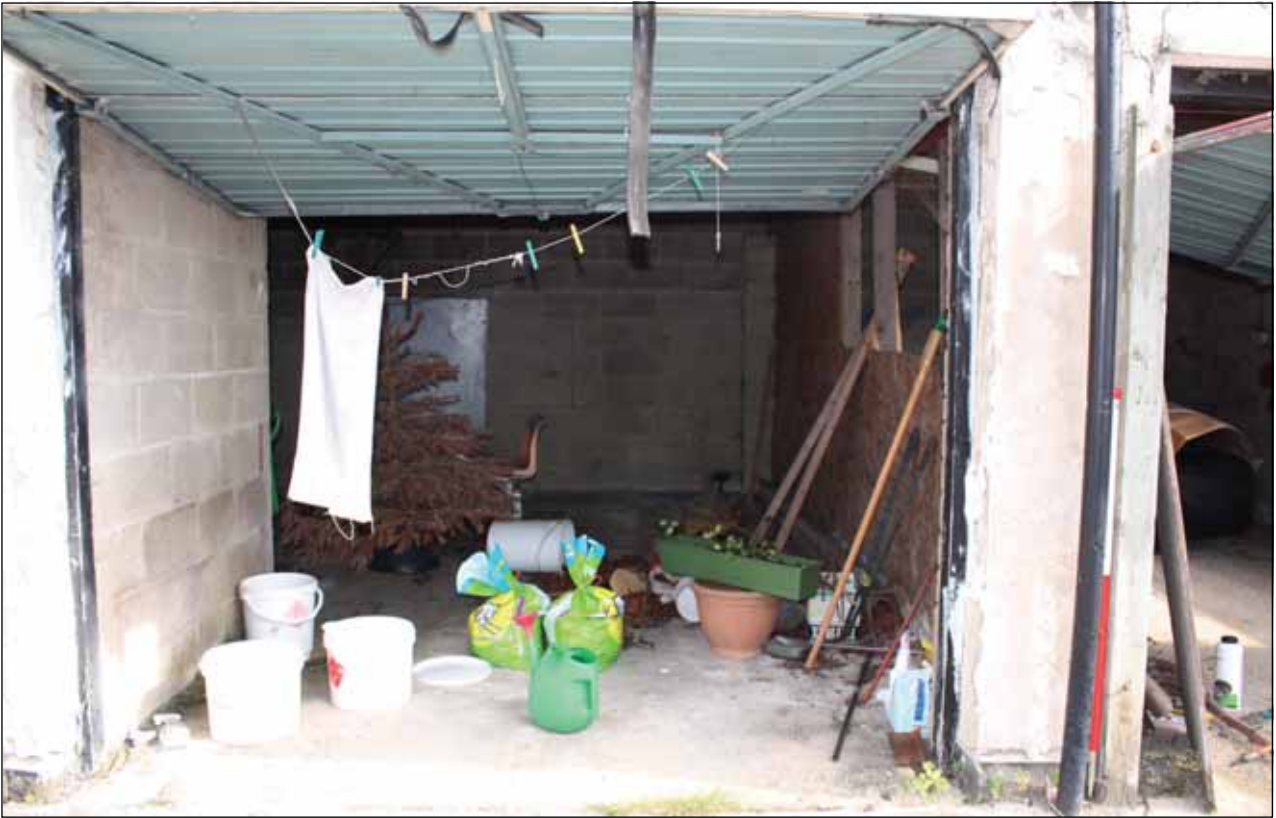
Plate 25: General room view, G8, Outbuilding 3
