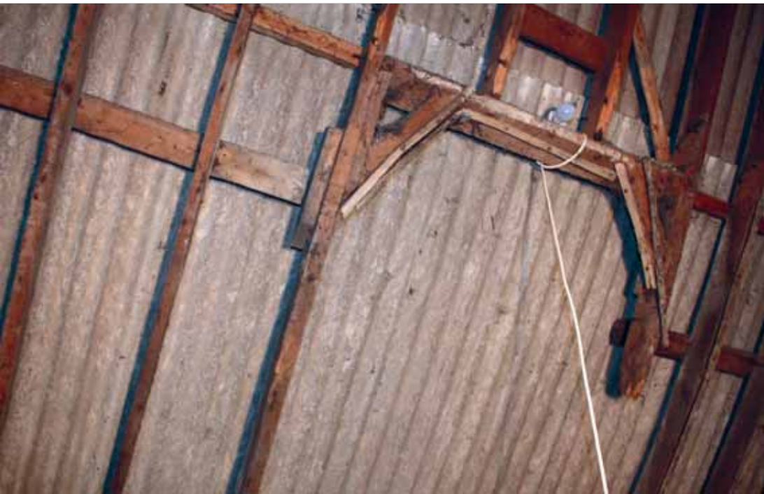
Plate 16: Detail of position of former dormer window, F2, Outbuilding 1
