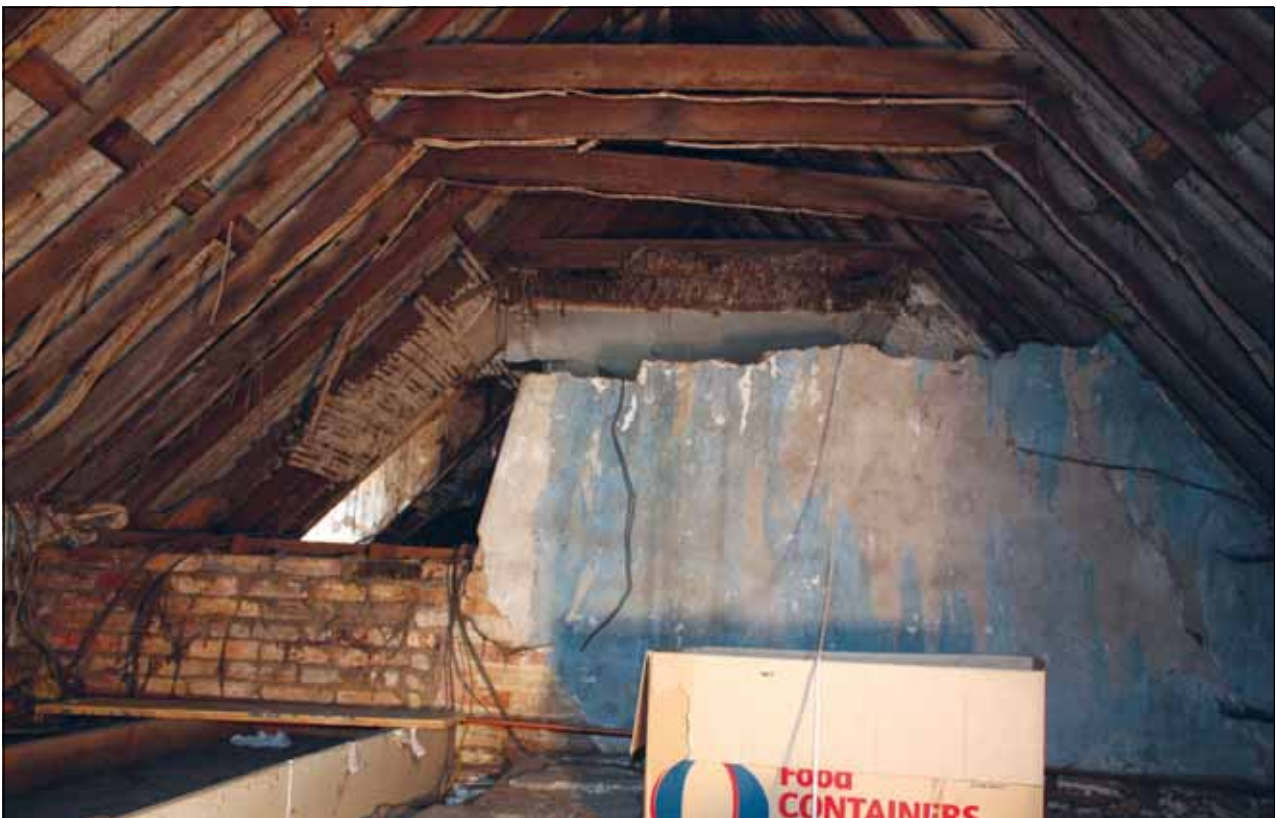
Plate 12: Detail of internal partition within roof space
