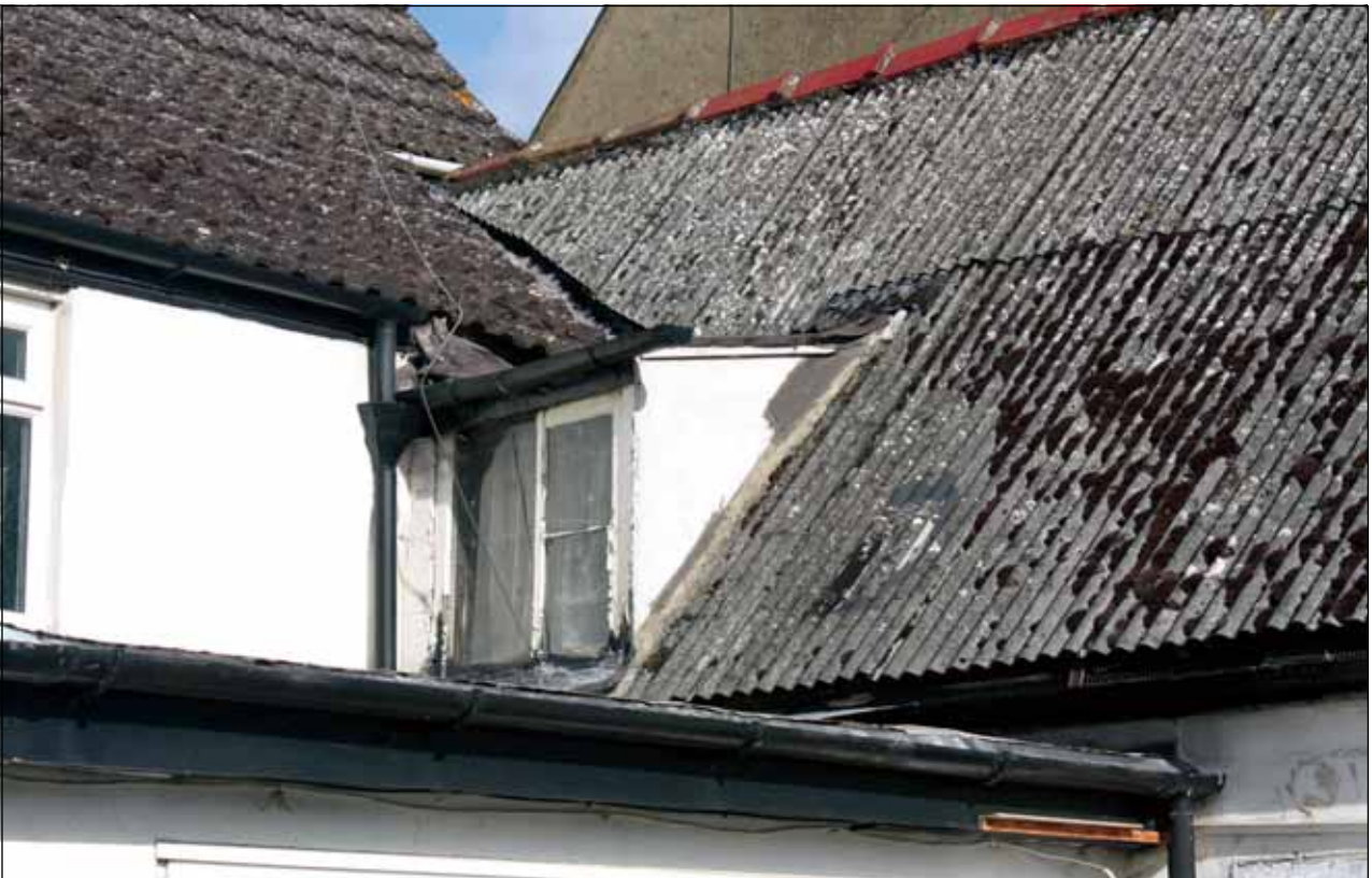
Plate 4: Dormer window of Outbuilding 1
