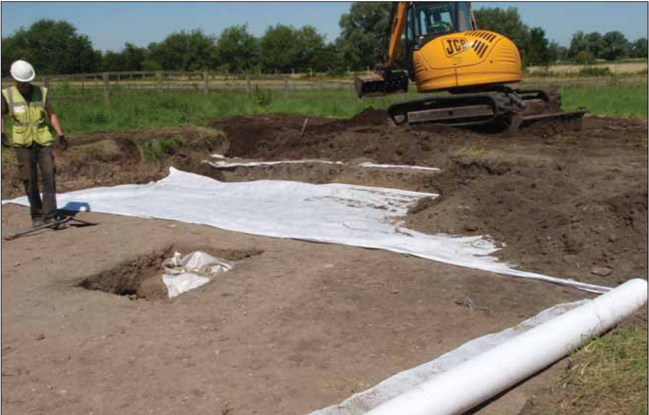
Plate 11: Laying of terram after infilling of test pits and burrows and prior to backfilling by machine (from south-east)
