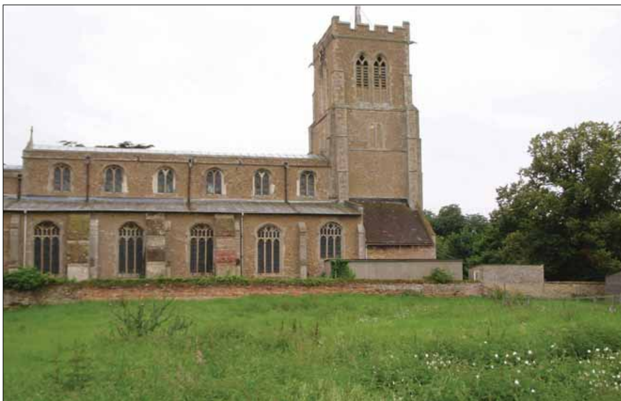
Plate 1: View of the site before excavation (from north)
