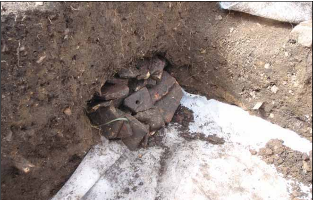
Plate 10: Detail of packing of one of the burrows/tunnels in Test Pit 1 and laying of terram prior to infilling by hand.
