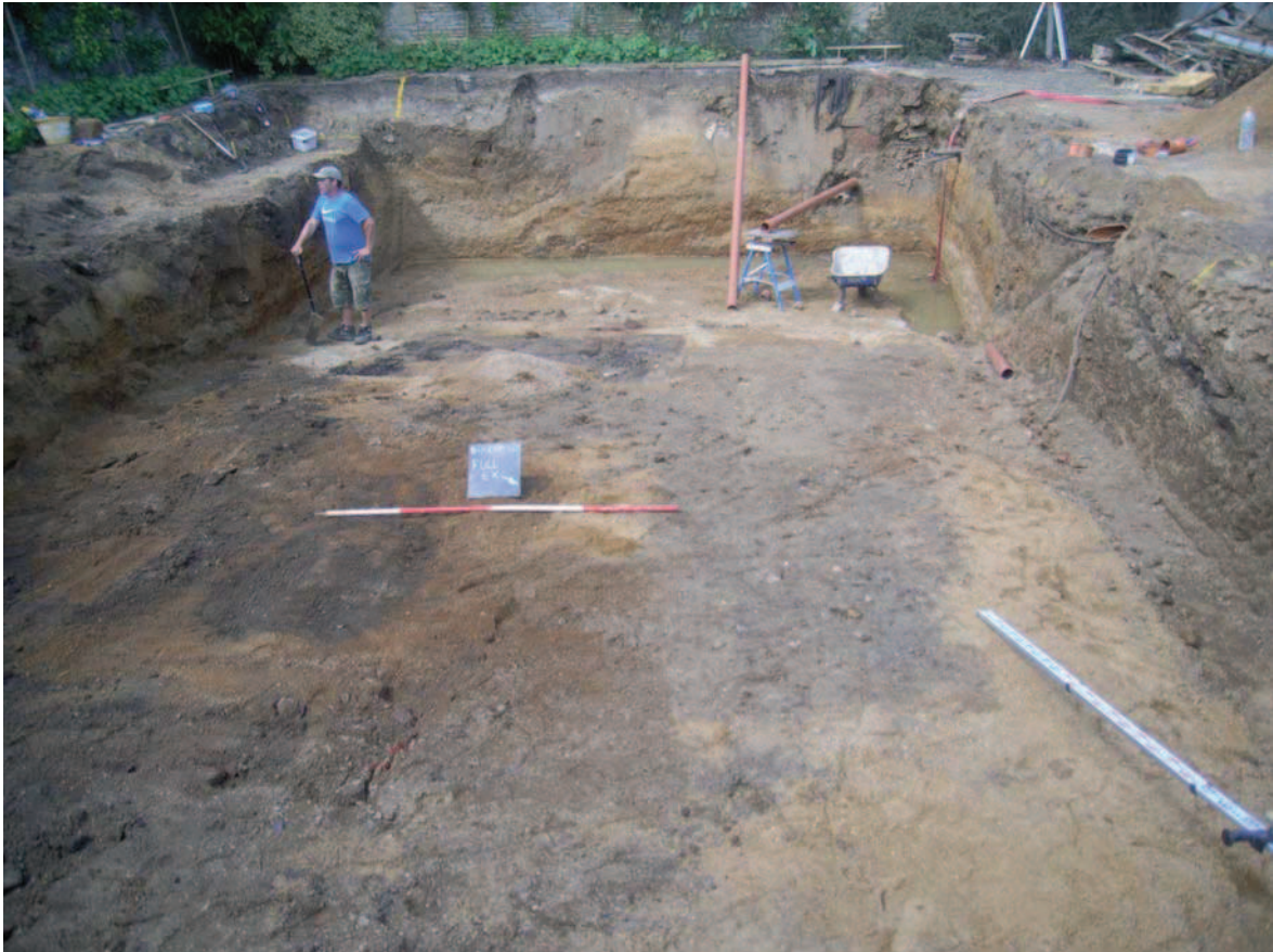
Plate 2: Swimming pool fully excavated, looking west
