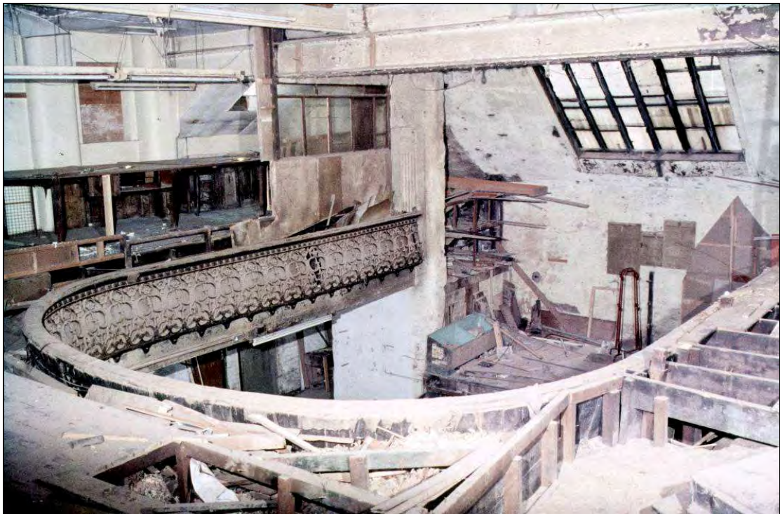
Plate 50: Horseshoe gallery with cast iron scrollwork balustrade (courtesy of the Visual Resources Centre at MMU)
