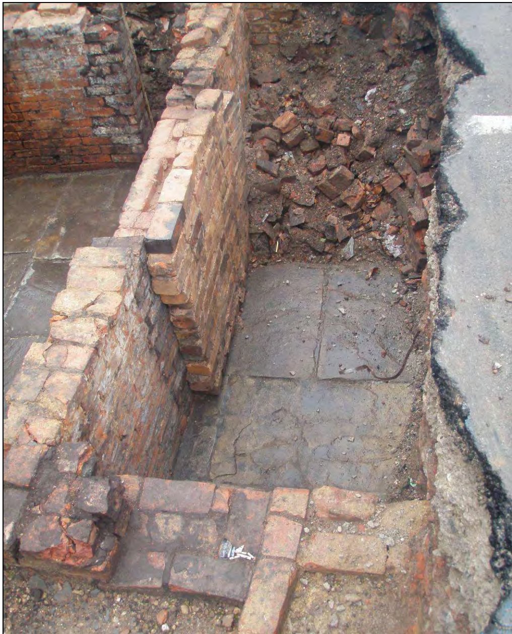
Plate 12: Cellar floor 1023 , showing firebrick 'skin' against rebuild 1005
