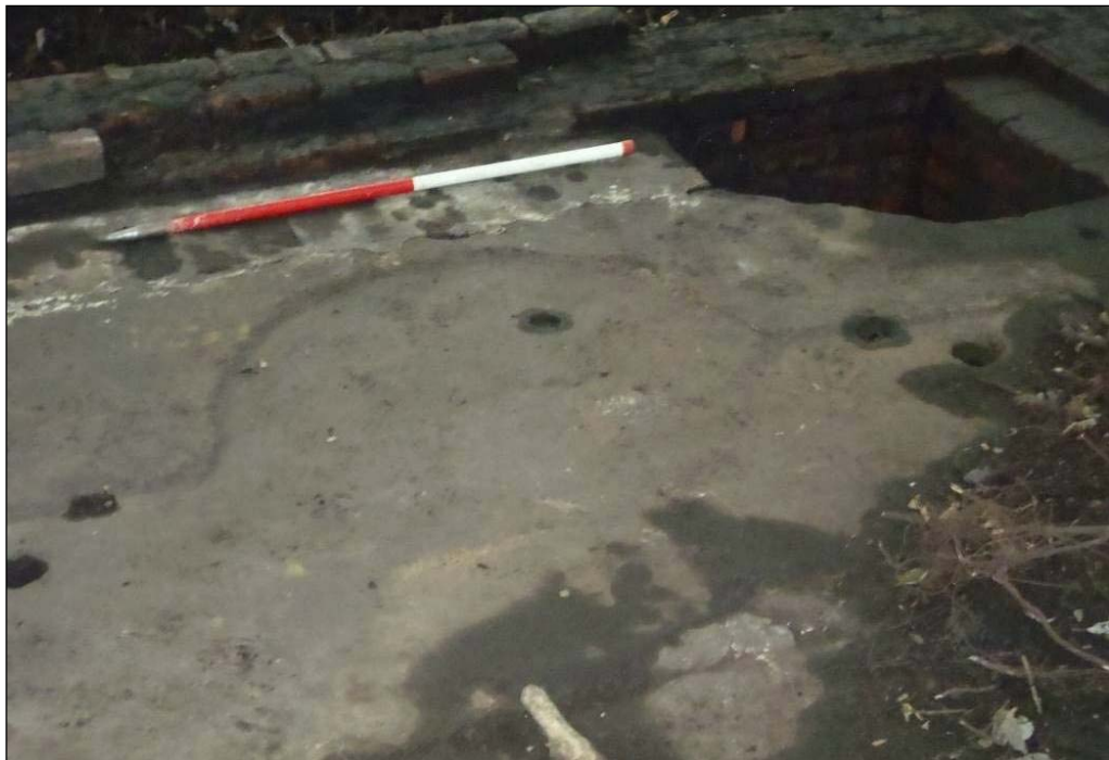
Plate 41: Shallow rebate cut into the surface of the stone engine bed
