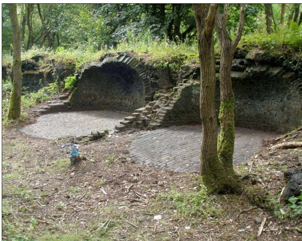
Plate 26: General view of part of the coke oven battery, looking west
