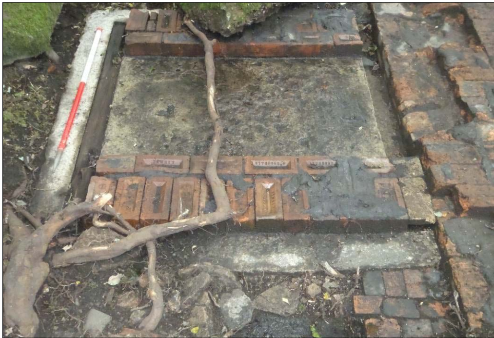
Plate 36: Small chamber within the fan house, probably representing the housing for an electric motor
