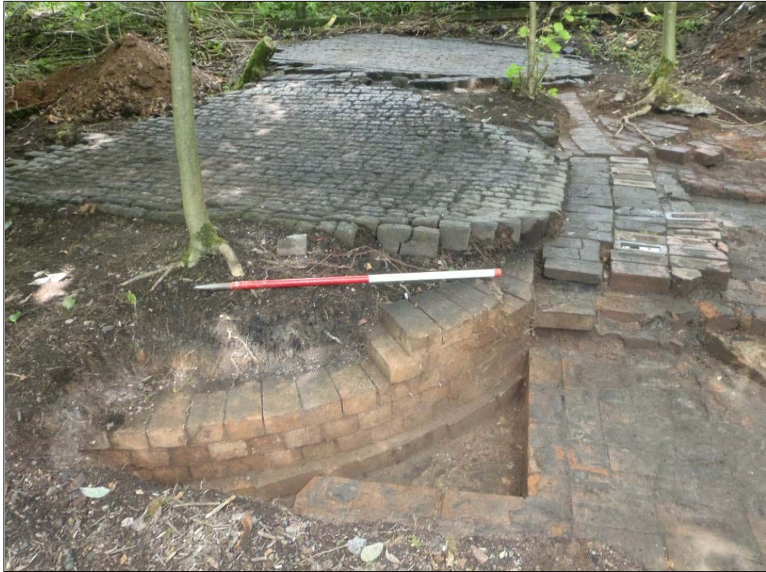
Plate 29: The remains of one of the coke ovens added to the main double bank between 1893 and 1909
