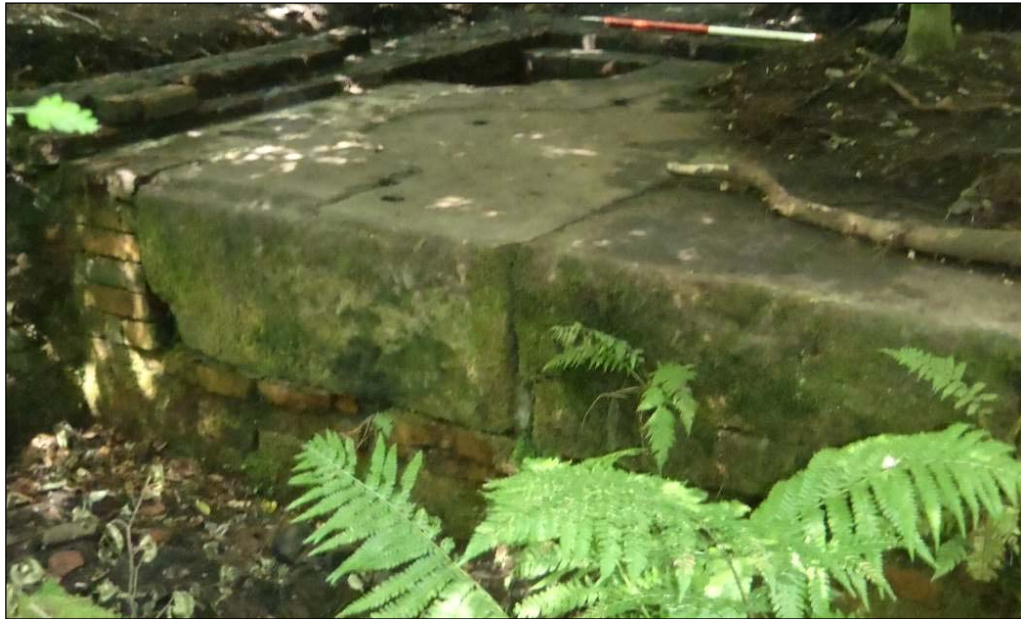
Plate 40: Large stone blocks forming the base for a small steam engine
