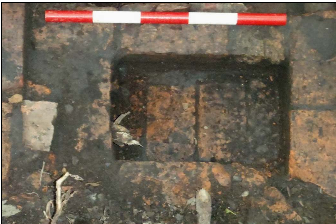
Plate 35: Setting for a vertical post on the wall of the fan house
