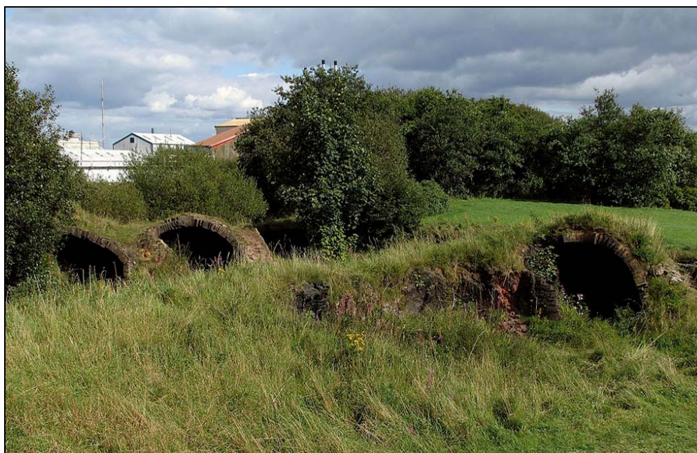
Plate 58: The remains of the beehive coke ovens at Aspden Colliery near Oswaldtwistle are comparable in size, form and date to those at Jubilee, but are afforded legal protection as a Scheduled Monument
