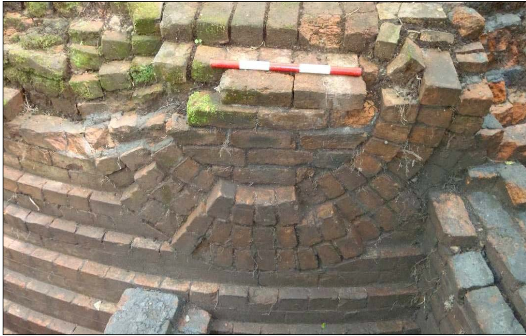
Plate 24: Relieving arch associated with a flue on the south-western side of the chimney
