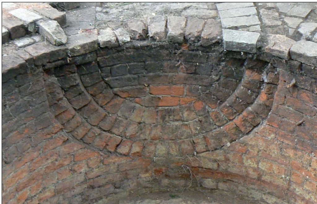
Plate 25: Relieving arch in the northern side of the chimney
