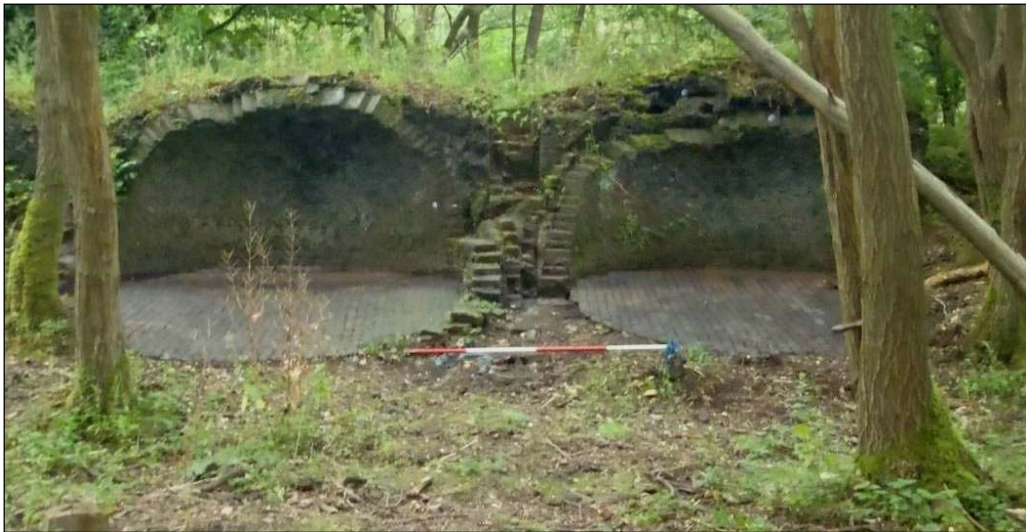
Plate 27: View of two of the surviving coke ovens in the main double bank
