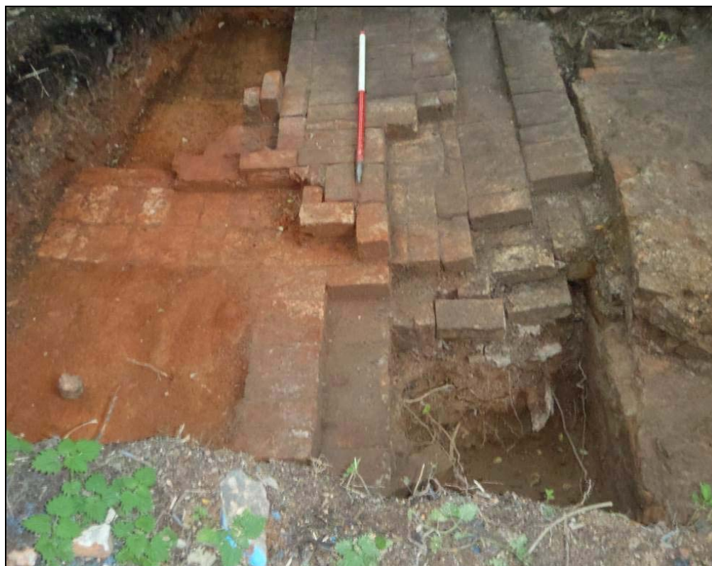
Plate 15: The floor of the boiler house to the east of the central flue, showing part of the earlier stone-built wall
