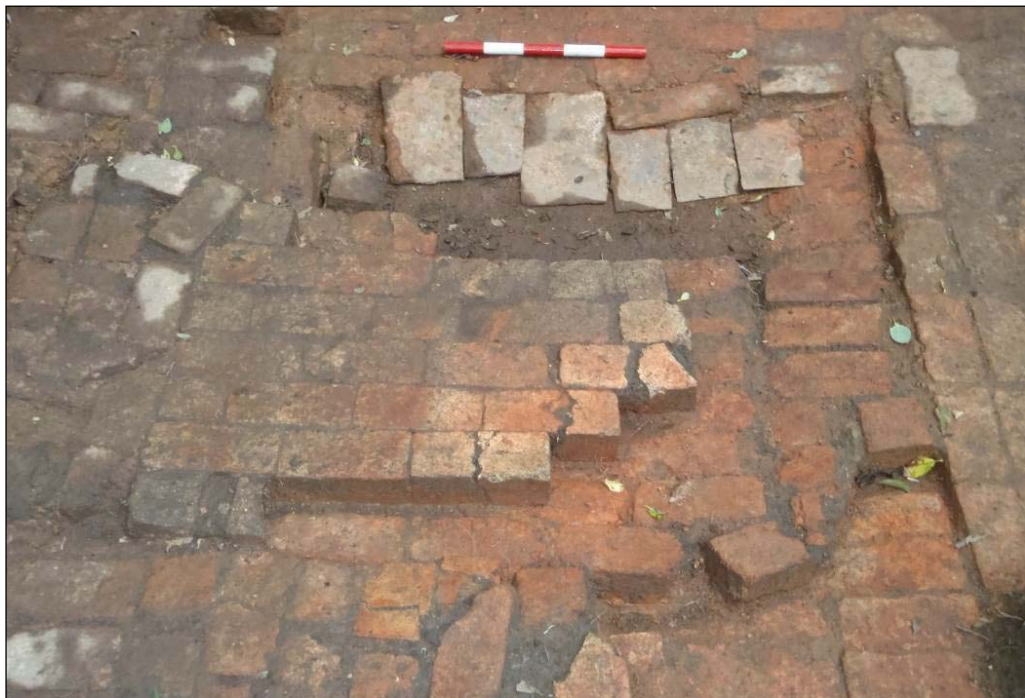
Plate 14: An area of sagging brickwork, with sloping slates to the south
