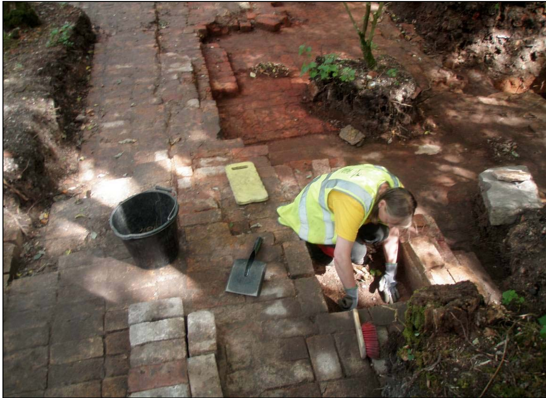
Plate 55: Excavating the rear part of one of the boiler bays
