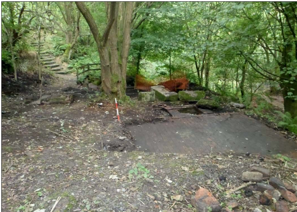
Plate 33: General view of the trench to the south of the upcast shaft
