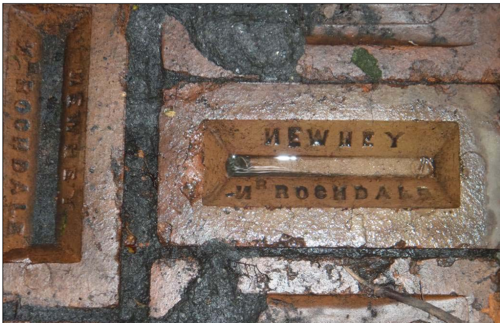
Plate 37: New Hey bricks in the fabric of the chamber wall
