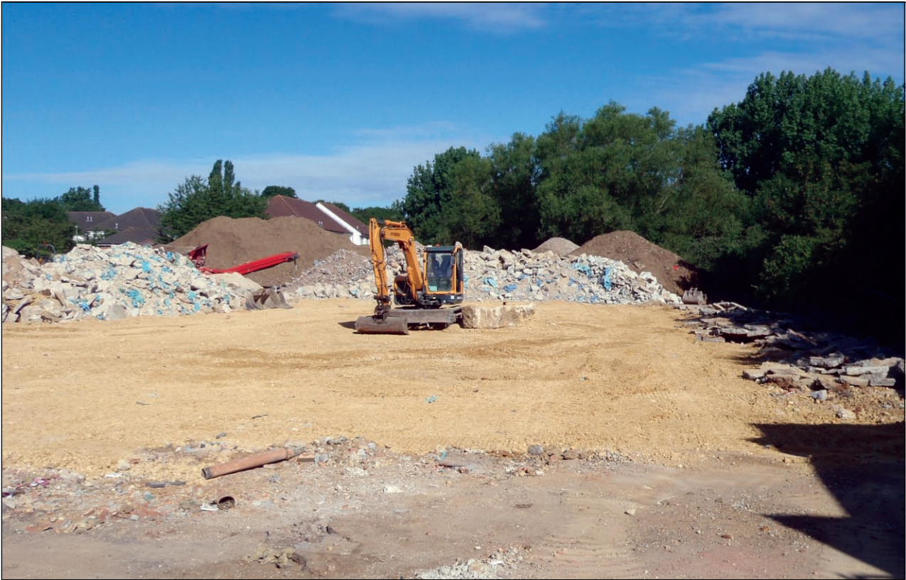
Plate 1: Demolition on site looking west
