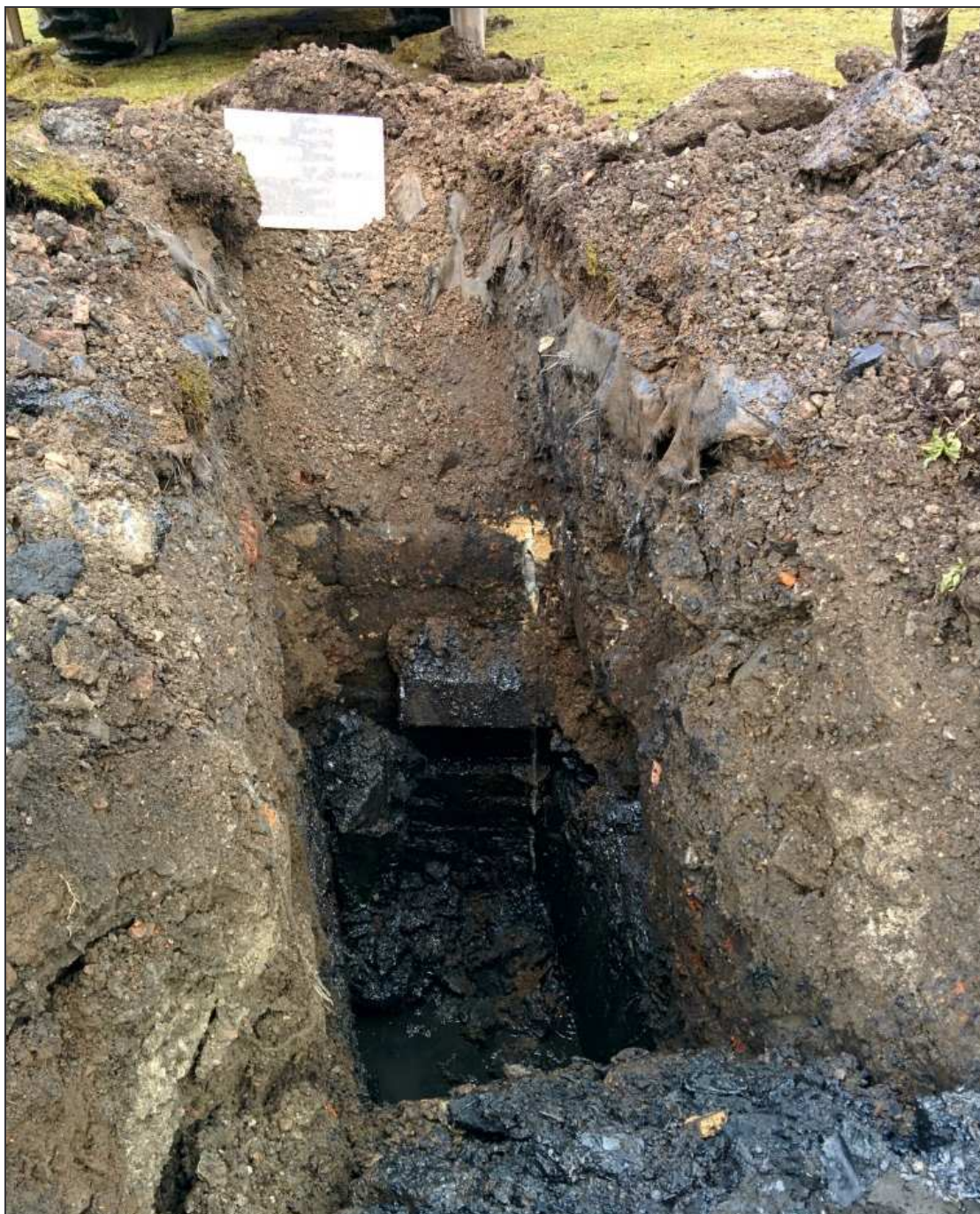
Plate 7: Structural remains exposed in TP2, presumably representing the original canal wall
