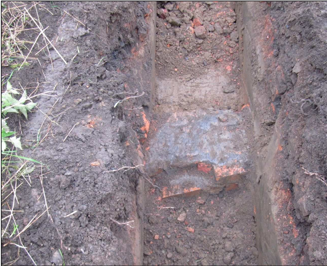
Plate 2: The brick wall in TP-116
