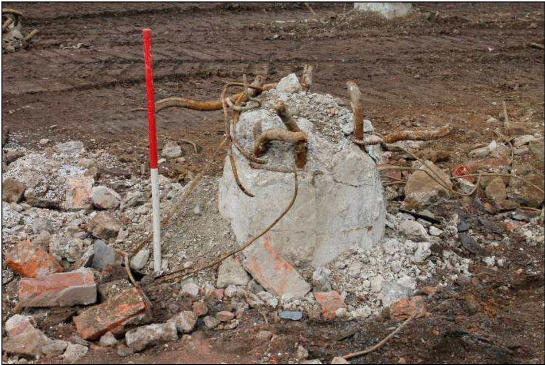
Plate 40: Octagonal reinforced concrete pile
