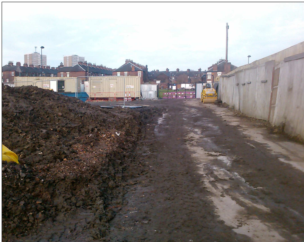
Plate 4: The site of the workers' housing prior to the commencement of any earth-moving works required by the construction programme
