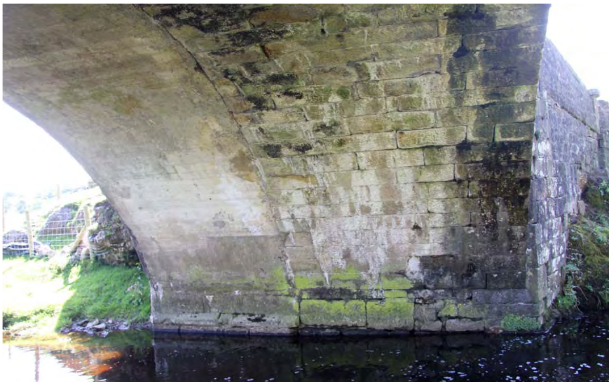
Plate 20: Underside of the primary arch showing the 1930 concrete arch and western masonry arch
