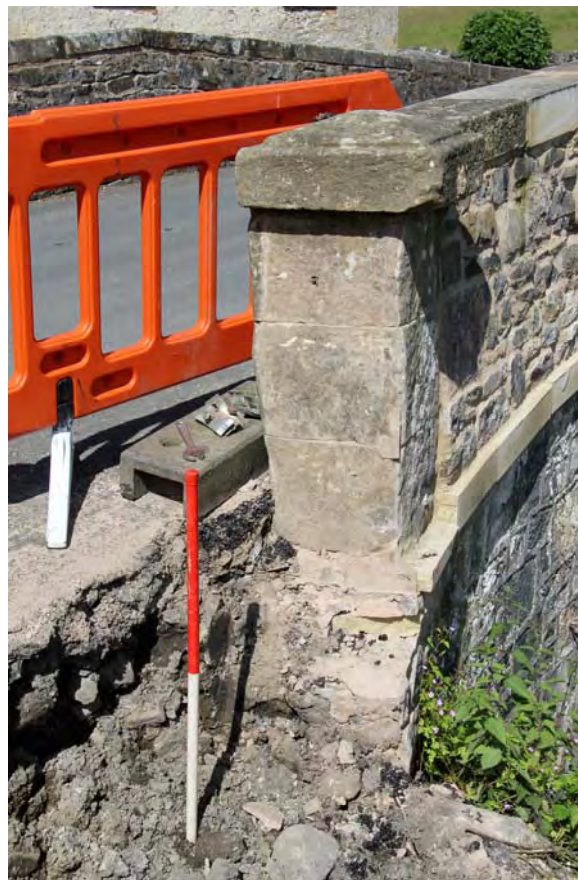
Plate 24: Southern terminal pillar of the eastern parapet, showing its placement on a modern section of string coursing following recent vehicle damage
