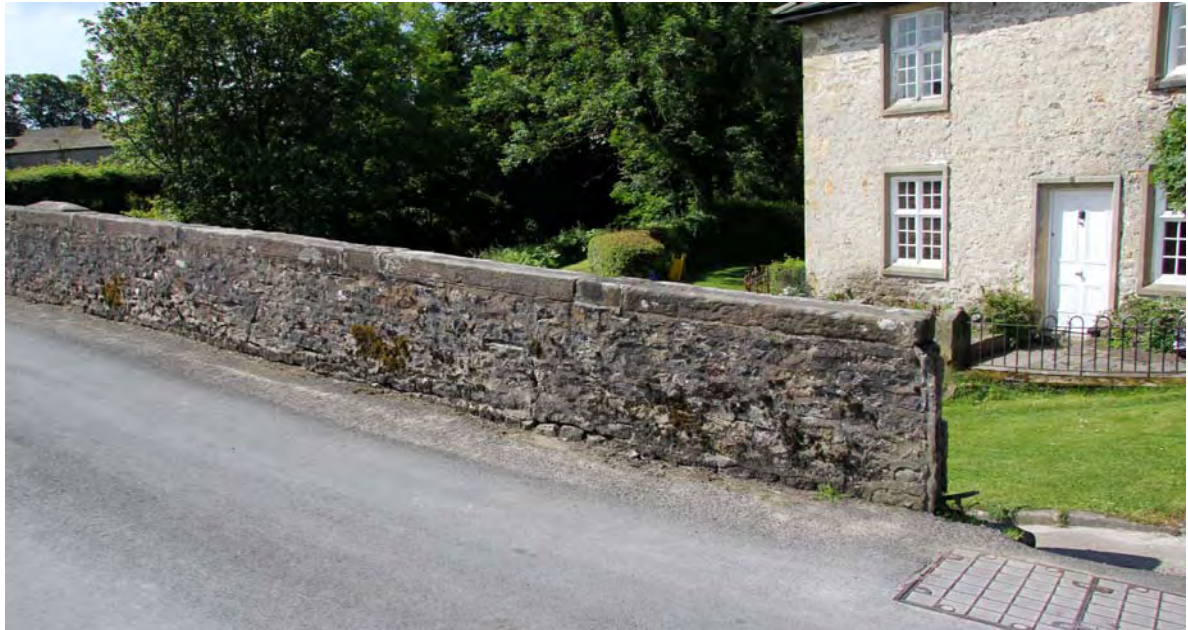
Plate 19: Northern section of western parapet showing the loss of the northern terminal parapet pillar
