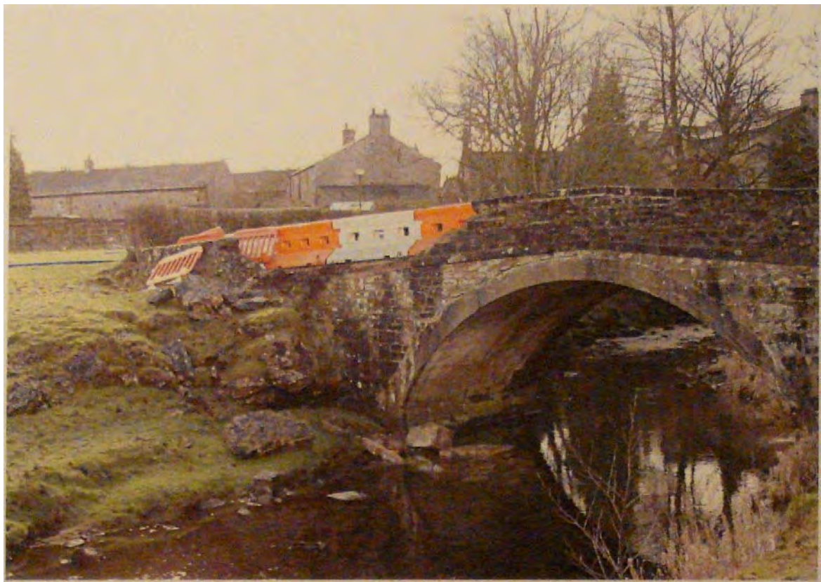
Plate 16: Damage to the bridge on 14/12/10 by a car in icy conditions (photo Slaidburn Archive)
