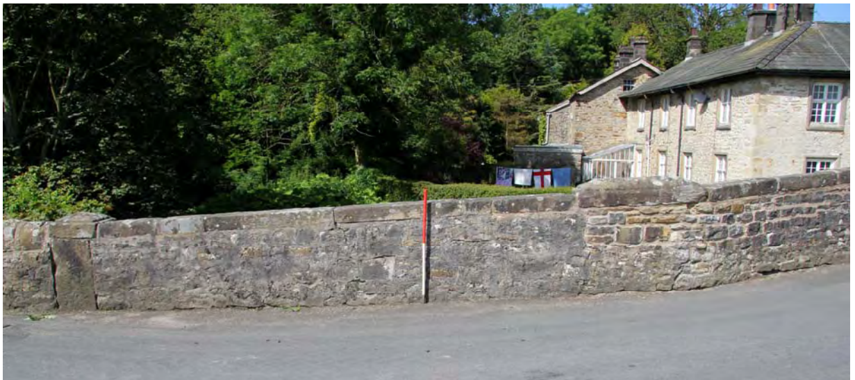
Plate 18: Western parapet showing patchy repairs as a result of vehicle damage
