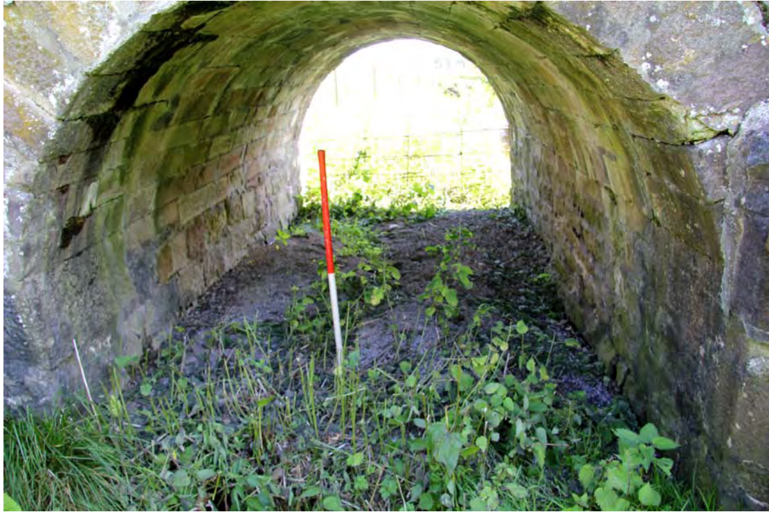
Plate 21: Underside of secondary arch, showing its patchy construction
