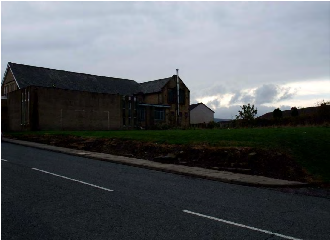
Plate 9: Site of former Mount Pisgah Chapel (Site 07)
