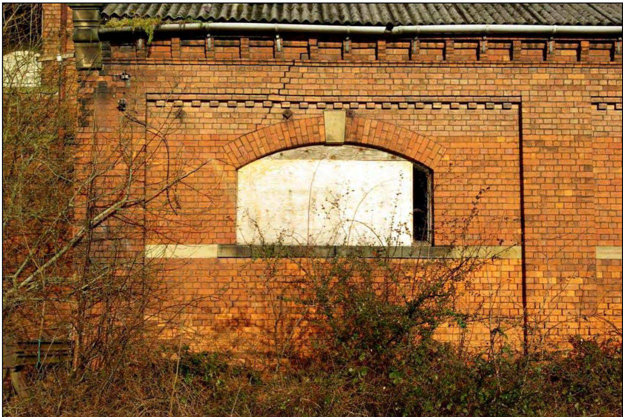
Plate 2: Example of a bay on the south elevation of the shed
