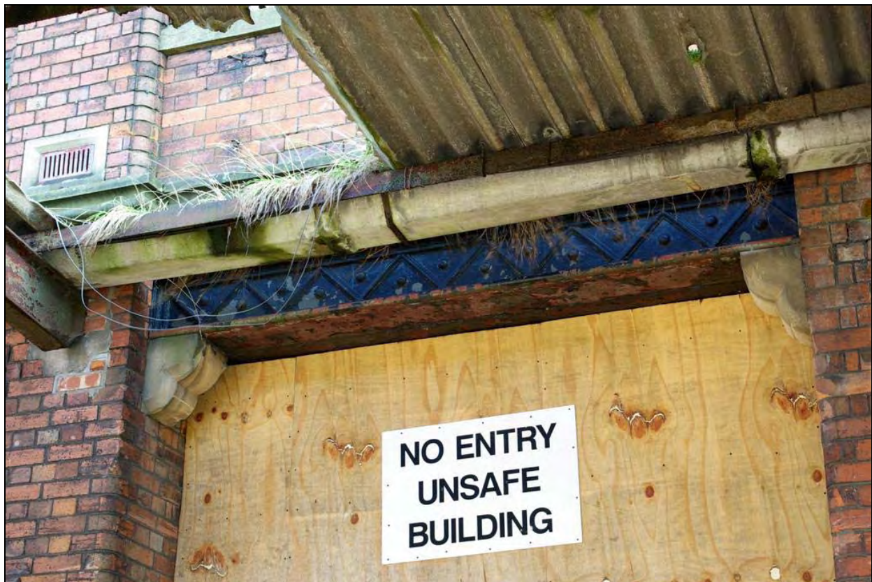
Plate 6: Decorative iron lintels above the apertures on the west elevation
