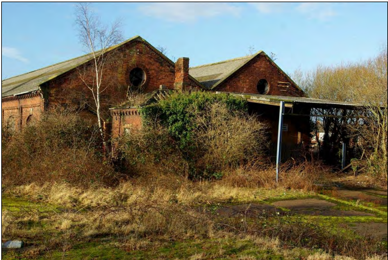
Plate 4: East elevation of the shed showing double pile construction, looking north-west
