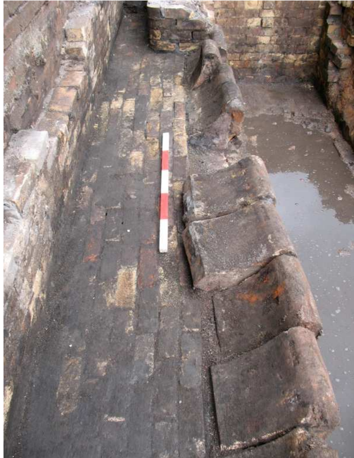
Plate 4: Detail of boiler mounting blocks and the side flue
