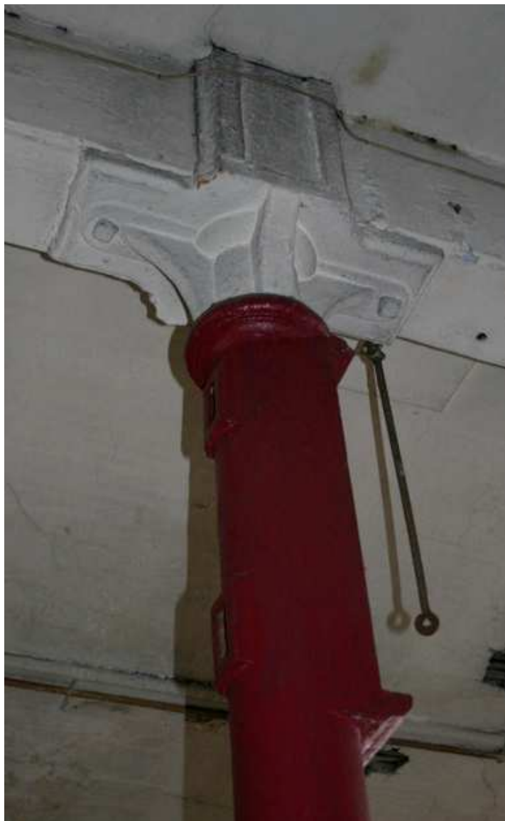
Plate 10: Cast-iron column head detail, second floor, Building A
