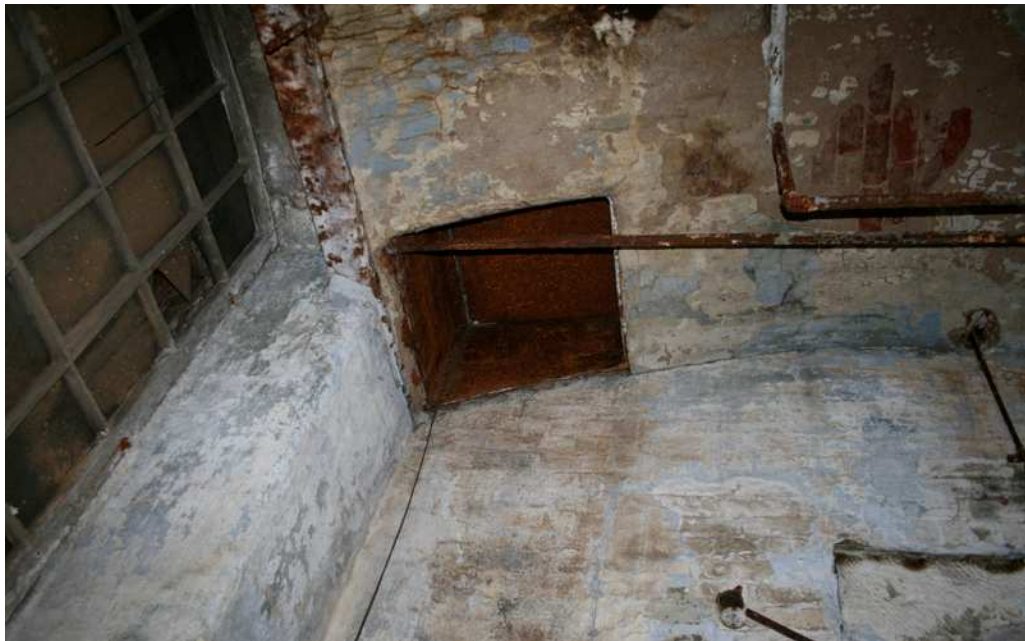
Plate 18: Blocked aperture in vaulted ceiling
