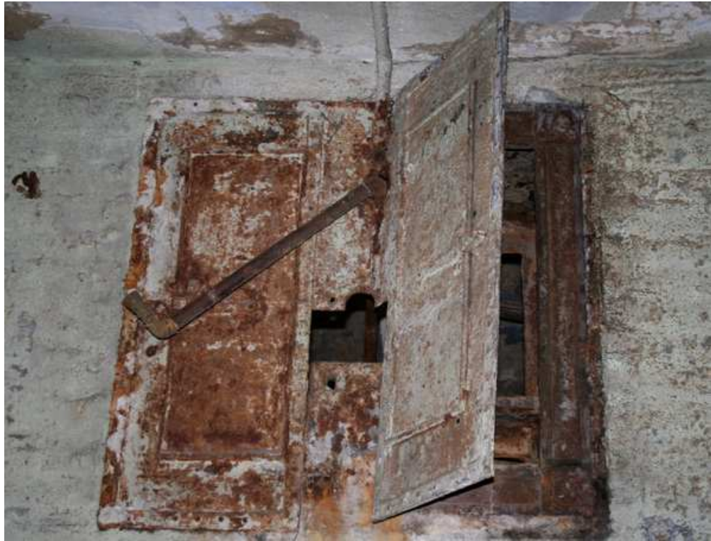
Plate 14: Shuttering on bearing box
