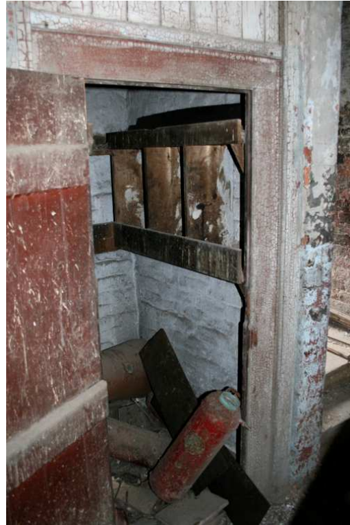
Plate 21: Hoist within the stair newel
