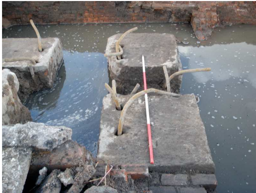
Plate 25: Engine bed, showing fixing bolts
