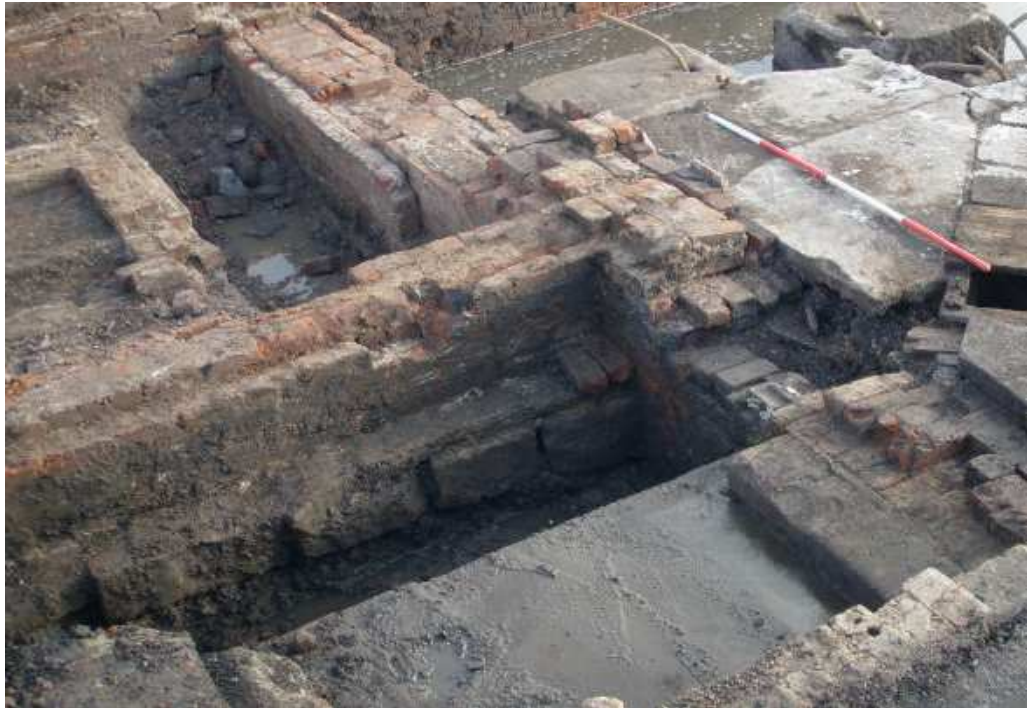
Plate 28: Sandstone footings for stair tower
