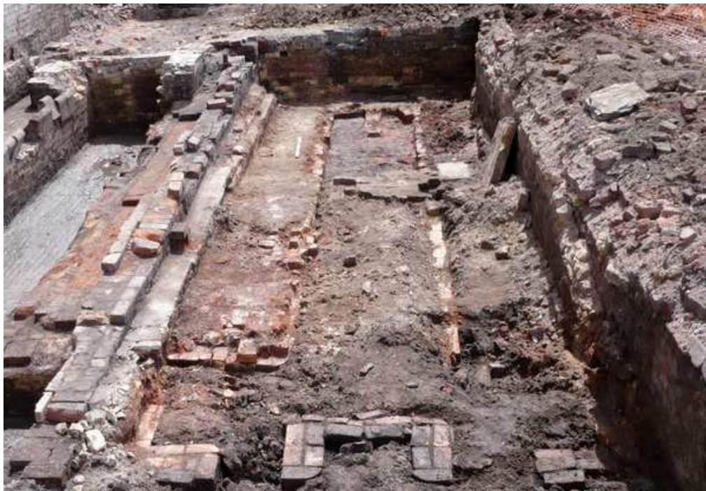
Plate 6: Foundation bed for the Lancashire boiler (Phase 2)
