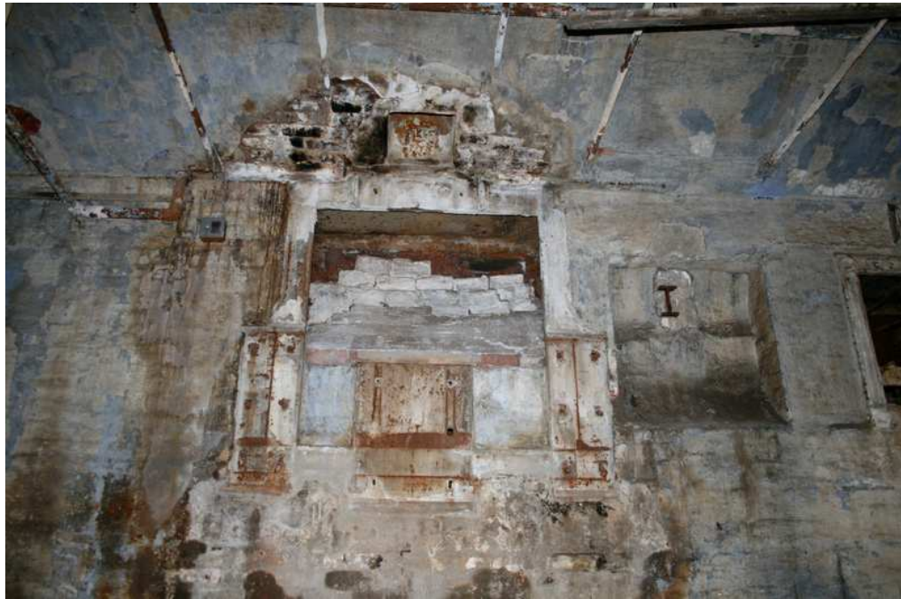
Plate 16: Main footstep bearing, blocked upright shaft aperture and drum cutaway
