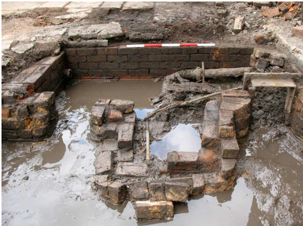
Plate 9: Remodelled 'blow down' and charging platform of Cornish boiler
