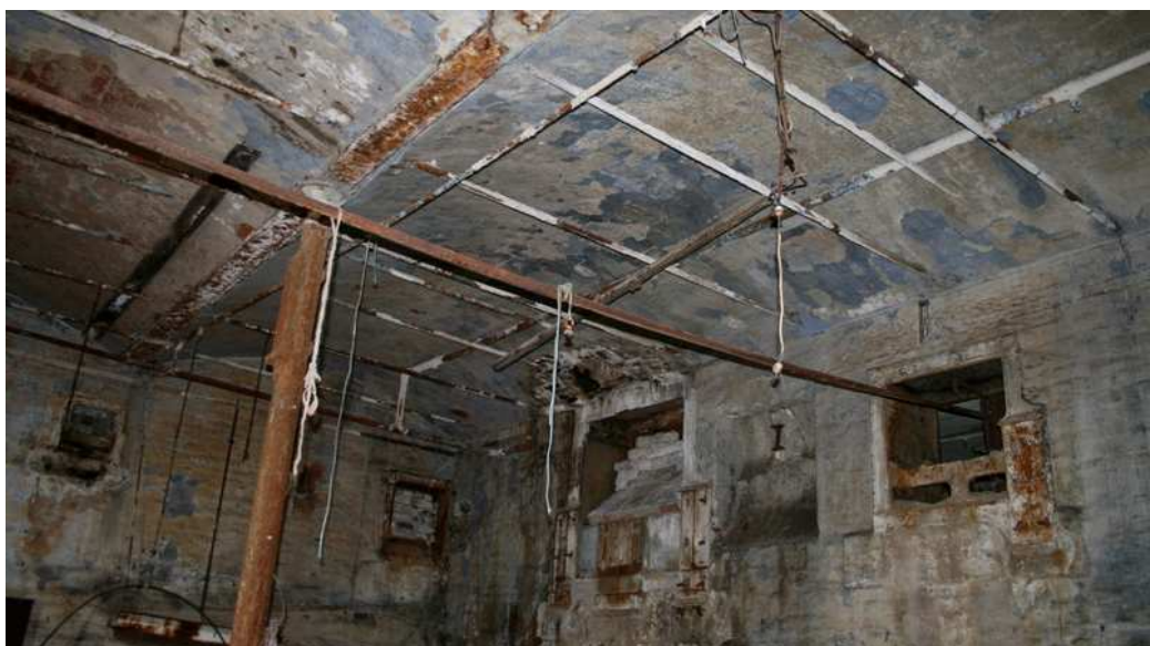
Plate 15: Brick-vaulted ceiling and line shaft carrier bracket, Building A
