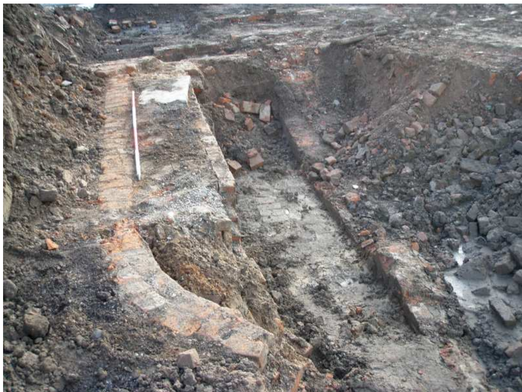
Plate 27: Truncated curving culvert below spinning block
