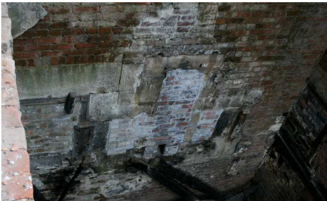
Plate 20: Pinion wheel housing within engine house
