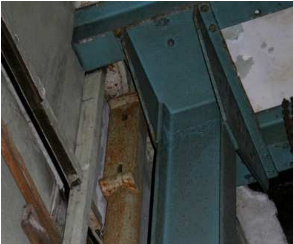
Plate 11: Line shaft hanger casting in column head, first floor, Building A
