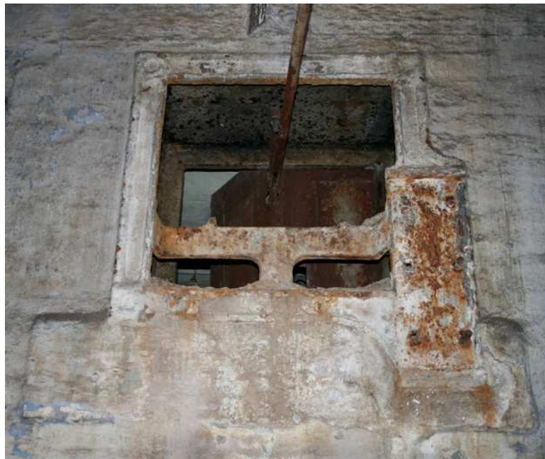
Plate 17: Bearing box for bevel gear
