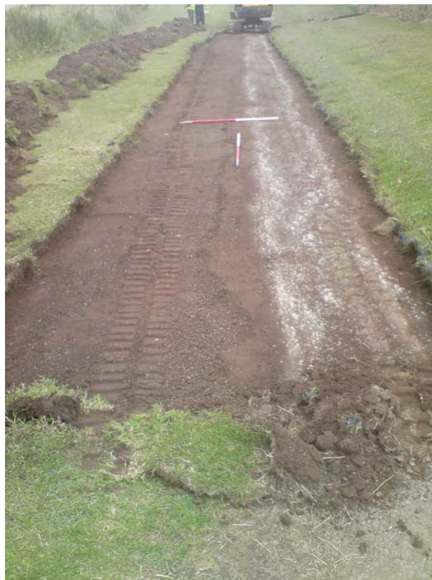
Plate 6: Section 12, facing north-east
