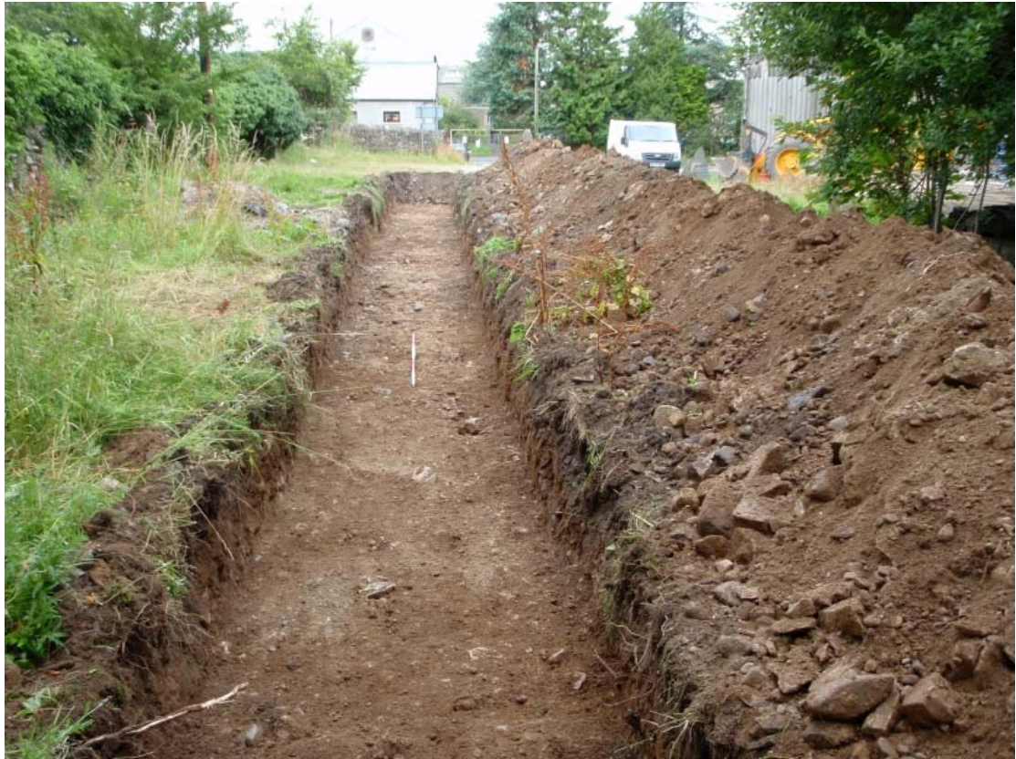
Plate 3: West-facing view of evaluation trench
