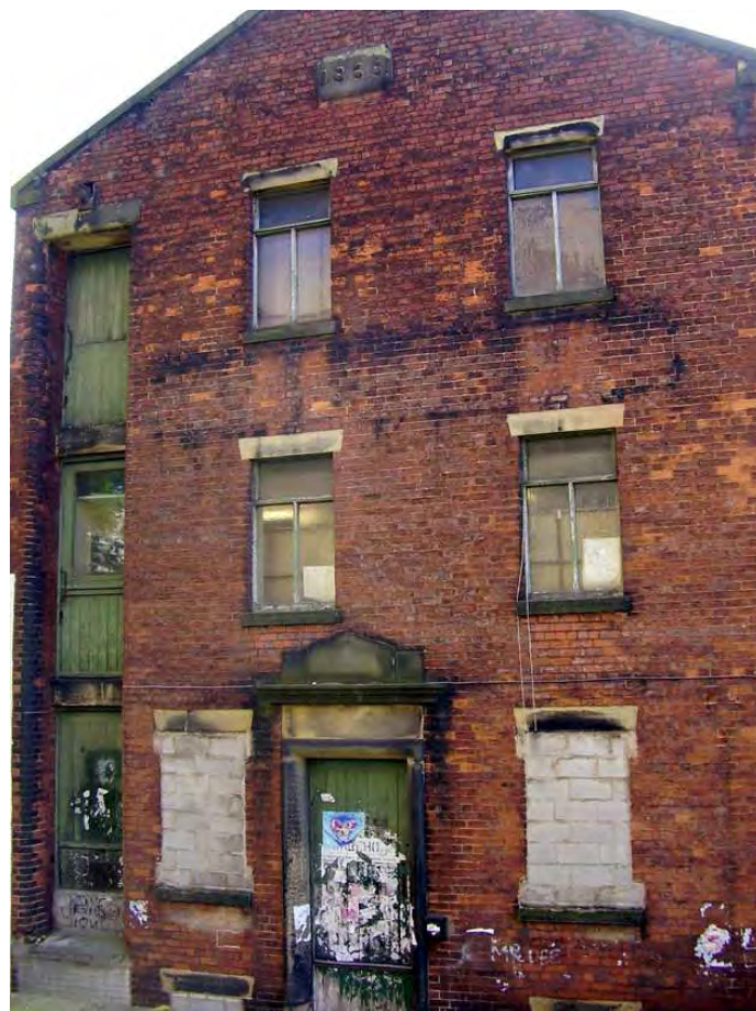
Plate 6: St John's Row. A three-storey warehouse, with a date stone of 1868 (Site 25 )
