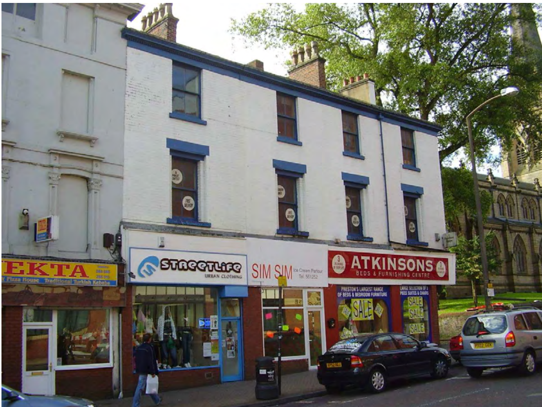
Plate 4: 136 and 138 Church Street (Site 29)
