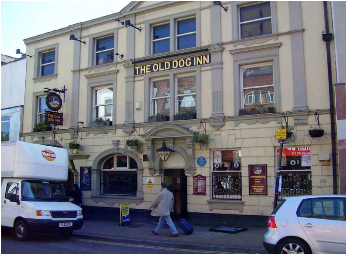
Plate 1: 133 Church Street, The Old Dog Inn (Site 08)
