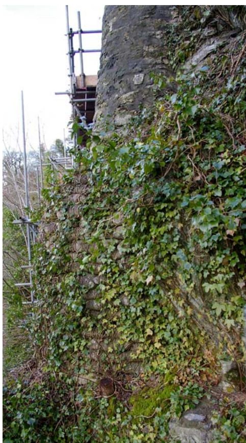
Plate 13: Turret 23 bolstered on the southern and eastern sides by a 2.1m height of concrete-filled sandbags laid around the base of the turret
