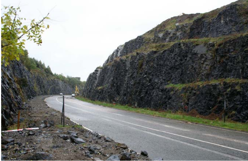
Plate 1: The Glyn Bends Bypass before stabilisation works
