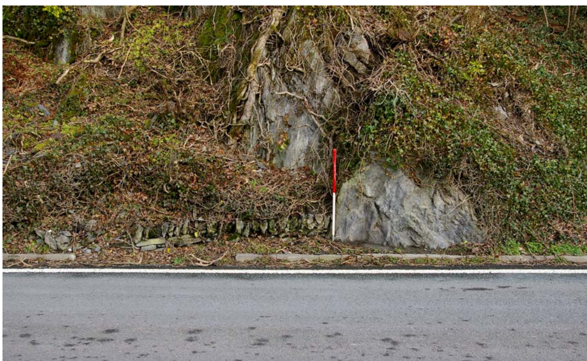
Plate 17: A short section of retaining wall (Site 21 ) at the base of a small quarry (Site 20 )
