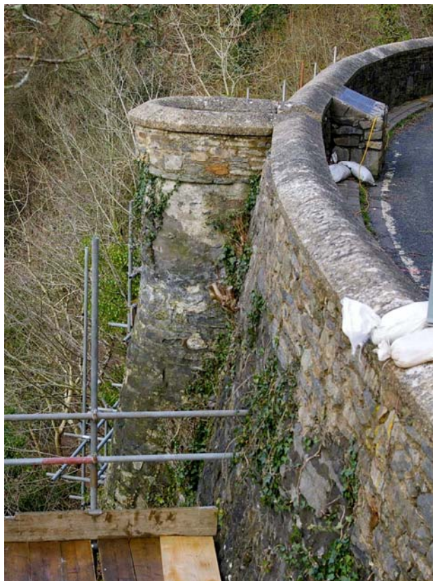
Plate 12: Turret 23 viewed from the east
