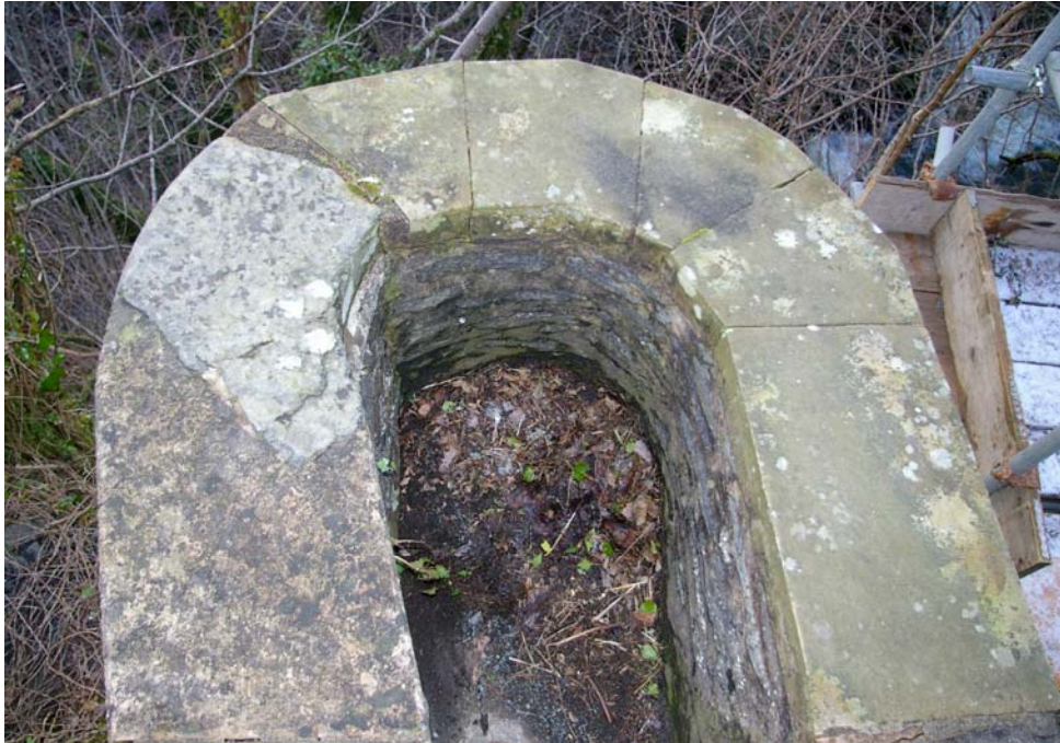
Plate 10: The horse-shoe shape of the western viewpoint turret (Site 10 ) with an original coping stone to the south
