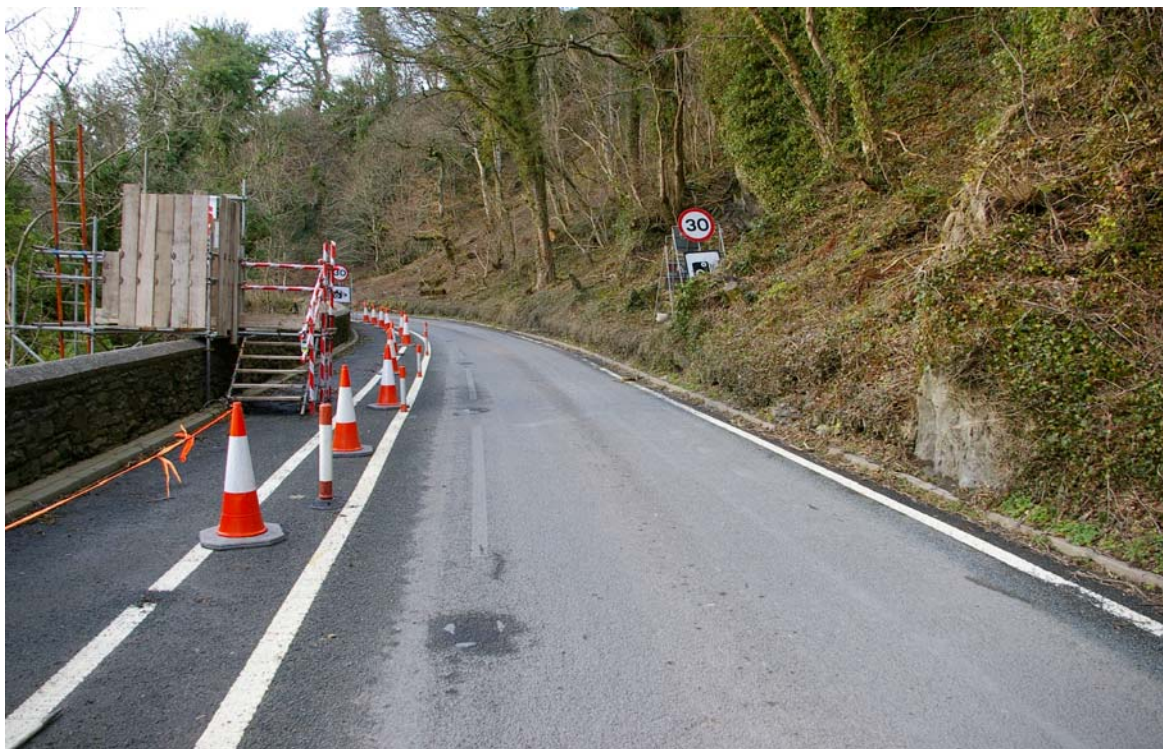
Plate 16: The well-preserved section of retaining wall - Site 18 , separated from Wall 17 by a small crag
