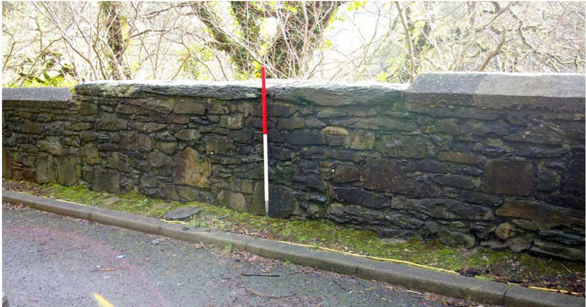
Plate 4: The original slate topstones have been replaced on a later rebuild of the parapet (Site 02)
