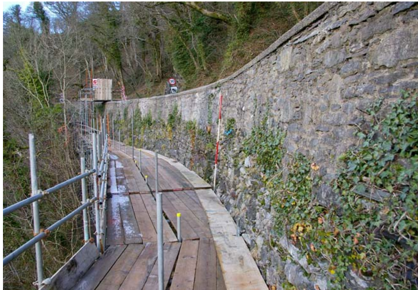
Plate 2: The random rubble build of the embankment wall (Section Site 01)
