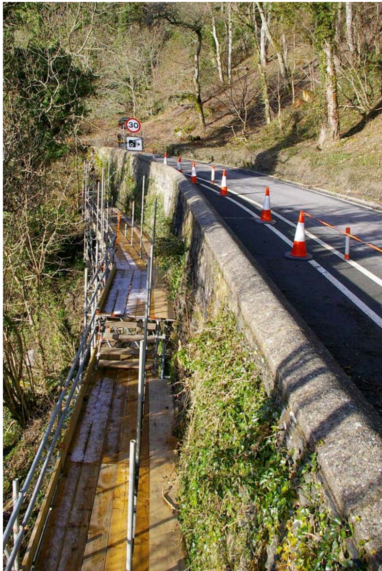
Plate 5: Section 03 of the embankment wall showing the concrete copings on the rebuilt parapet wall
