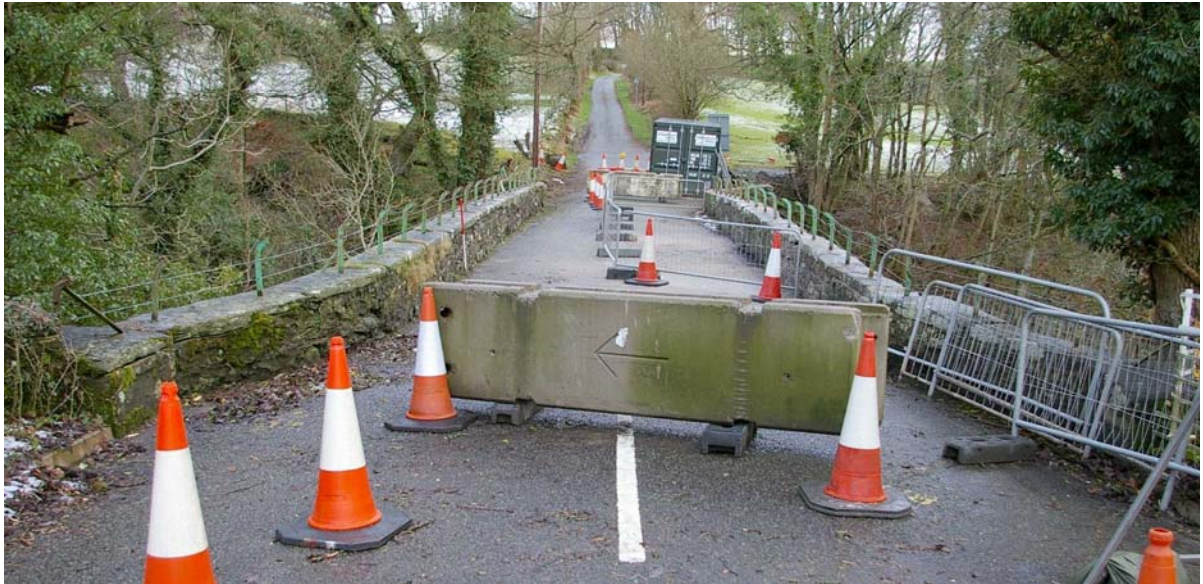
Plate 8: The top of the turnpike bridge (Site 05), looking south
