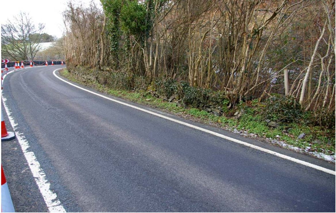
Plate 18: The longest section of retaining wall (Site 24 ) at the eastern end of the embanked road section
