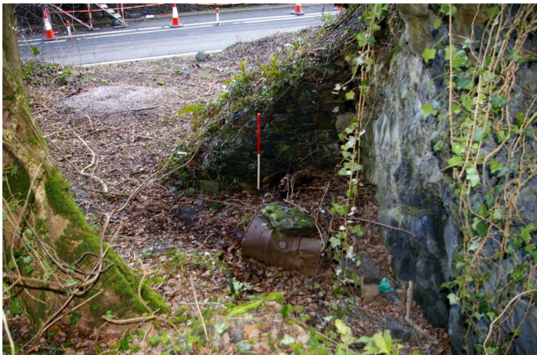
Plate 20: Decayed dry-stone structure (Site 13 ), set within a quarry (Site 12 )
