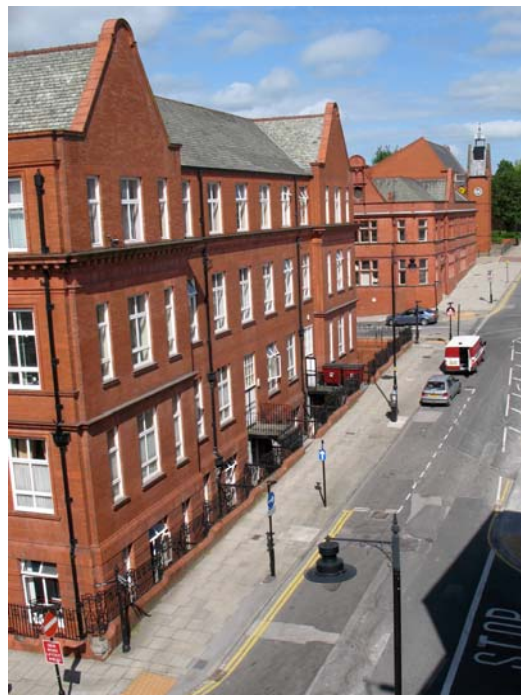
Plate 5: The Town Hall, with cellar lights
