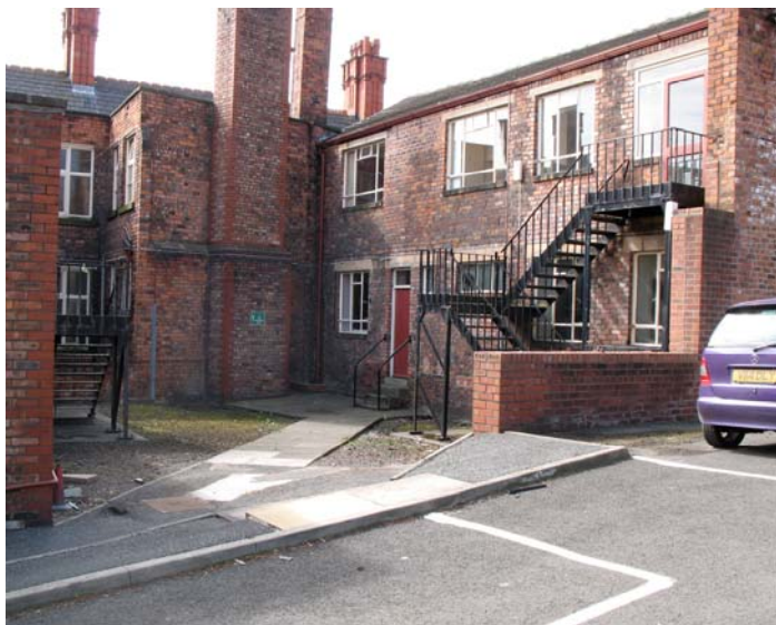
Plate 7: Area between wing to north of Municipal Building
