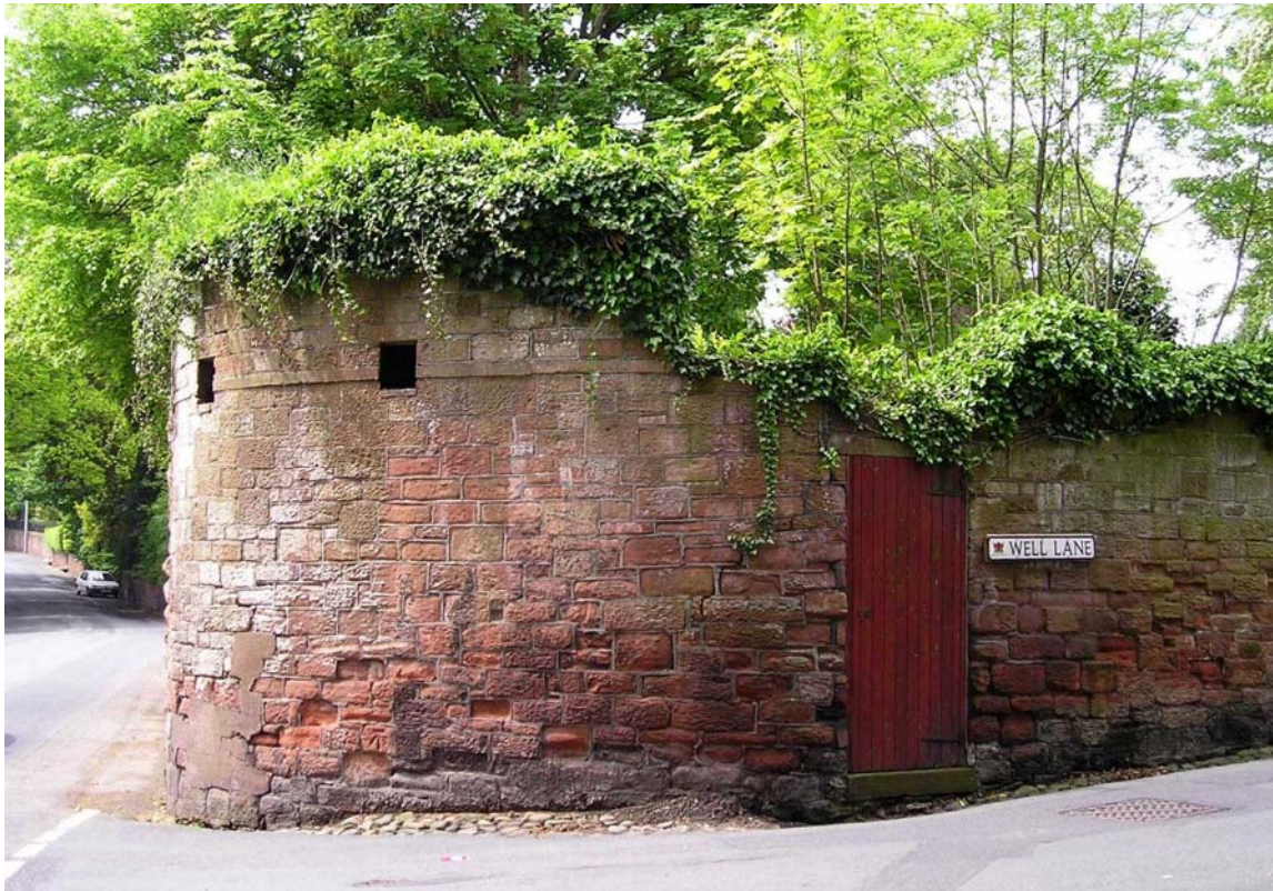
Plate 12: World War II pillbox in a wall at the junction of Brampton Road and Well Lane, Stanwix (M84)
