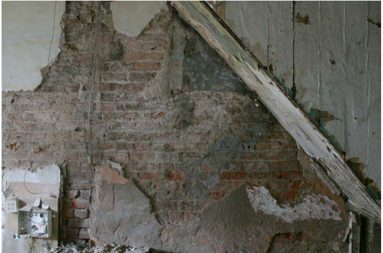
Plate 7: Wall scar of original stairs and later partition, 34 Oldham Road
