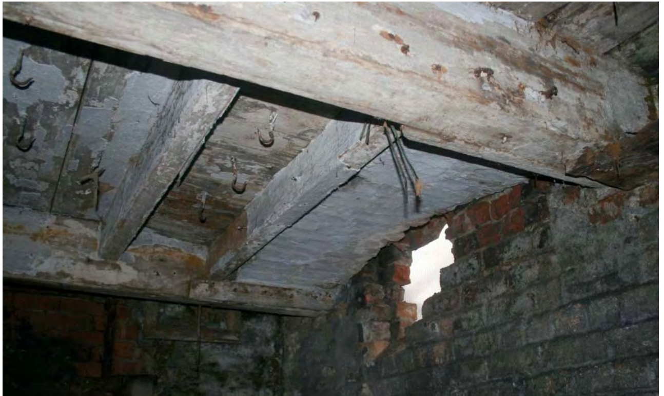
Plate 14: Brick vault within cellar, 34 Oldham Road
