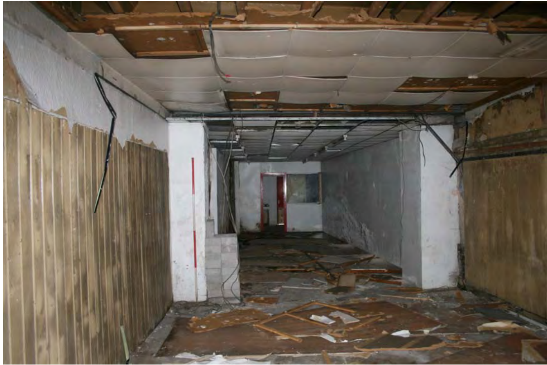
Plate 15: Timber panelling and rebuilt rear section of 36 Oldham Road
