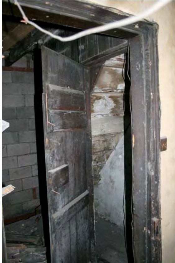
Plate 21: Understair cupboard, first floor, 36 Oldham Road
