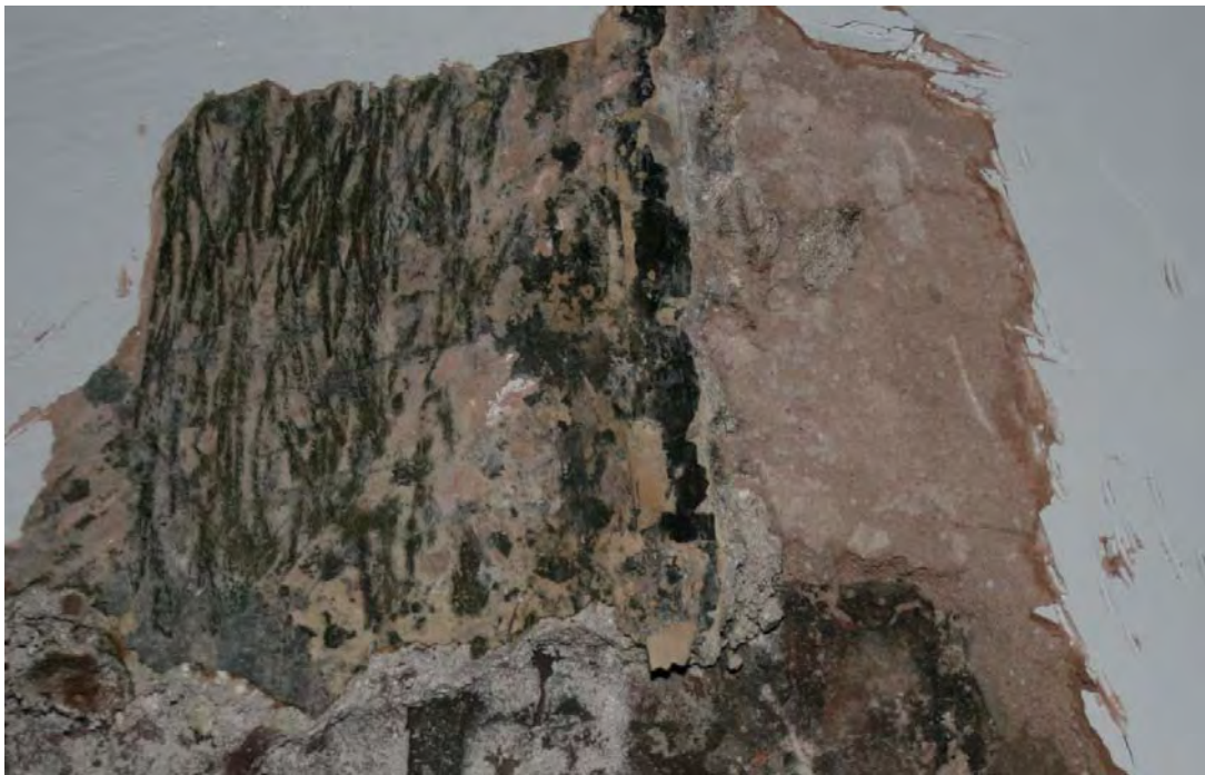
Plate 10: Straight joint between early plaster around chimney breast and late mid-brown plaster, 34 Oldham Road
