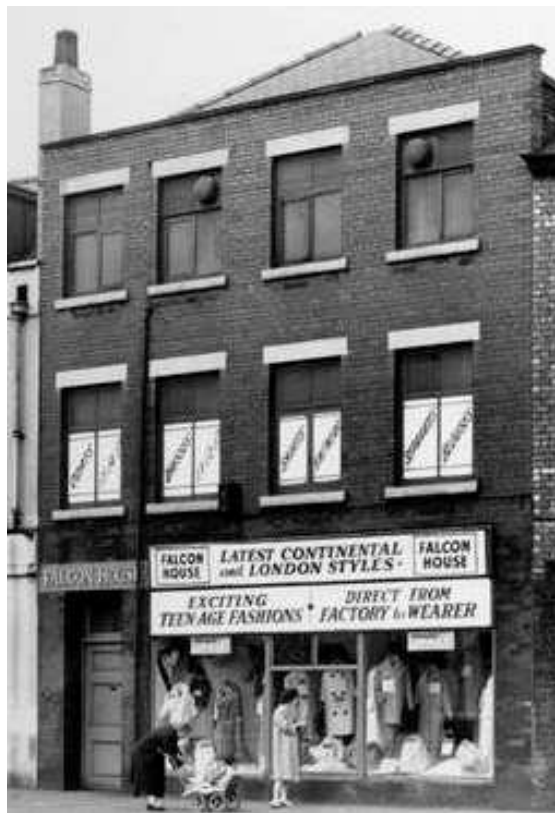
No 38 Oldham Road in 1961
