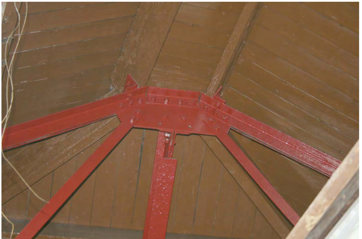
Plate 28: Detail of flat ridge section, 38 Oldham Road
