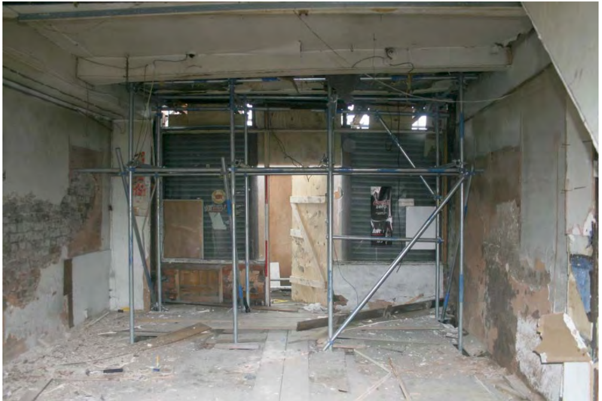
Plate 5: Internal view of ground floor, 34 Oldham Road
