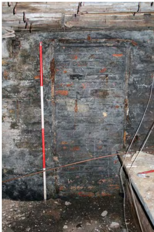
Plate 12: Blocked doorway between cellars of 34 and 36 Oldham Road
