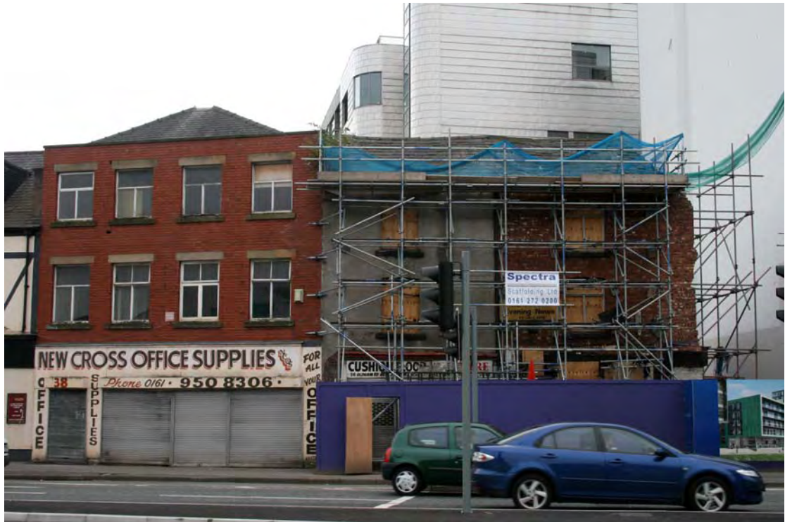
Plate 1: Nos 32-38 Oldham Road
