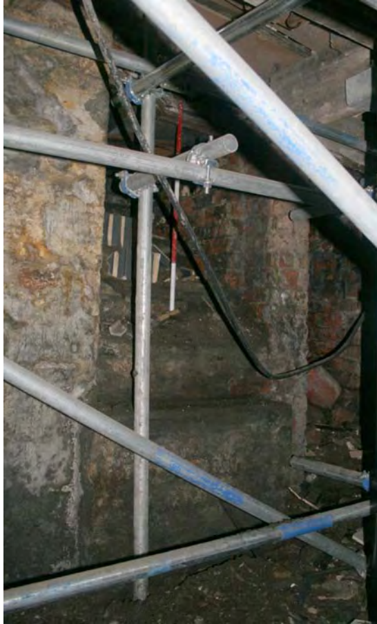
Plate 11: Steps in cellar, 34 Oldham Road
