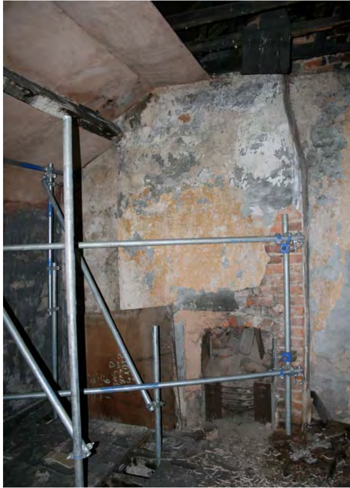
Plate 23: Tapered chimney breast, second floor, 36 Oldham Road
