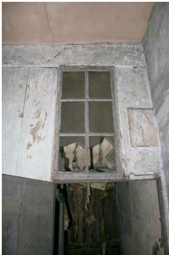
Plate 26: Skylight above stairwell, second floor, 36 Oldham Road
