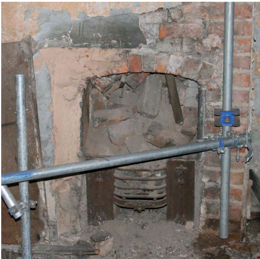
Plate 22: In-situ decorated fireplace, second floor, 36 Oldham Road
