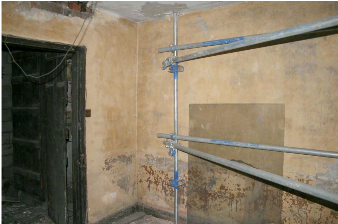
Plate 18: Painted wall plaster, skirting board and architrave, 36 Oldham Road
