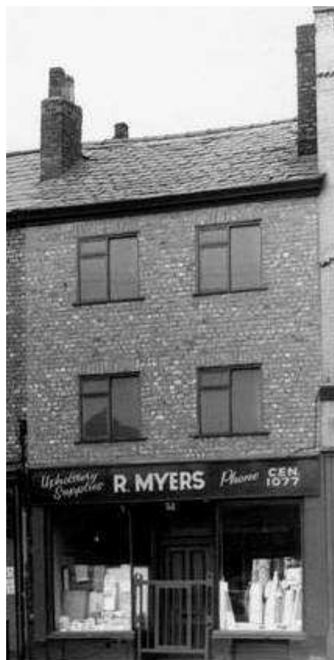
No 32 Oldham Road in 1961
