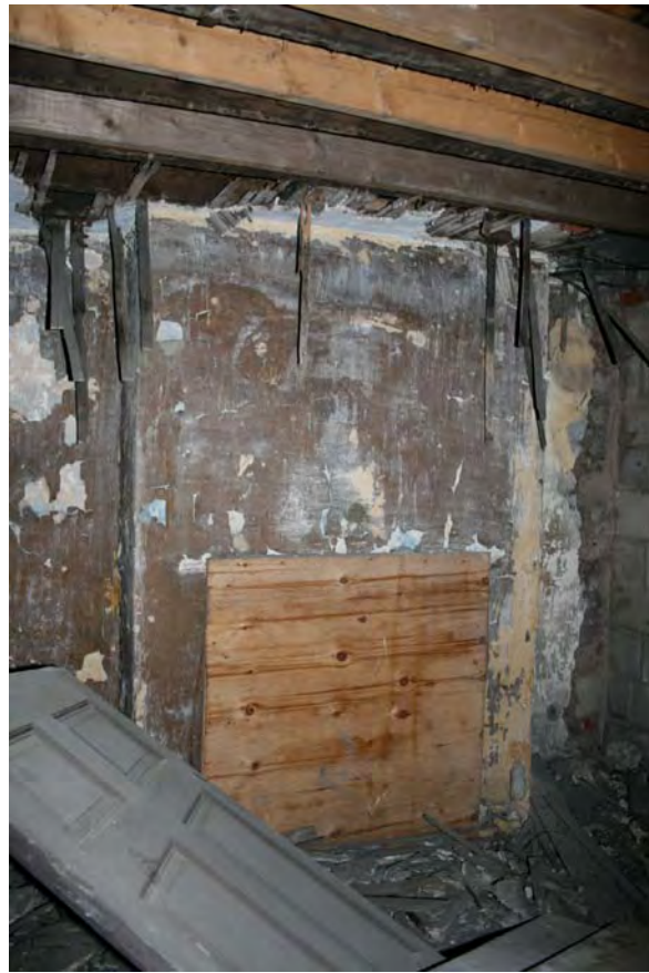
Plate 19: Intact chimney breast, first floor, 36 Oldham Road
