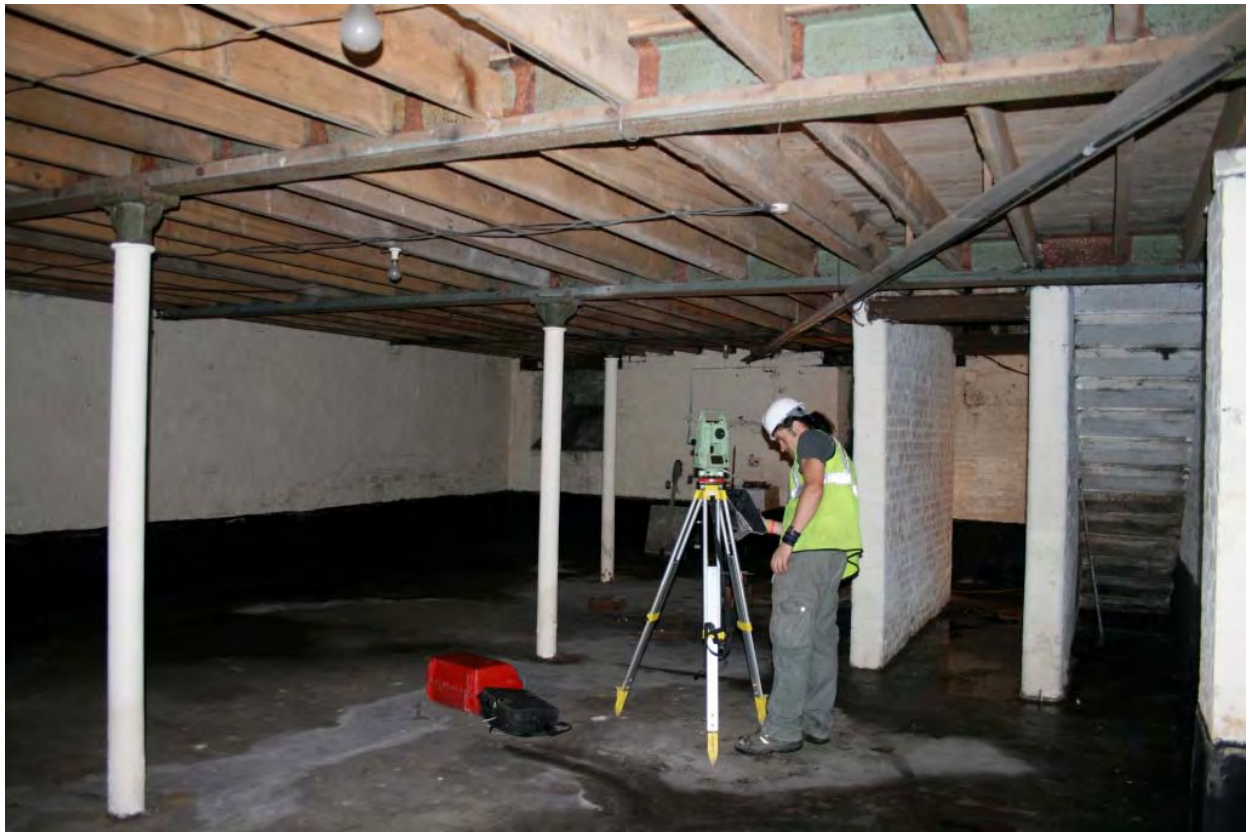
Plate 31: Stair walls and columns, basement, 38 Oldham Road
