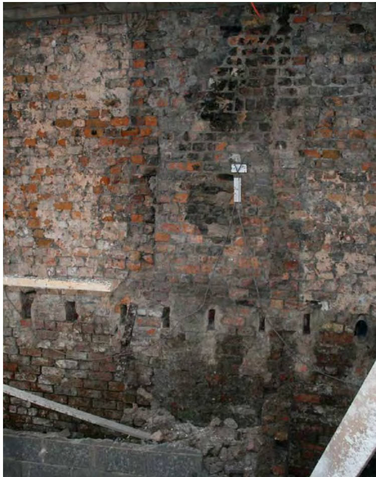
Plate 4: Floor joist sockets and fireplace scars, 32 Oldham Road
