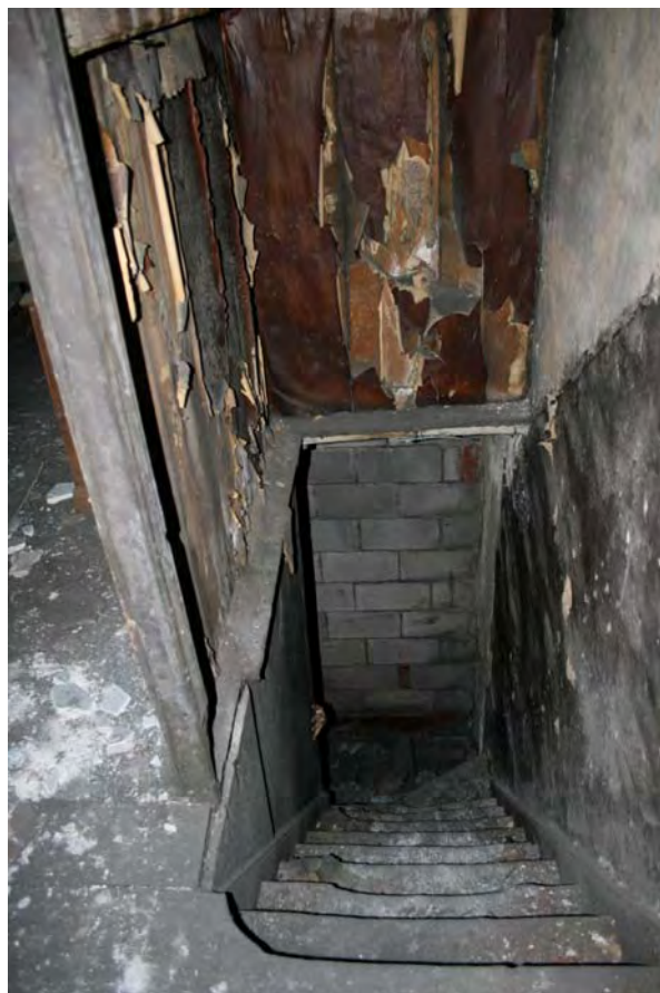
Plate 20: Stair between first and second floors, 36 Oldham Road
