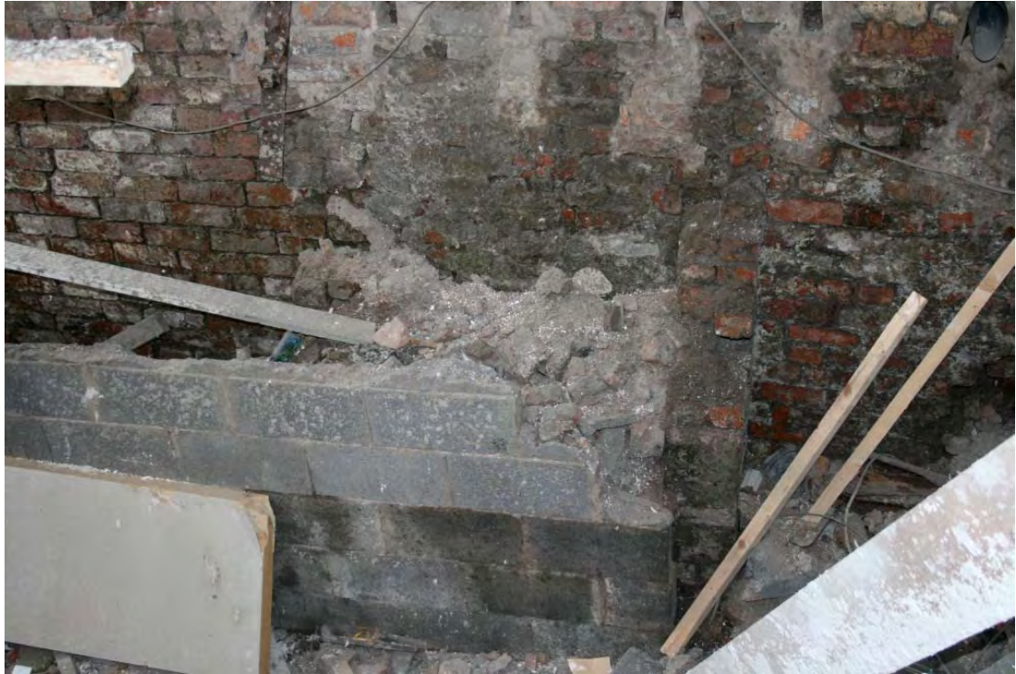
Plate 3: Fireplace within cellar, 32 Oldham Road
