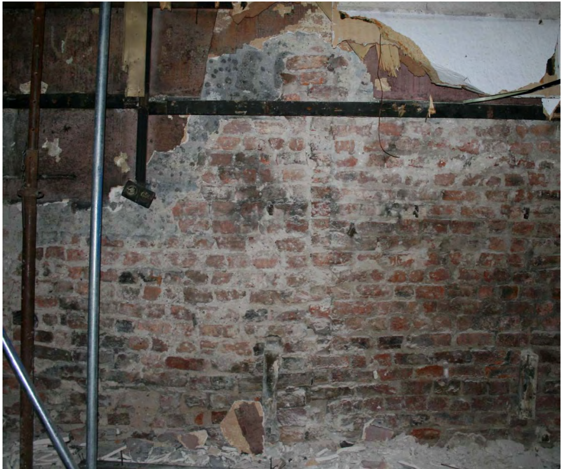
Plate 17: Wall scar of removed internal partition, 36 Oldham Road
