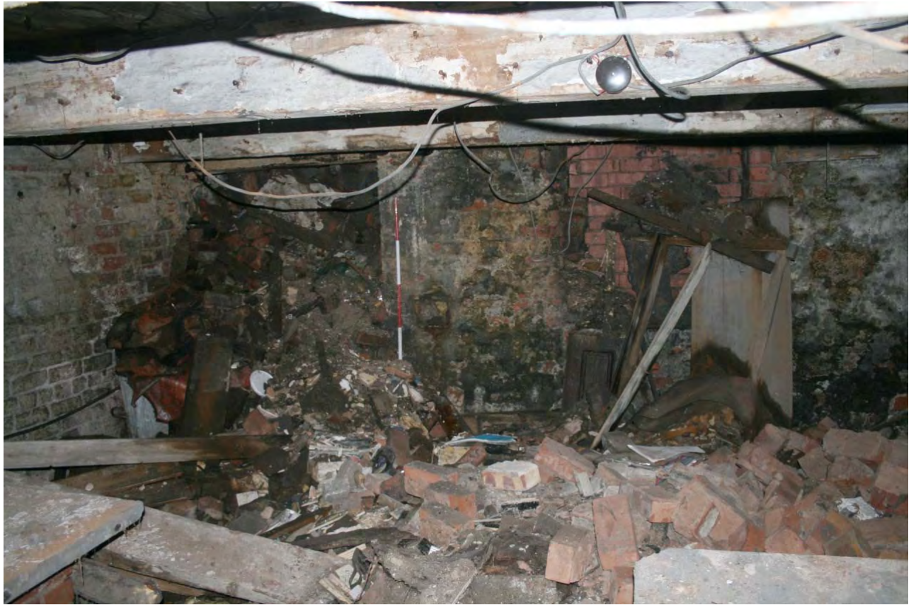
Plate 13: Rear of cellar, 34 Oldham Road
