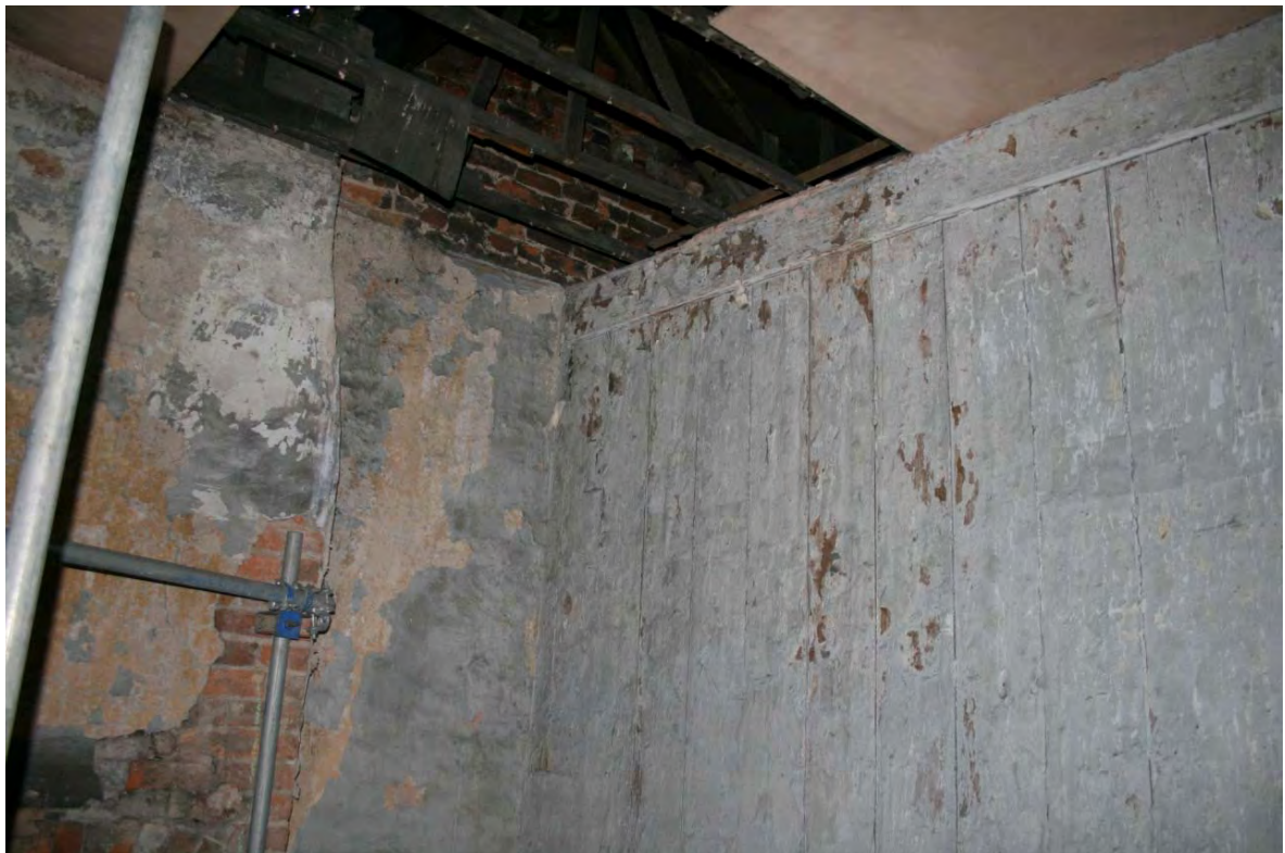
Plate 24: Timber partition, second floor, 36 Oldham Road
