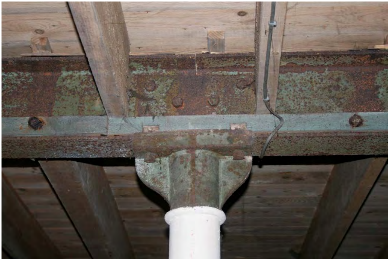
Plate 32: Column cap detail, basement, 38 Oldham Road
