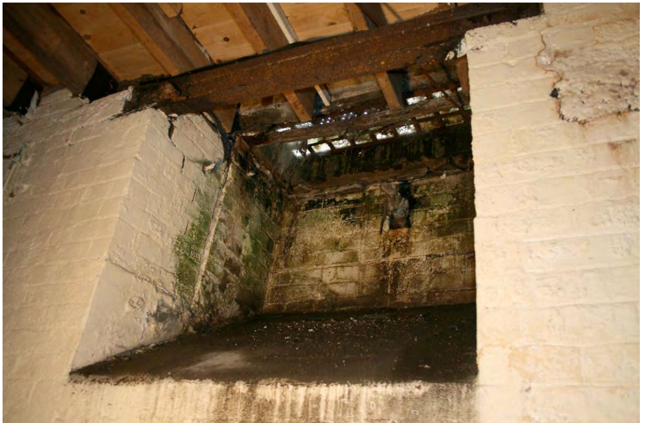
Plate 30: Remodelled pavement light, basement, 38 Oldham Road
