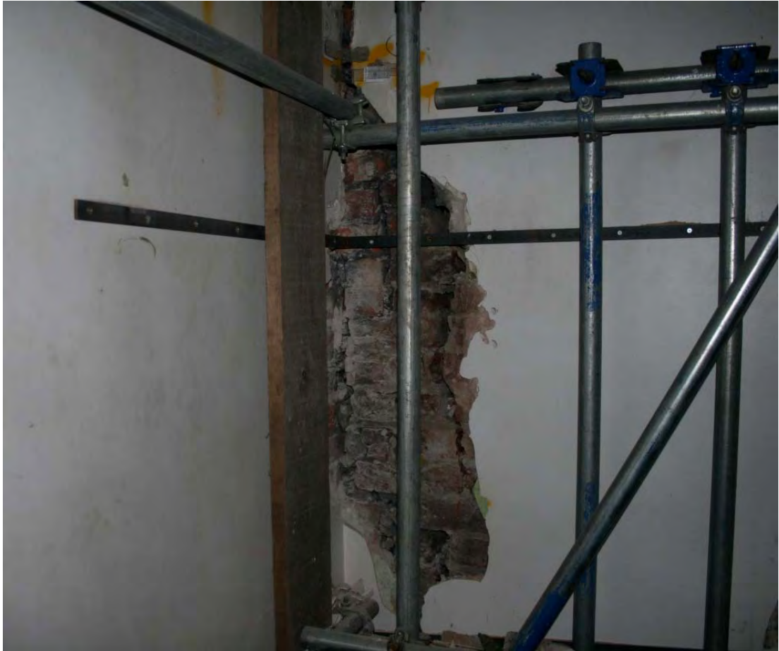
Plate 9: Rebuilt facade (left) butting broken end of original wall, 34 Oldham Road
