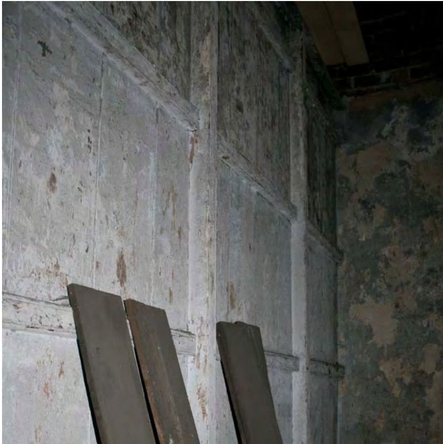
Plate 25: Beaded studs on rear of panelling, second floor, 36 Oldham Road
