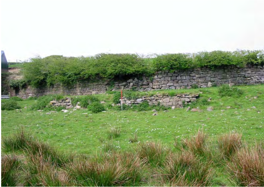
Plate 29: Site 46 , mill pond revetment wall remains at Scale Bank
