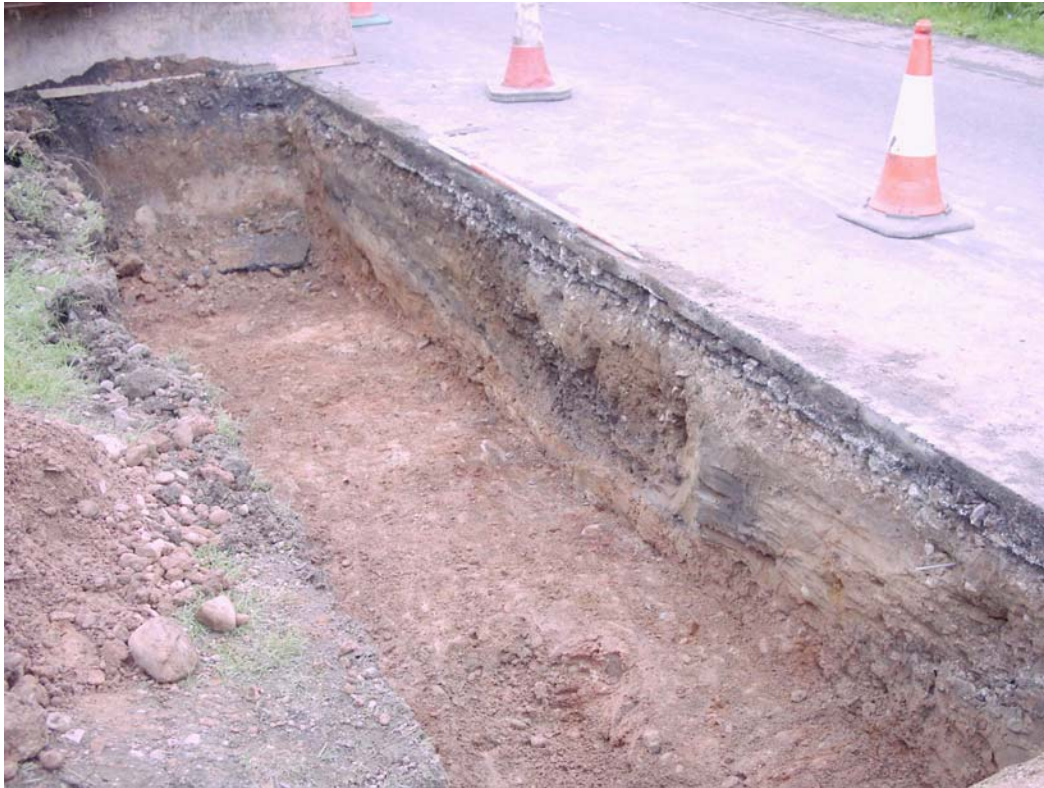
Plate 11: North-east-facing section of Site D, Trench 2, showing Ditch 62I , and compacted layer 620/626
