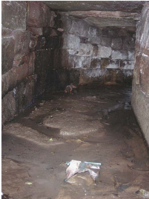
Plate 8: Intact section of culvert 738/739 , adjacent to Site A, looking north-east
