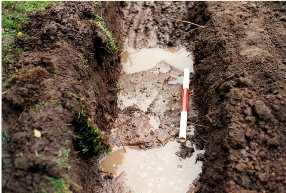
Plate 1: Culvert 103 , looking north
