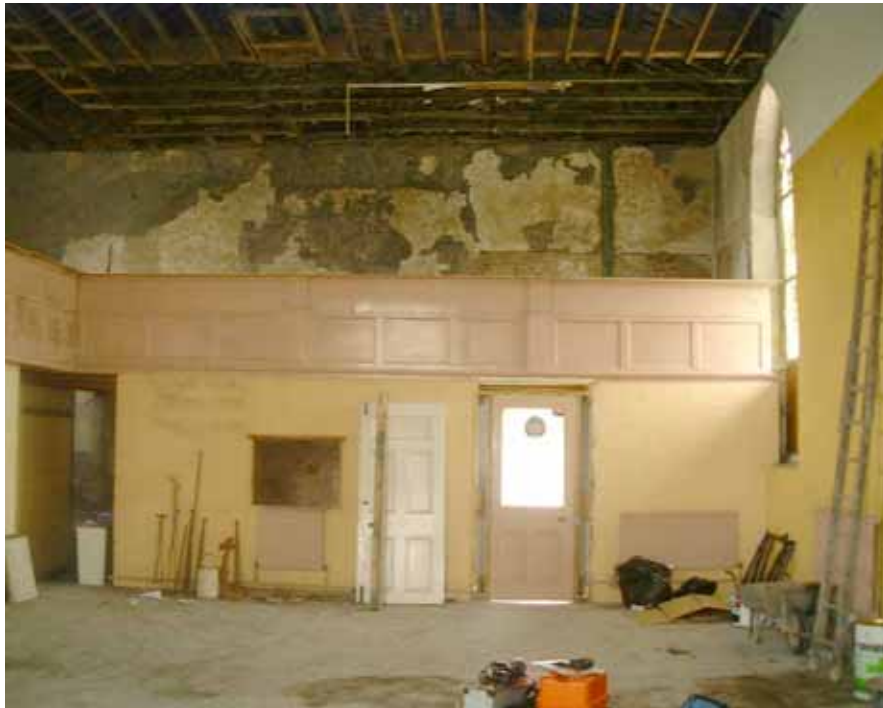
Plate 2: East-facing wall of the gallery
