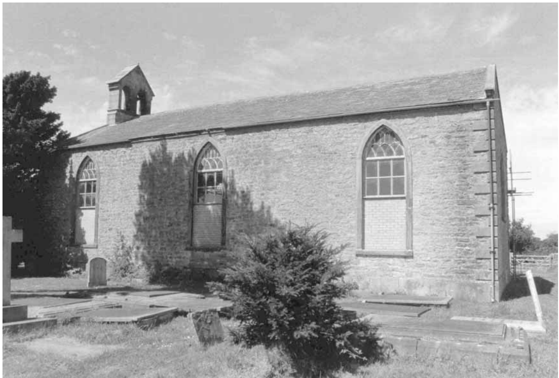
Plate 8: South-facing external elevation
