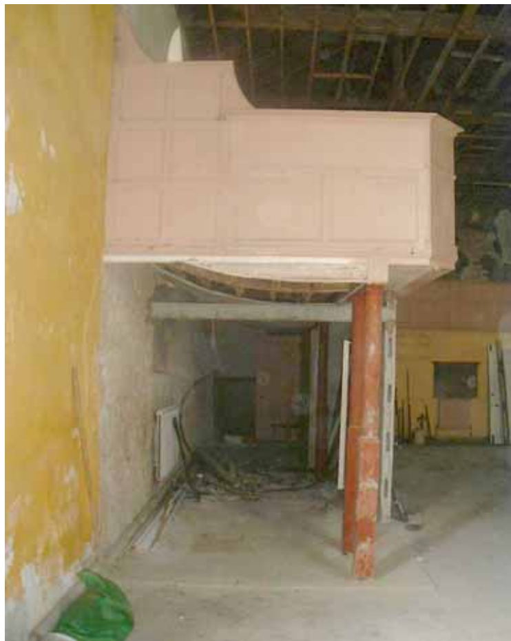
Plate 4: East end of the south side of the gallery
