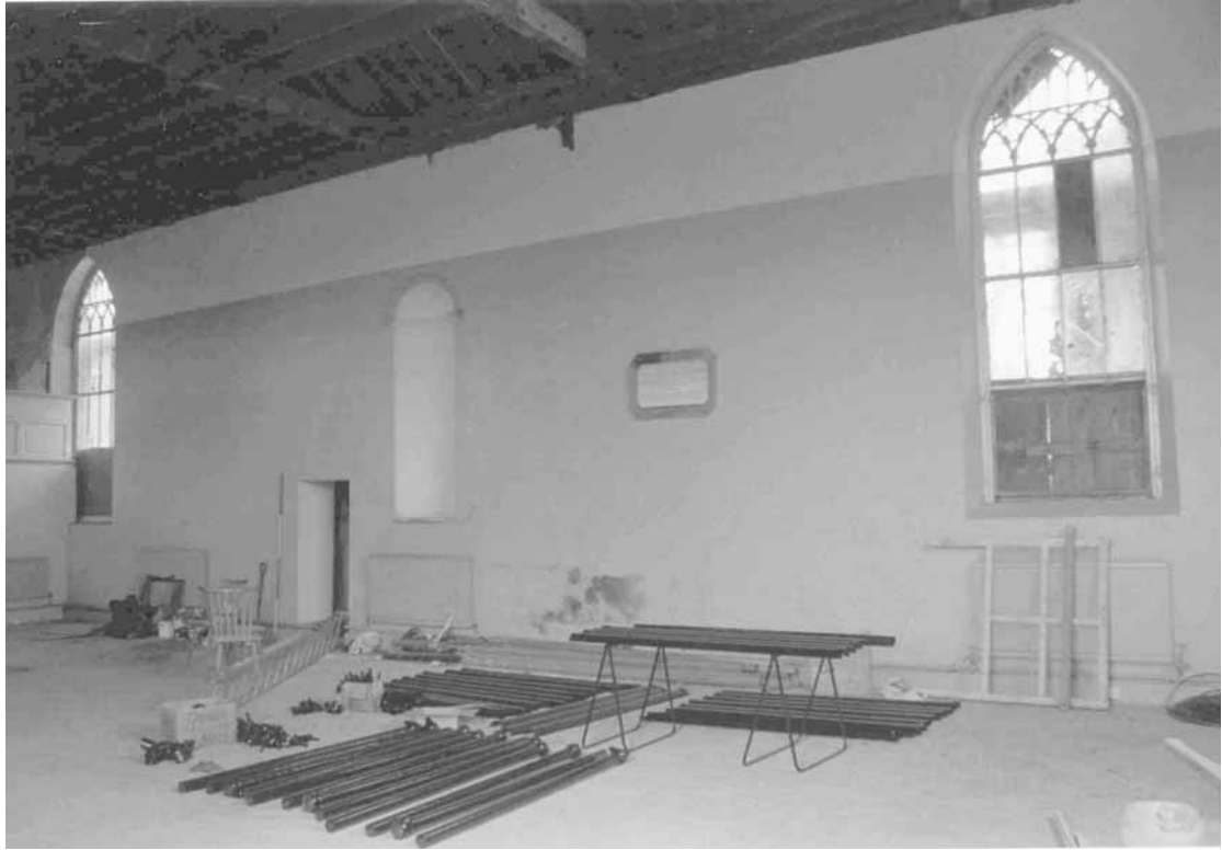
Plate 5: South-facing internal elevation of the nave
