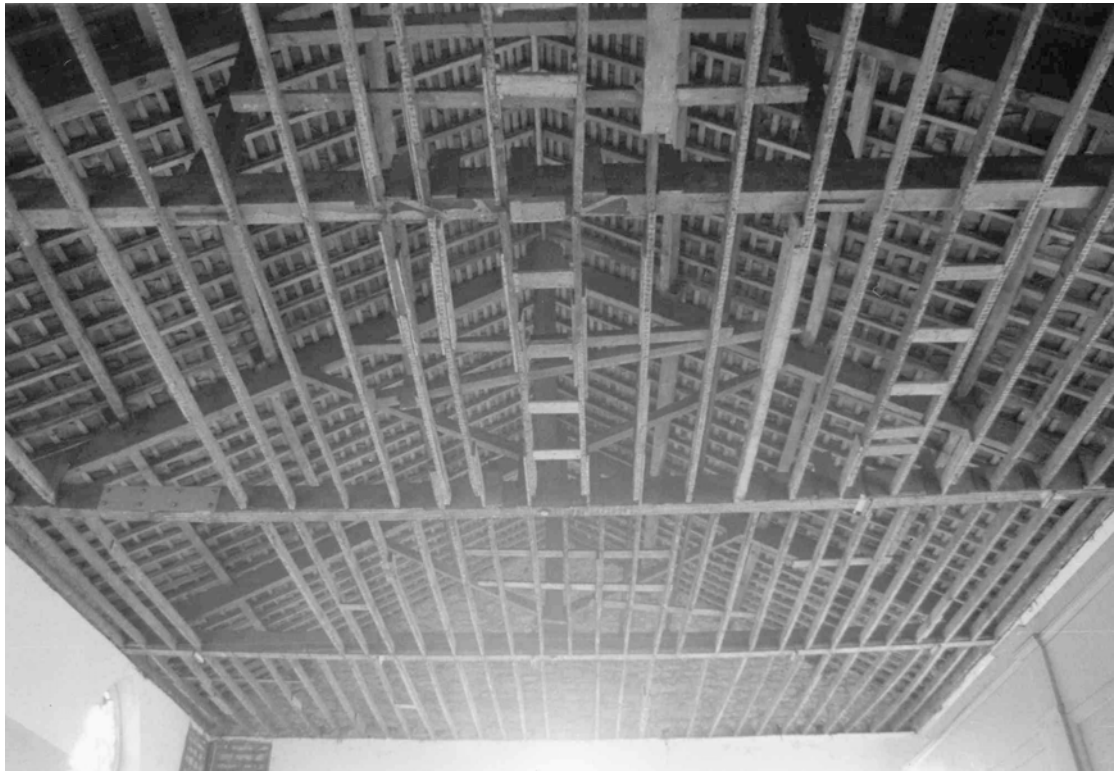
Plate 6: Roof Structure, facing East
