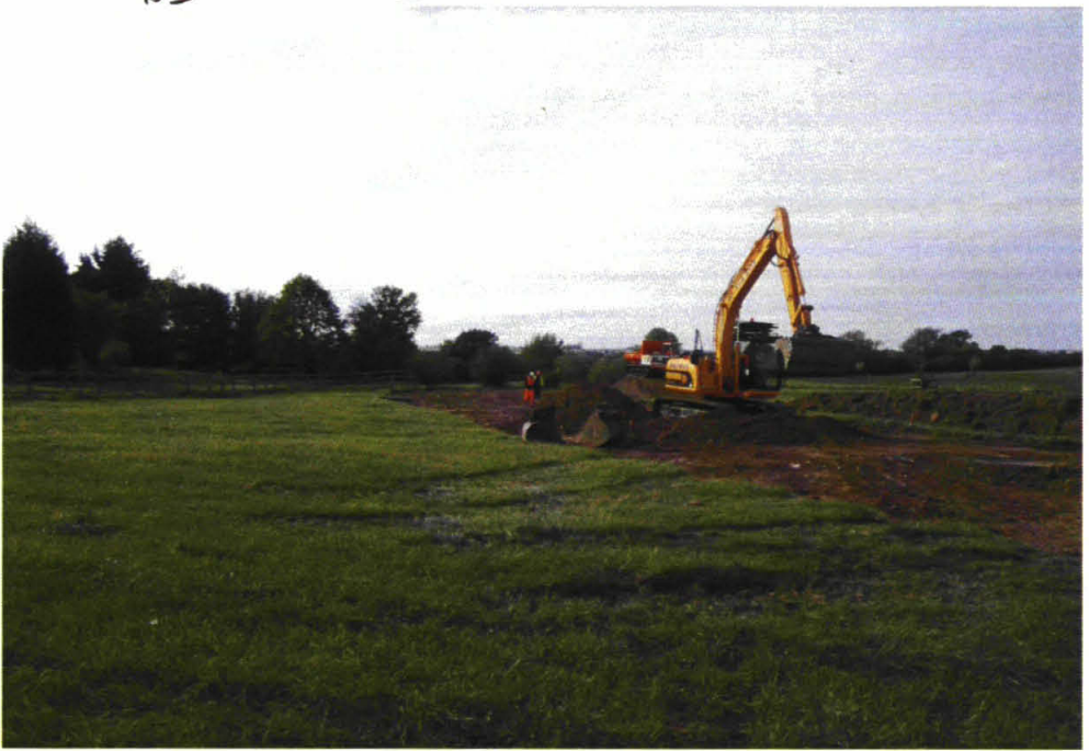
10) 009.jpg Working shot, topsoil strip → SW
