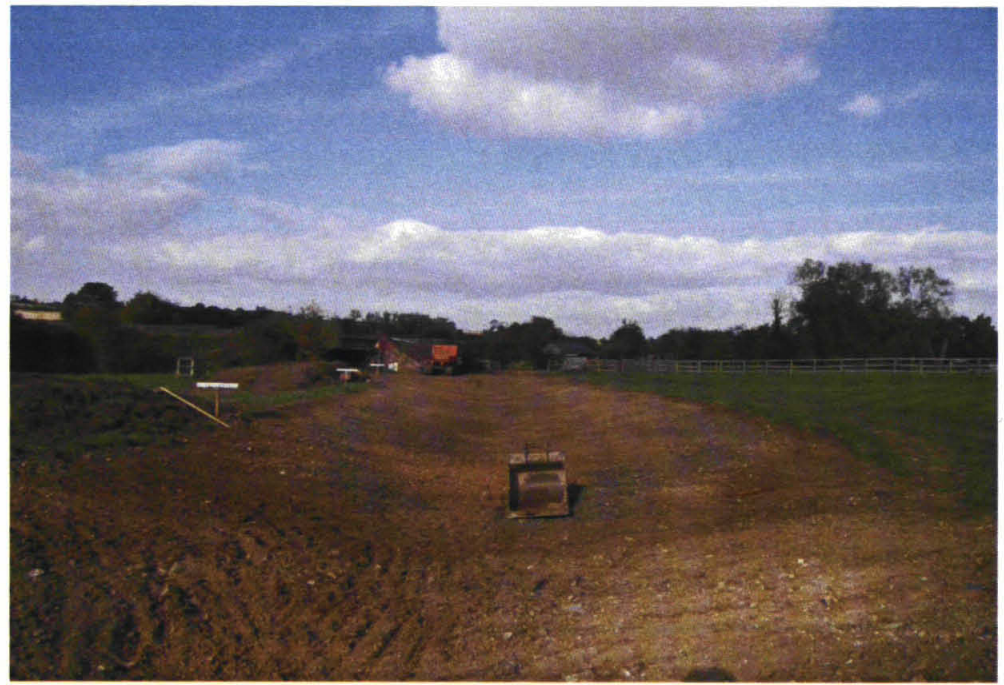
31) 30.jpg Finished length of swale \rightarrow NW
