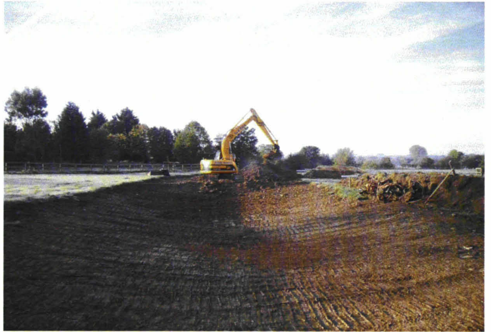
24) 023.jpg Excavation of the site → SW
