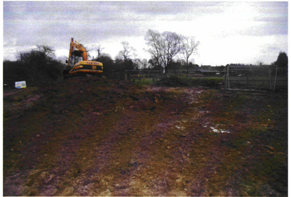
44) 044.jpg Construction of northern bond → NE
