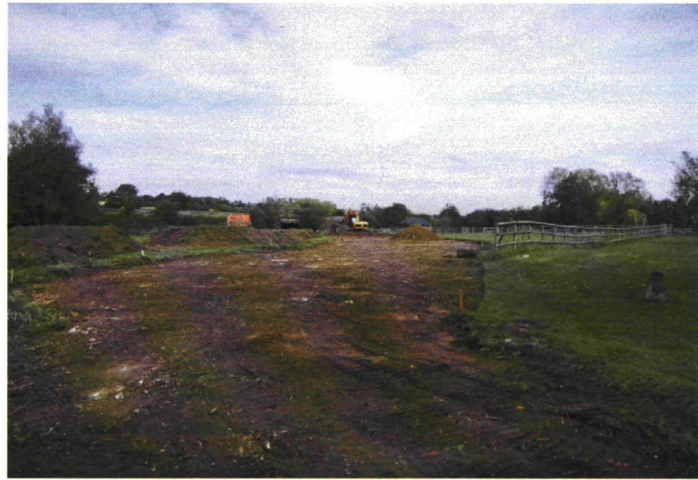
13) 012.jpg Post-ex view of trench strip → NE
