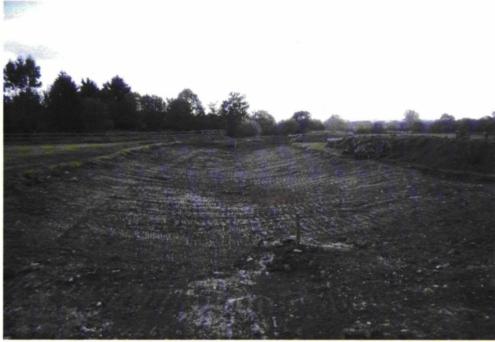
34) 033.jpg Finished length of swale → SE
