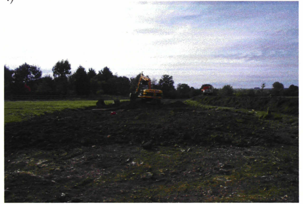
4) 003.jpg Topsoil strip for swale → SW
