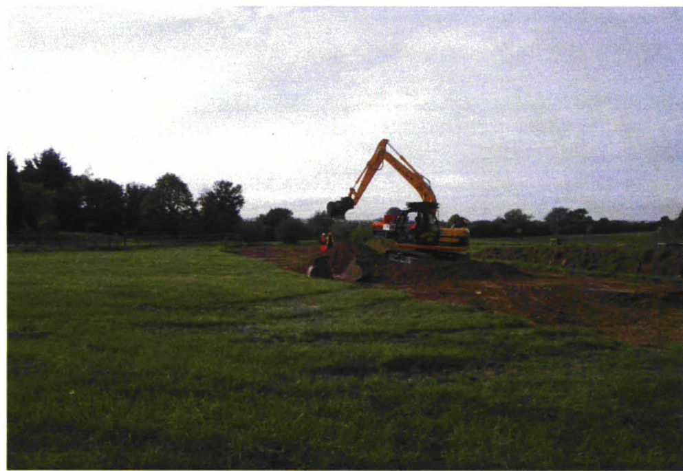
11) 010.jpg Working shot, topsoil strip → SW
