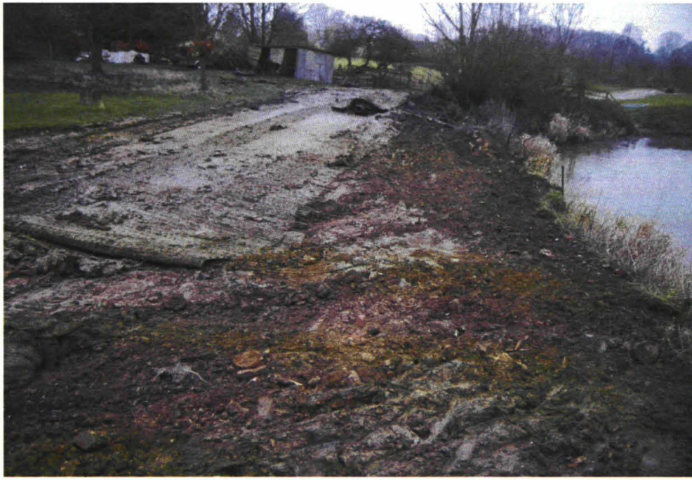
45)045.jpg Connection of the swale to the evenlode
