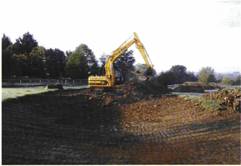
26) 025.jpg Excavation of swale → SW
