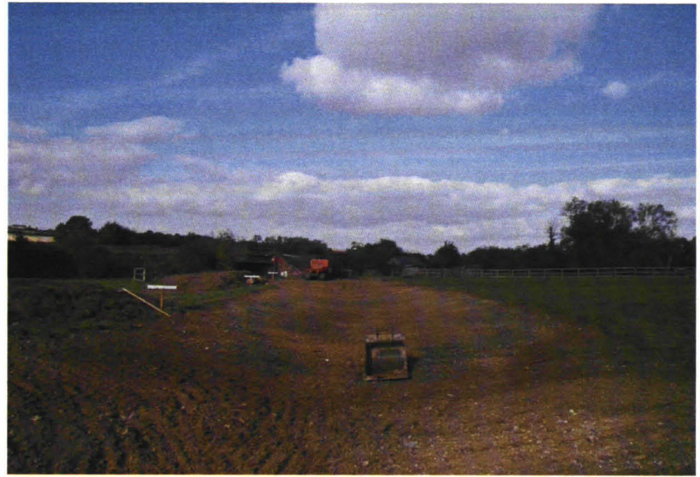
32) 031.jpg Finished length of swale \rightarrow NW
