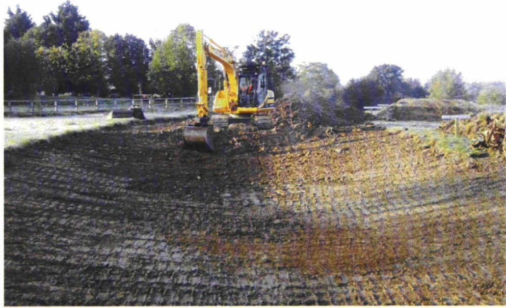
25) 024.jpg Excavation of swale → SW
