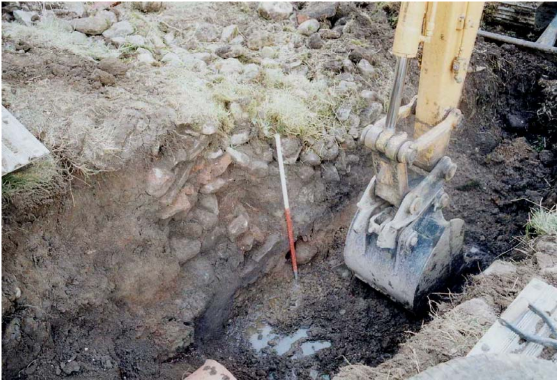
Plate 5: View of Mill Race wall as seen in Trench 2
