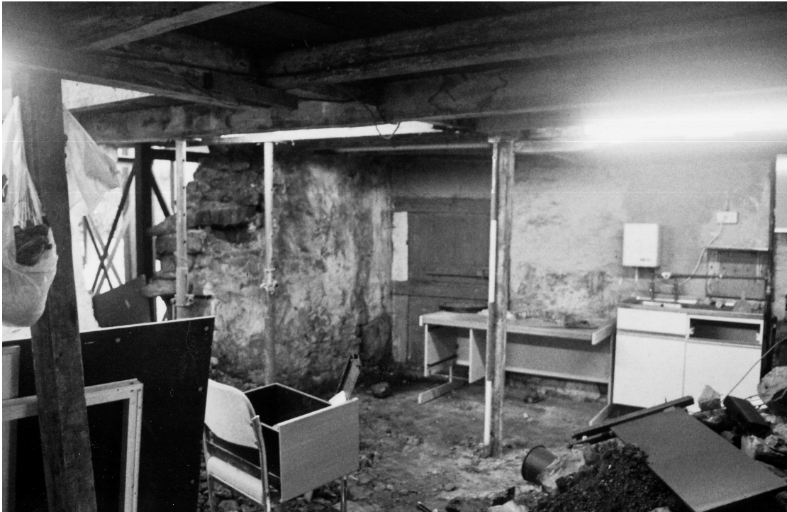
Plate 7: Room 3, looking southwest
