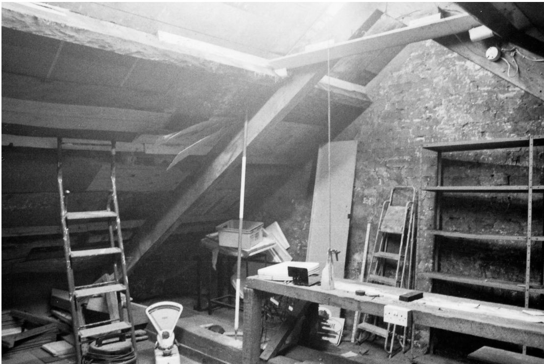
Plate 8: Truss in Room 10, looking southwest
