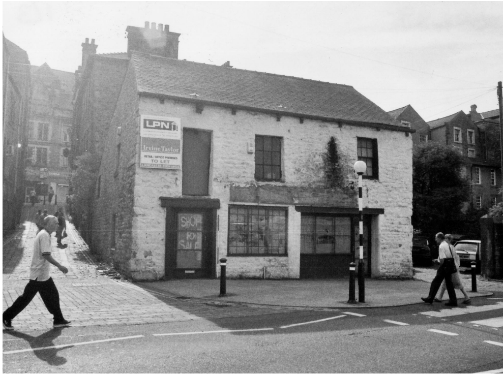
Plate 5: The front (north) external elevation
