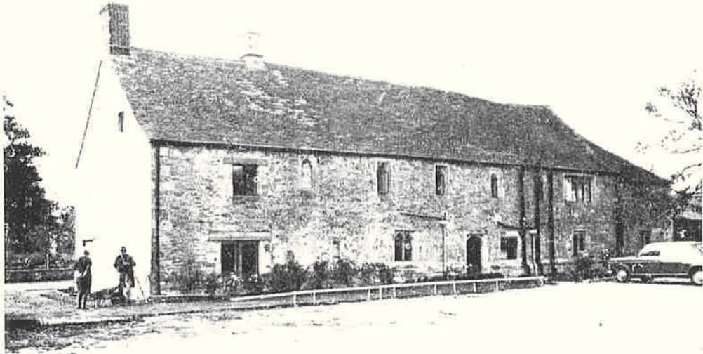
A : Minchery Farm, Littlemore : Dormitory range, from the east, showing the windows of the cells on the first floor (22-26 on plan). Photo : P. S. Spokes
