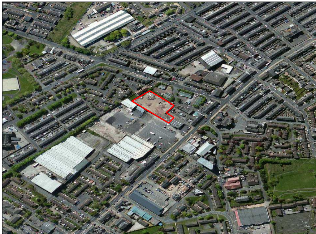
Plate 1: Aerial view looking south across the study area
