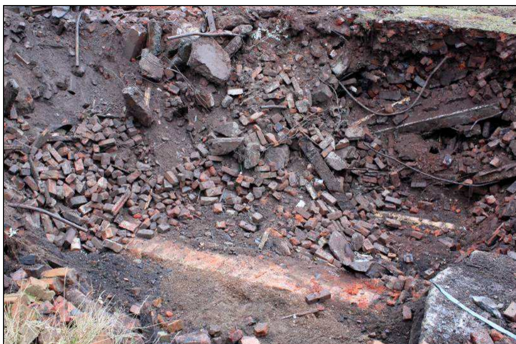
Plate 13: The extended excavation of Trench 1, looking east across the north-eastern wall of the engine house and the side of the refractory-brick lined flue to the rear
