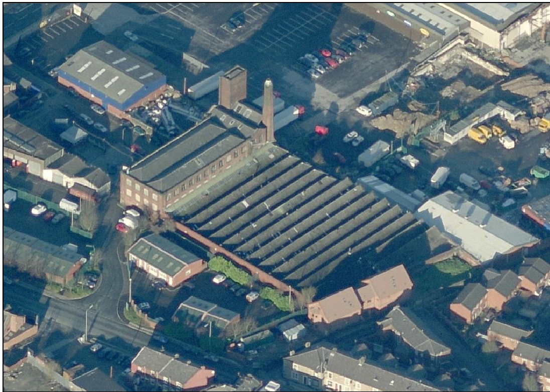
Plate 11: Aerial view of the mill shortly before demolition
