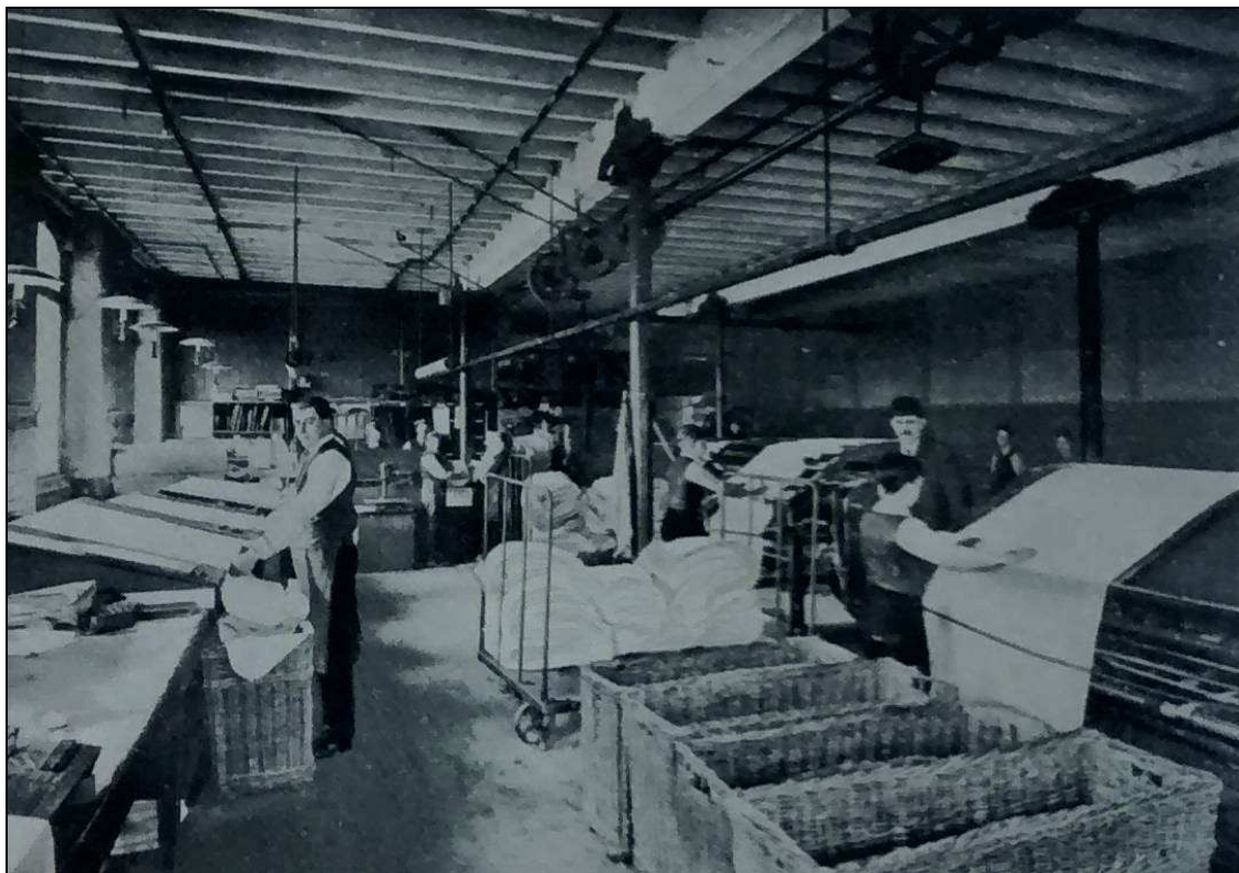
Plate 10: View of the cloth warehouse (from the Amalgamated Cotton Mills Trust Ltd, 1921)
