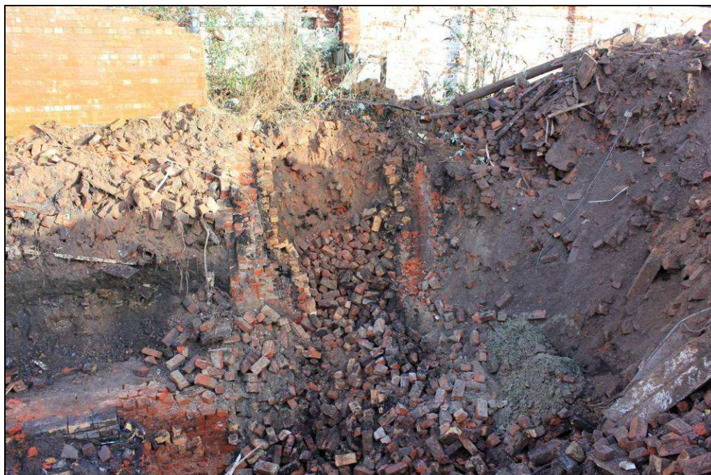
Plate 14: The remains of the demolished chimney stack, and the side wall of the flue
