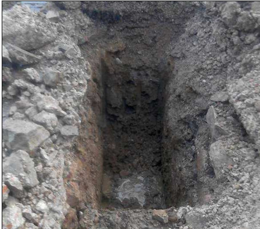
Plate 17: Trench 6, looking south-east
