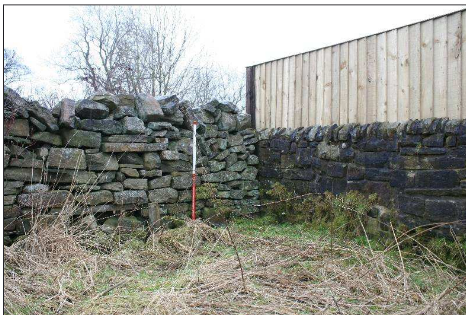
Junction between drystone wall (06) and cement mortar wall (07) wall, facing north-east
