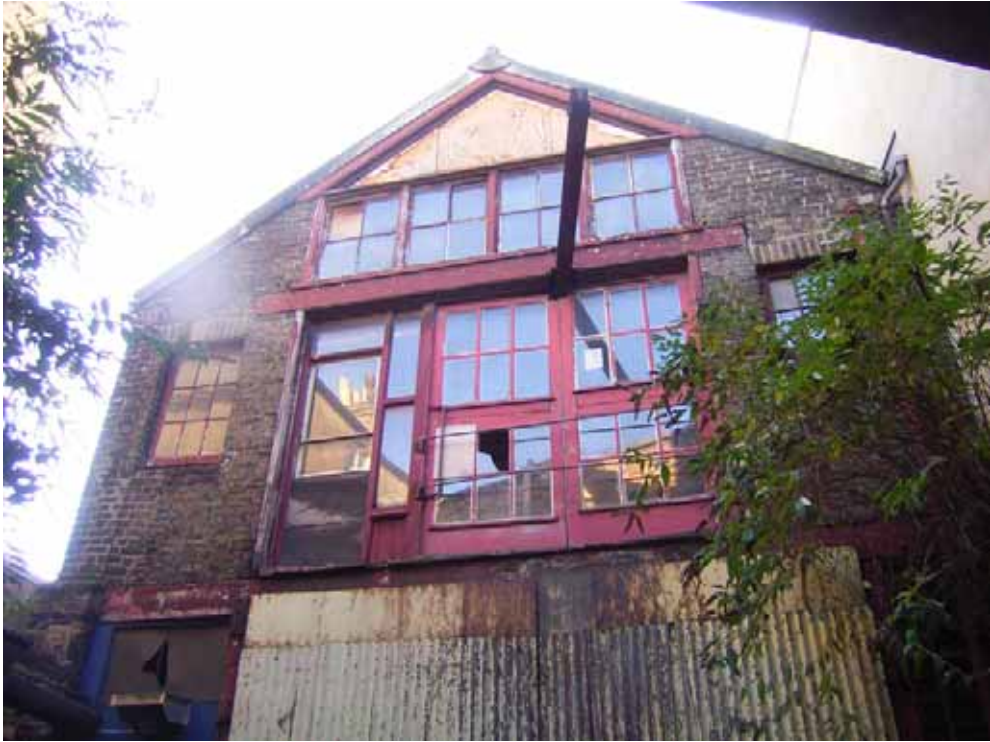
Glazed loading bay in north elevation
