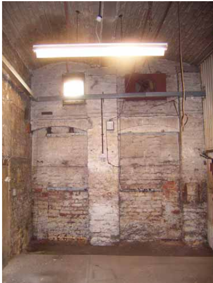
Detail of south interior elevation
