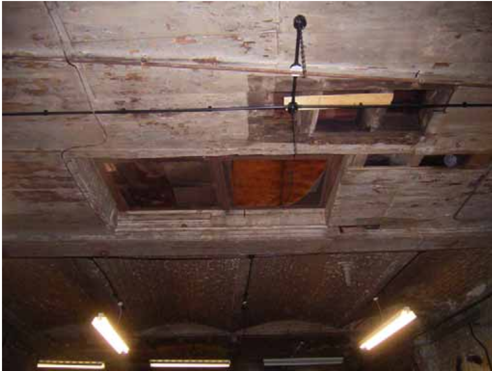
Ceiling detail, facing south
