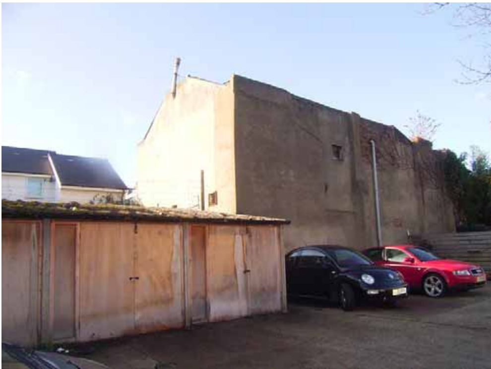
South and east elevations
