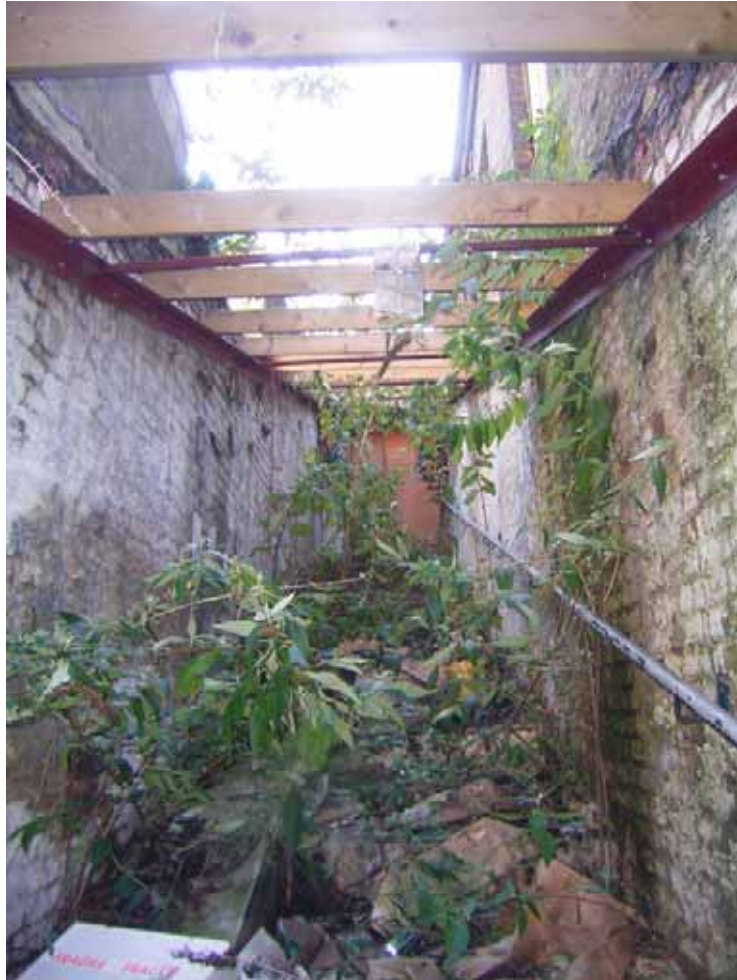
Exterior stairway on east wall
