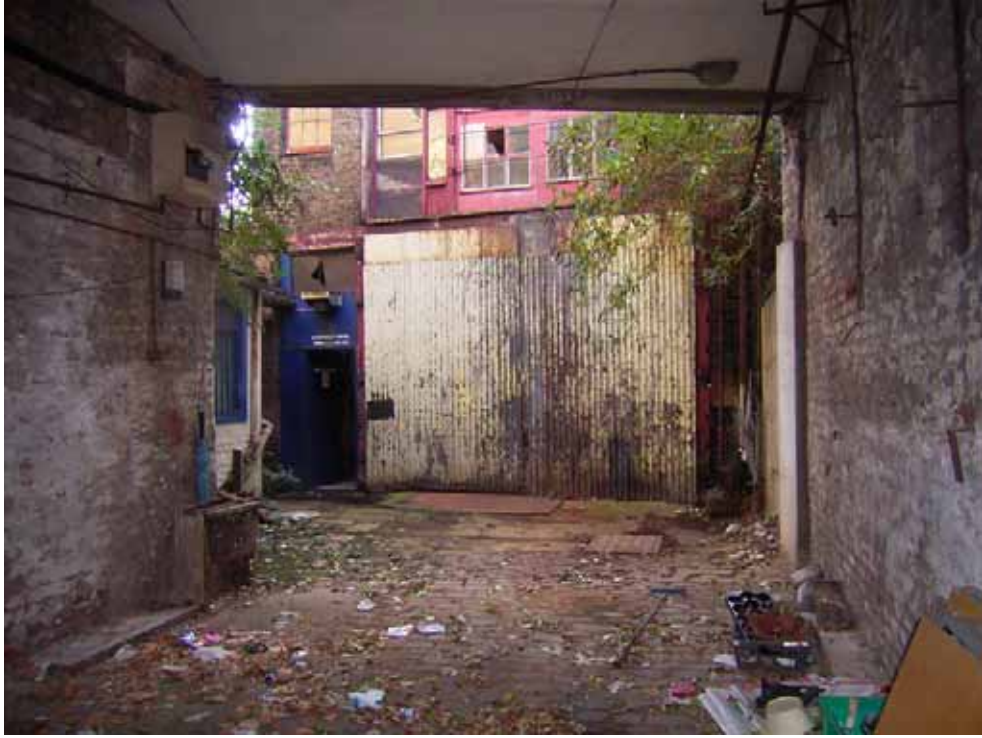
Entrance in north elevation
