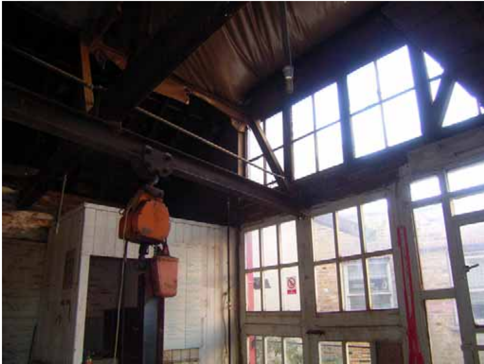
RSJ and winch attached to roof structure in north room on first floor
