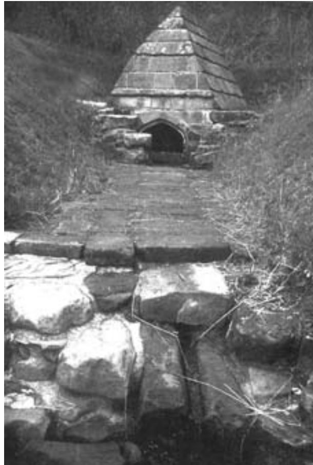
Above: This medieval well house in North Yorkshire shows how the Eynsham well house may have looked, with the spring head protected by a stone chamber, and the water lead away in a stone channel. Photograph by Patrick Greene.
