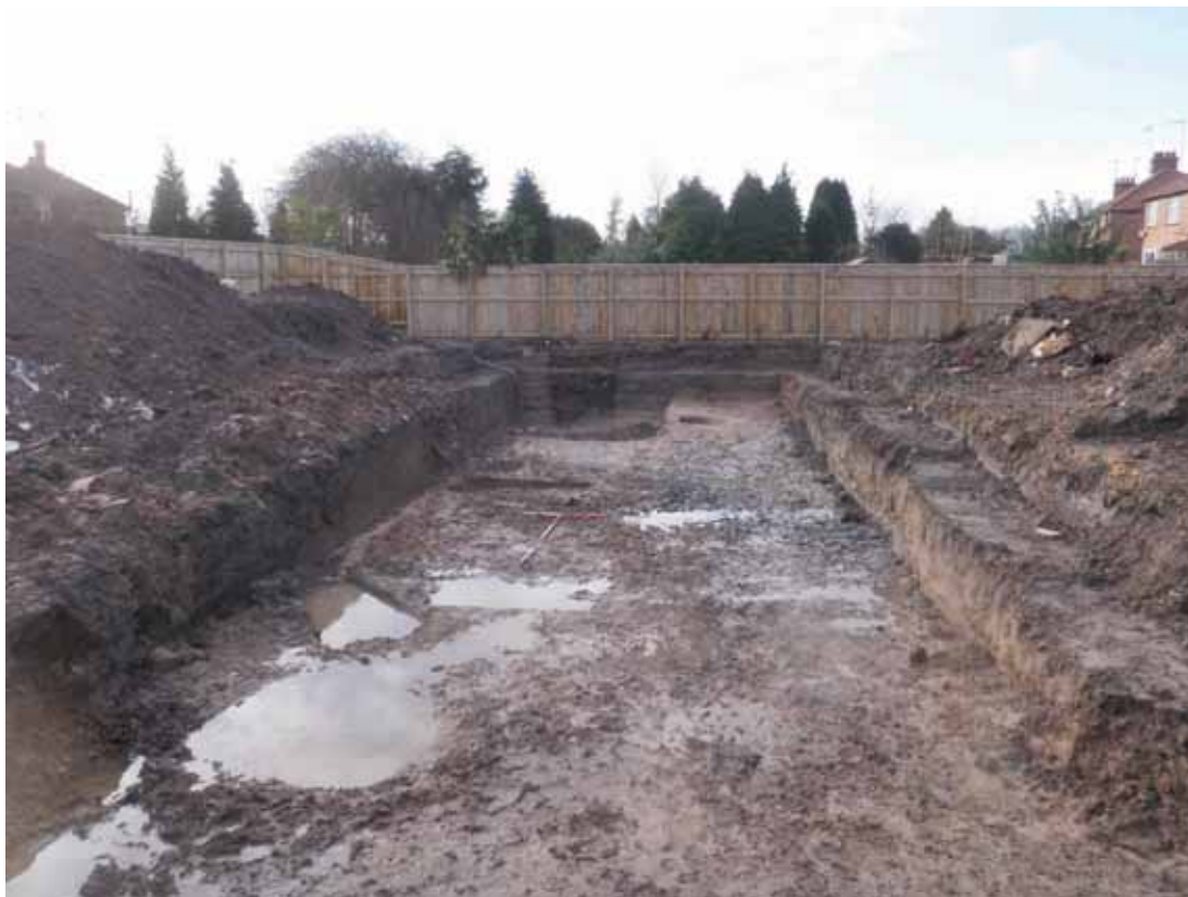
Plate 1: General view of the excavation area, facing south-west
