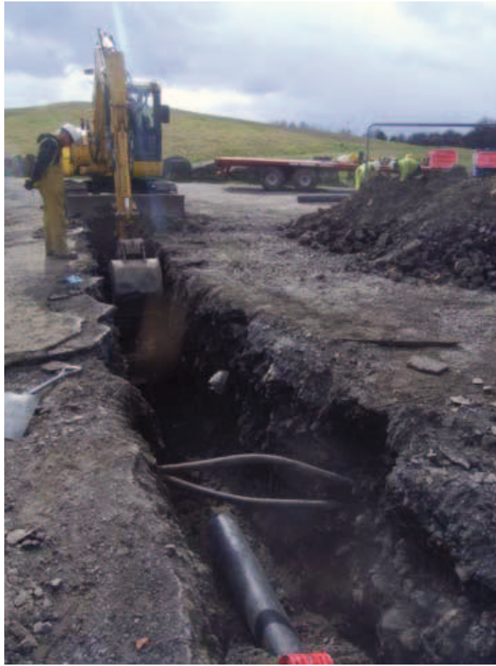
Plate 15: Pipe trench within White Rock car park
