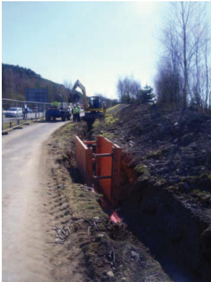
Plate 16: Pipe trench along the A4217
