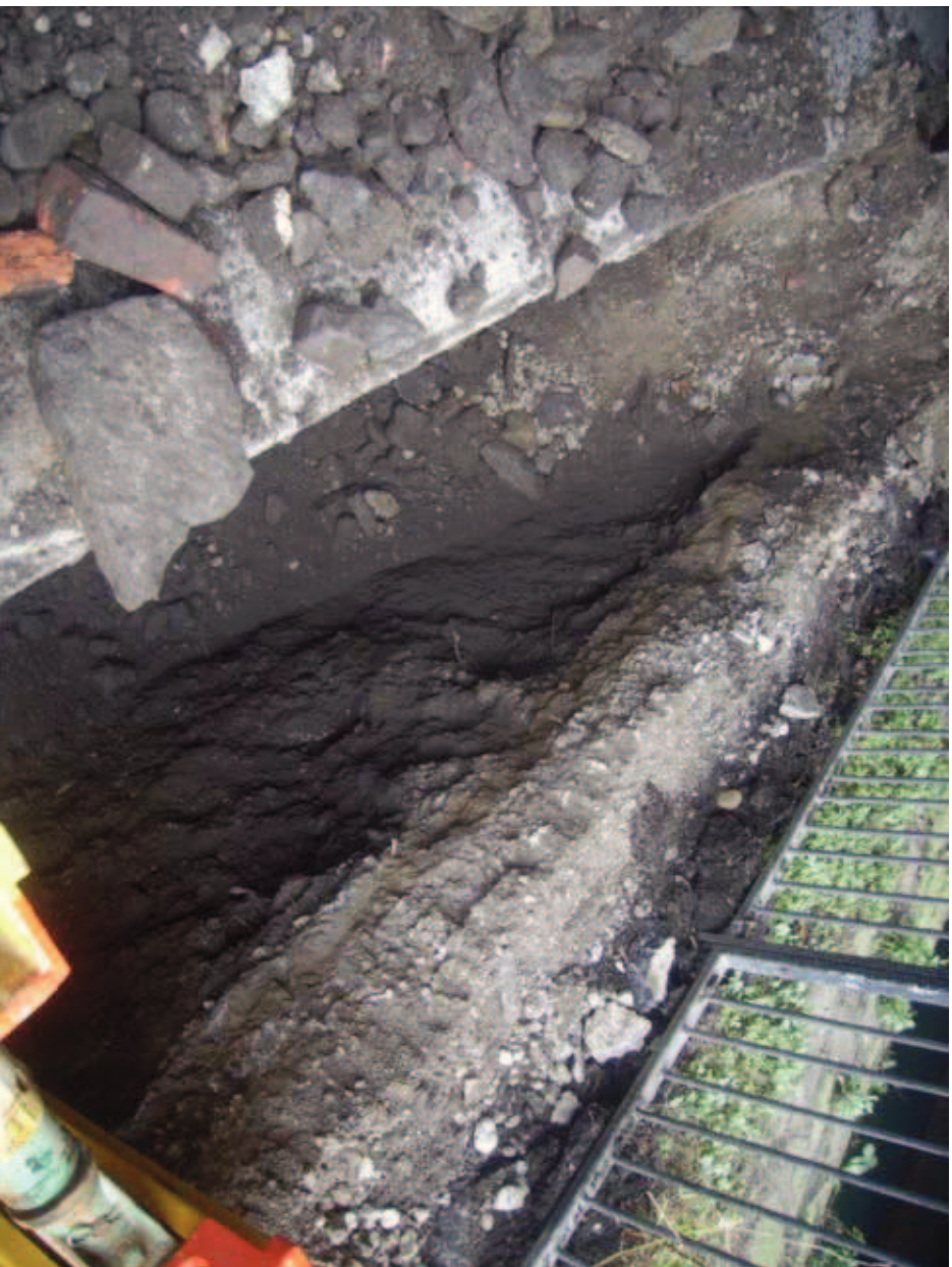
Plate 14: Deposits below road bridge
