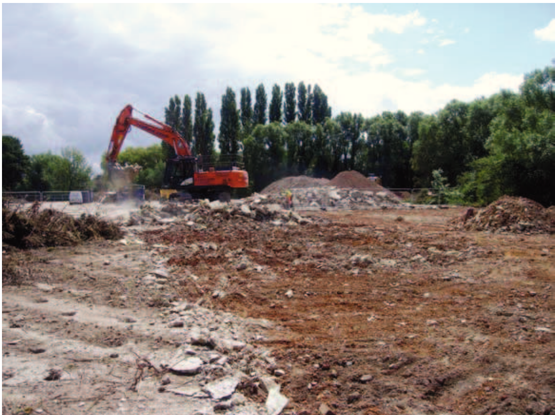
Plate 2: Removal of concrete slab
