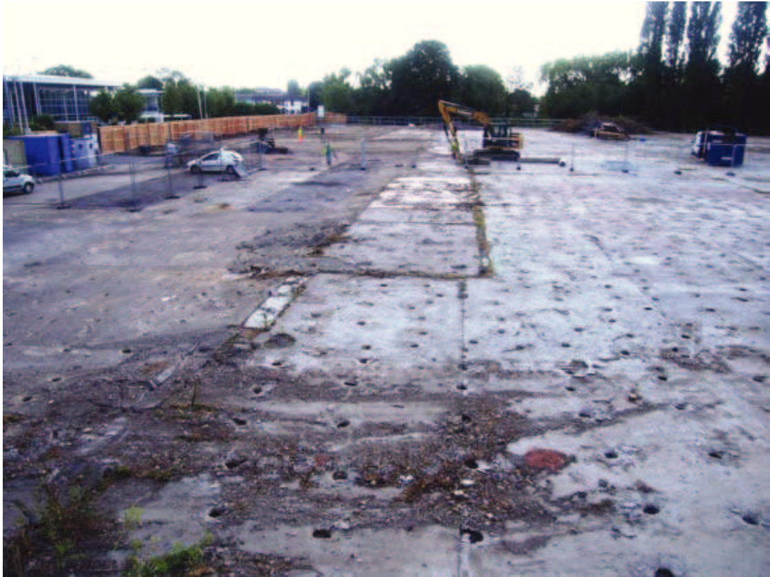
Plate 1: General shot, pre-concrete removal
