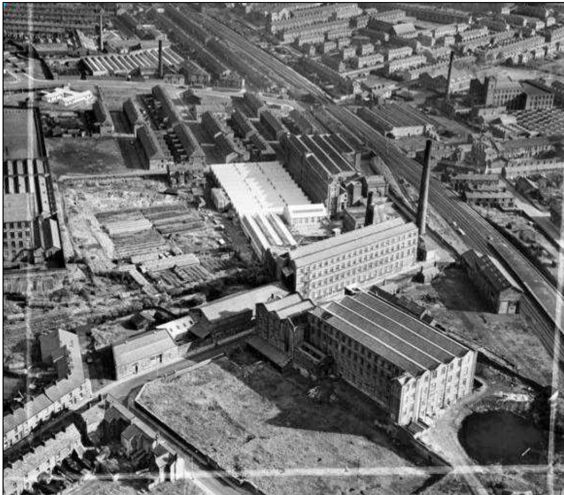
Plate 4: Aerial view across Mill Hill in 1950, showing the Mill Hill Cotton Works and Waterfall Mill to the rear. Part of the present study area is visible in the bottom left corner
