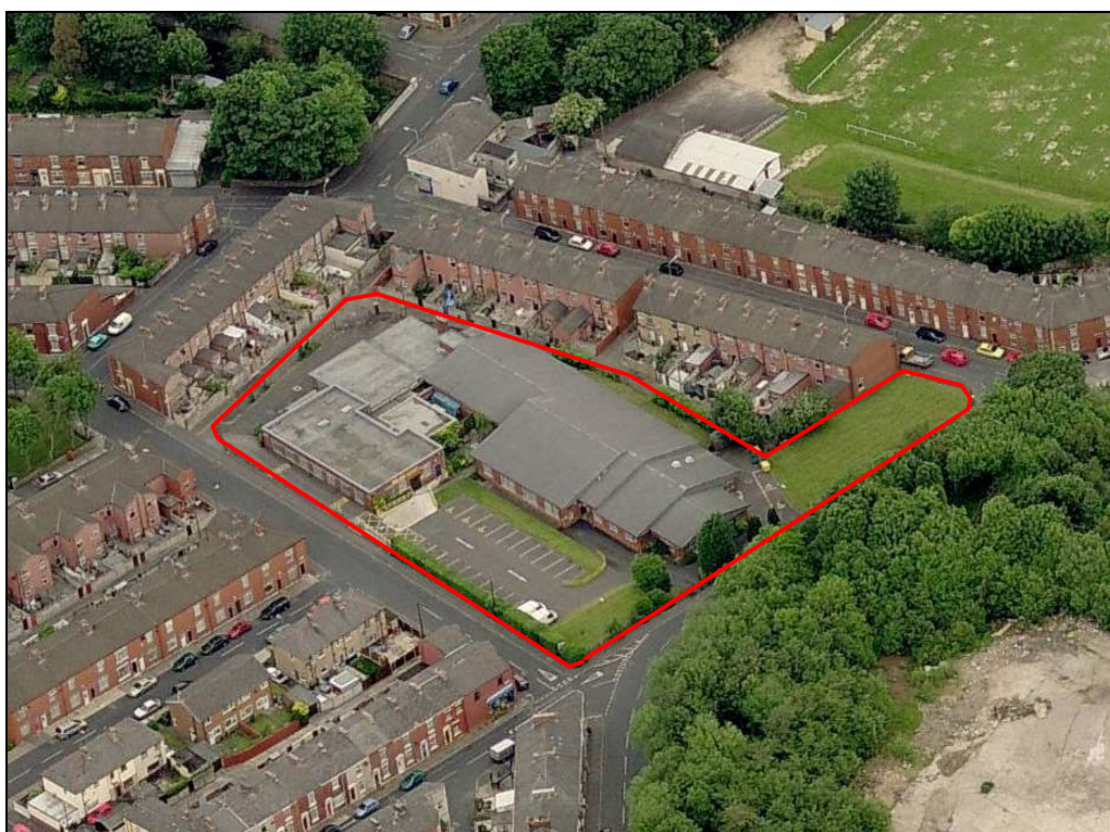
Figure 1: Recent aerial view of the development site
