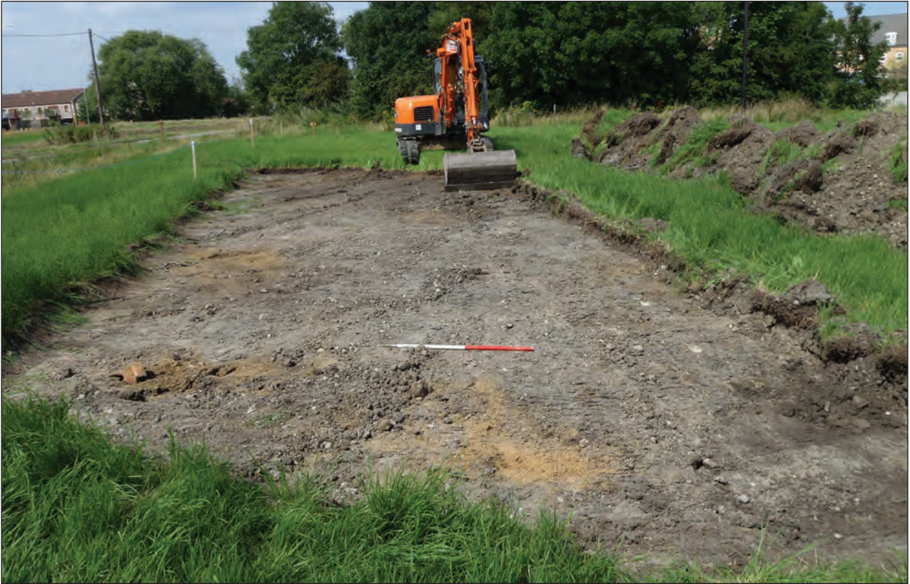
Plate 1: Field A topsoil strip, looking North
