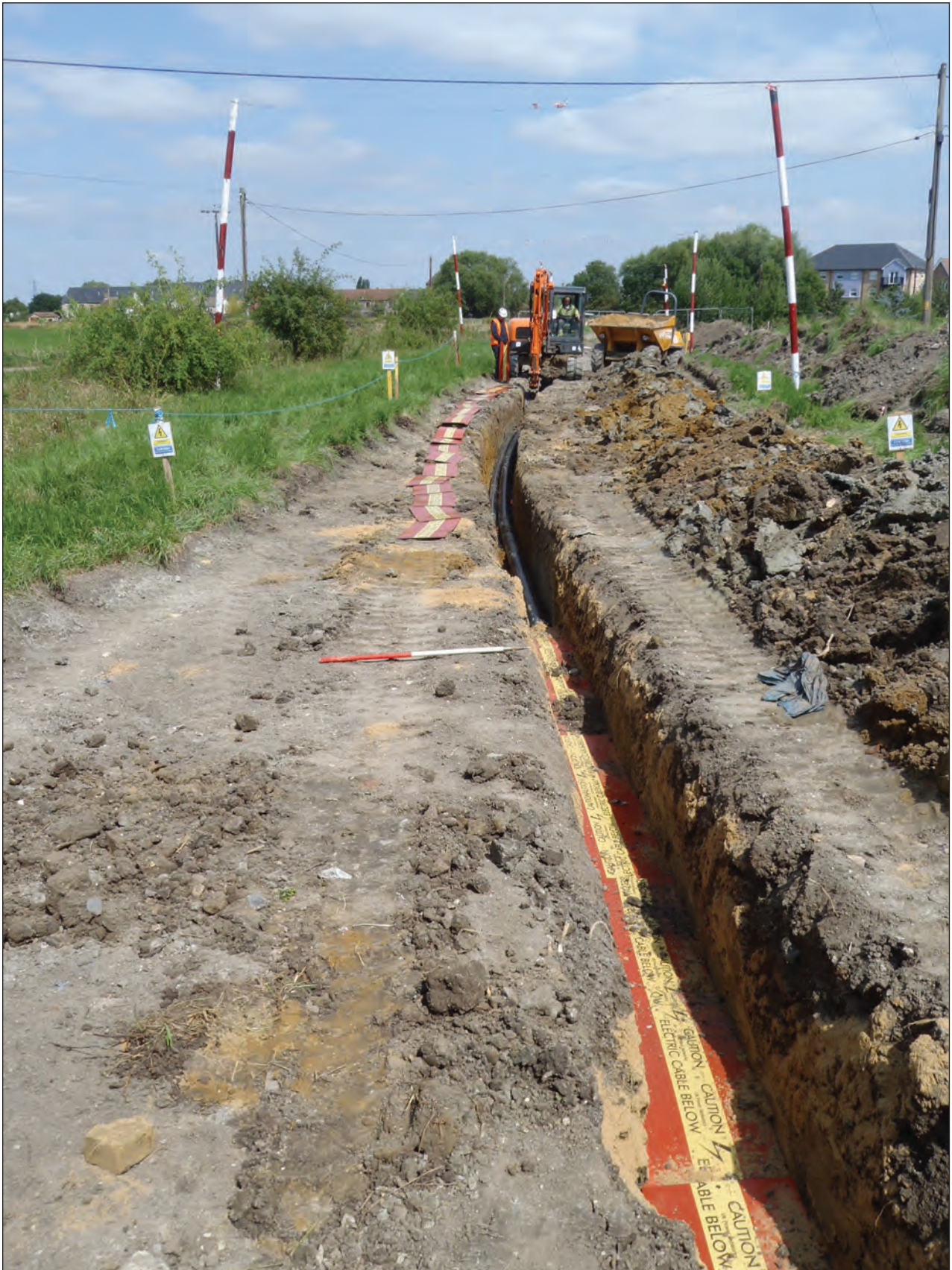
Plate 2: Field A cable trench, looking North
