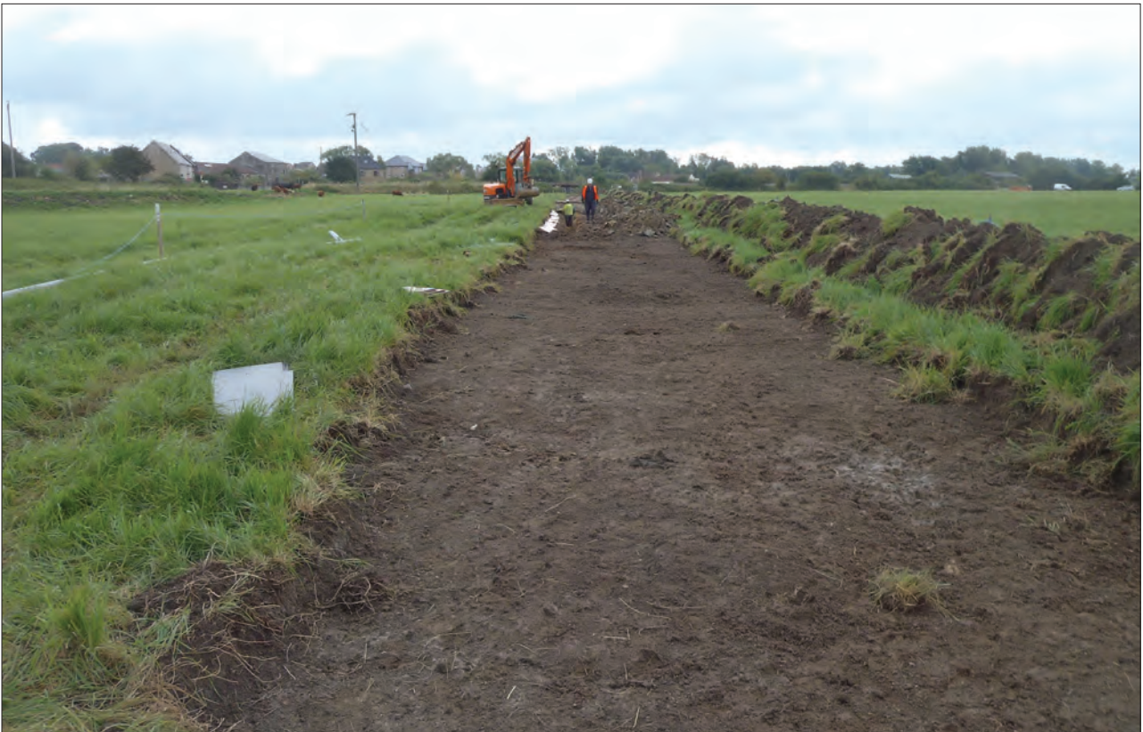
Plate 5: Field C topsoil and cable trench, looking East
