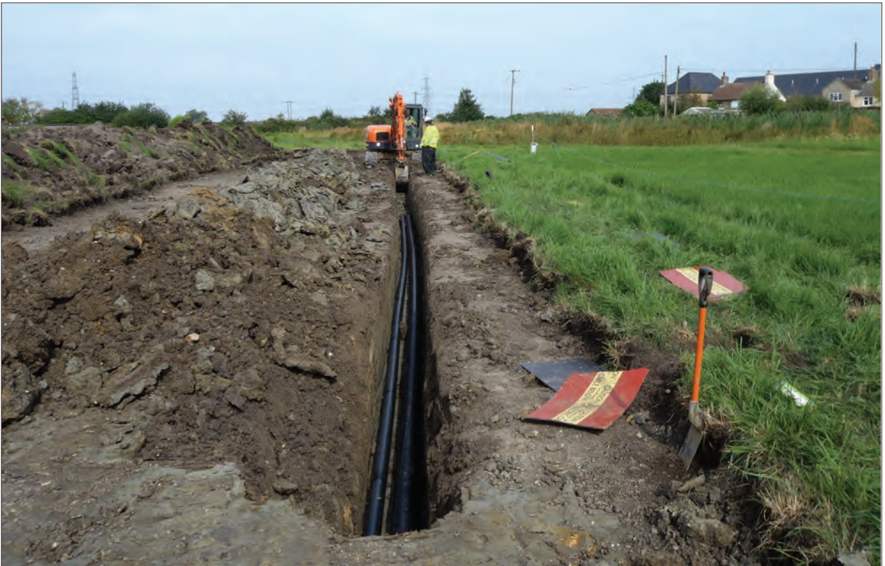
Plate 4: Field B cable trench, looking west
