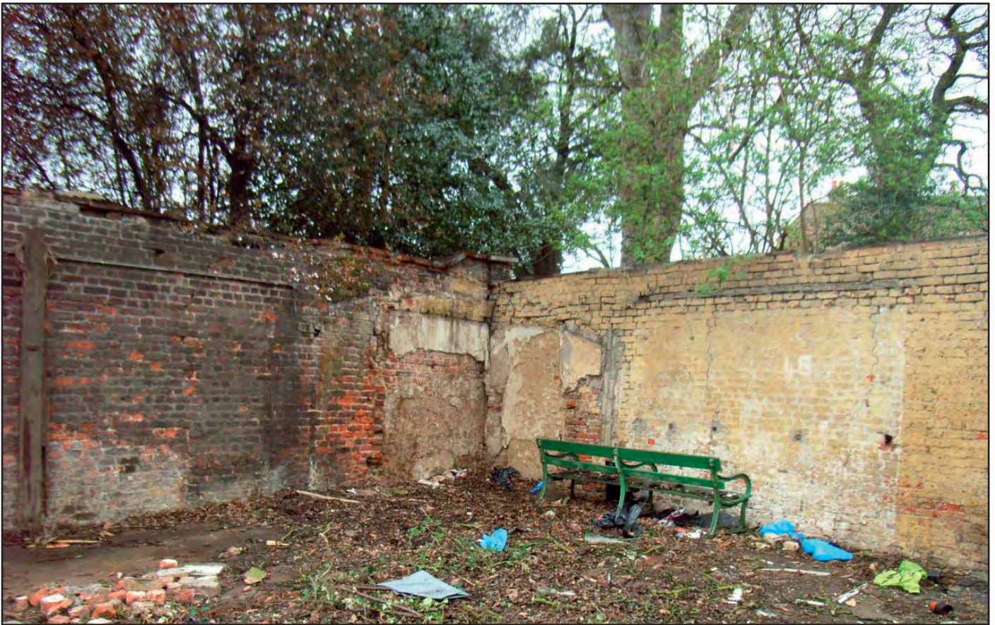
Plate 3: South corner between Walls 2a and 3
