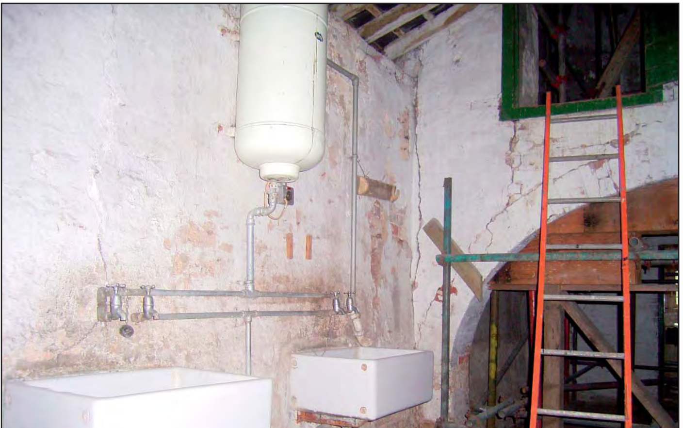
Plate 24: NW ground floor room in Dovecote
