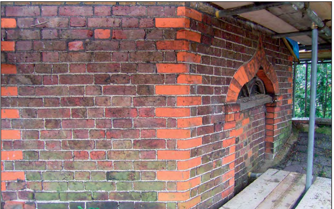
Plate 16: 1st floor of Dovecote
