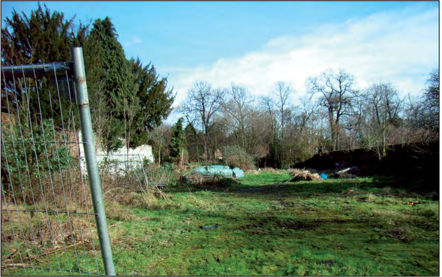
Plate 1: General view of Kitchen Garden from SW prior to start of works
