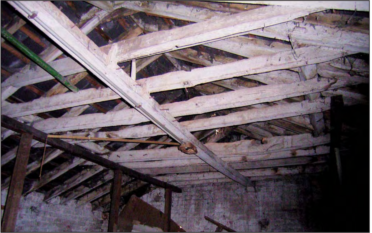
Plate 39: Roof in Granary
