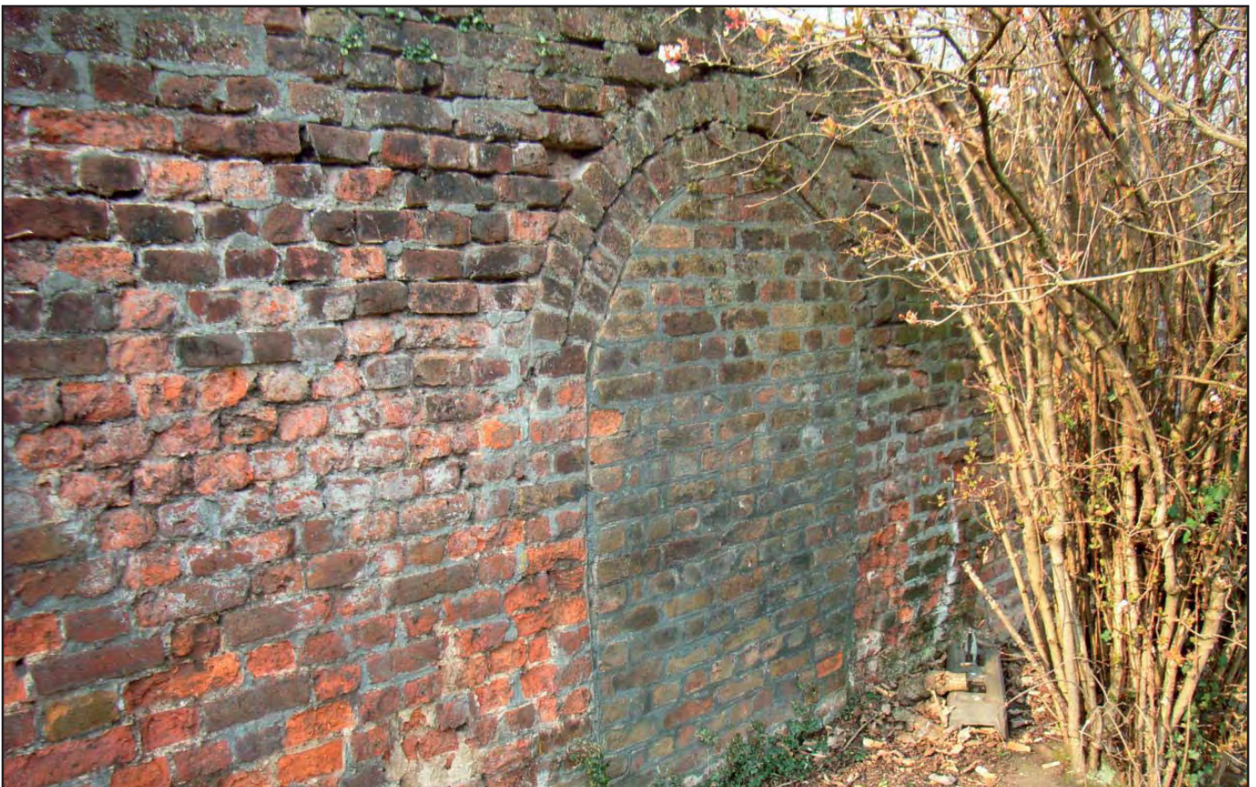
Plate 6: Infilled doorway in Wall 4
