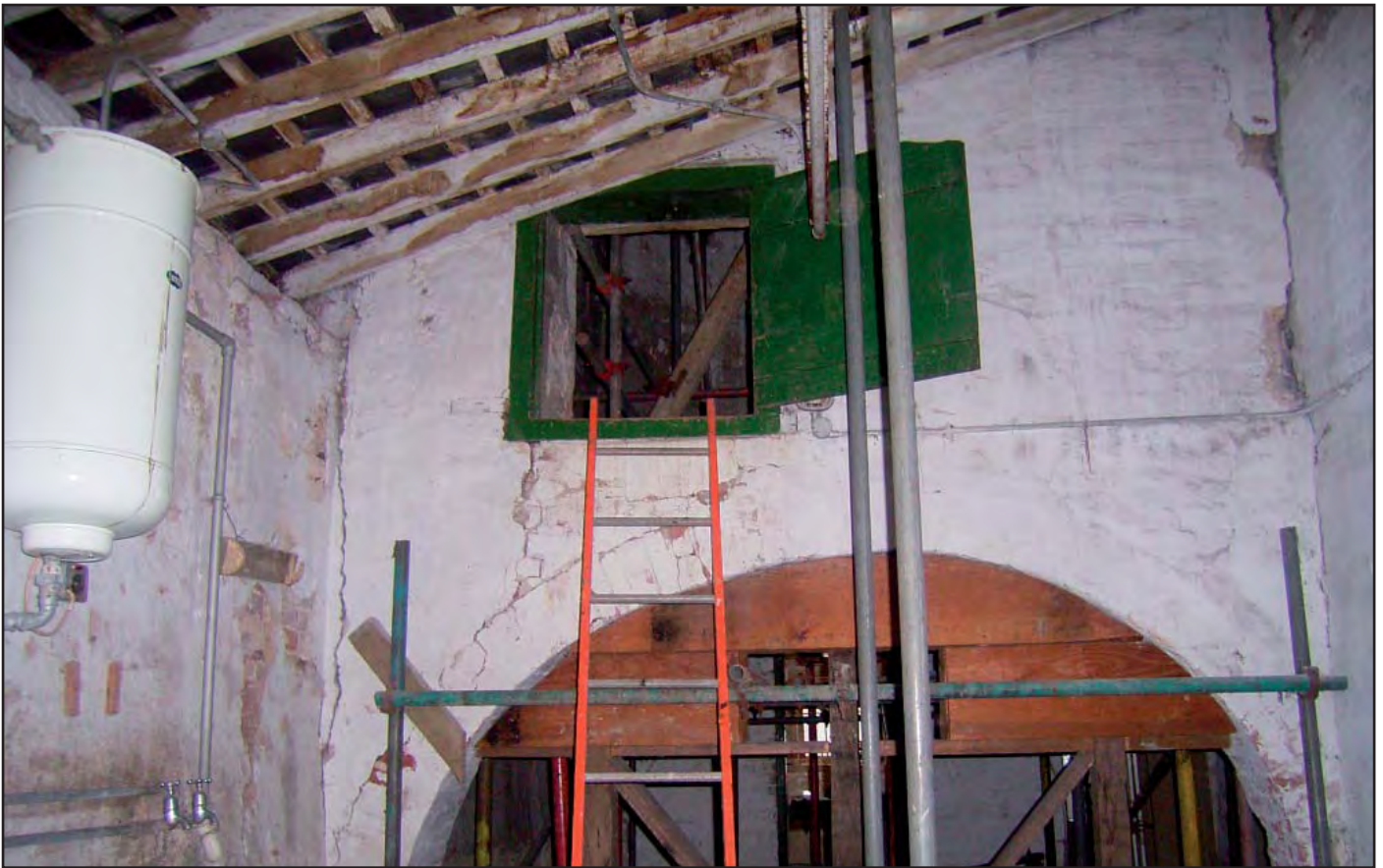
Plate 23: NW ground floor room in Dovecote
