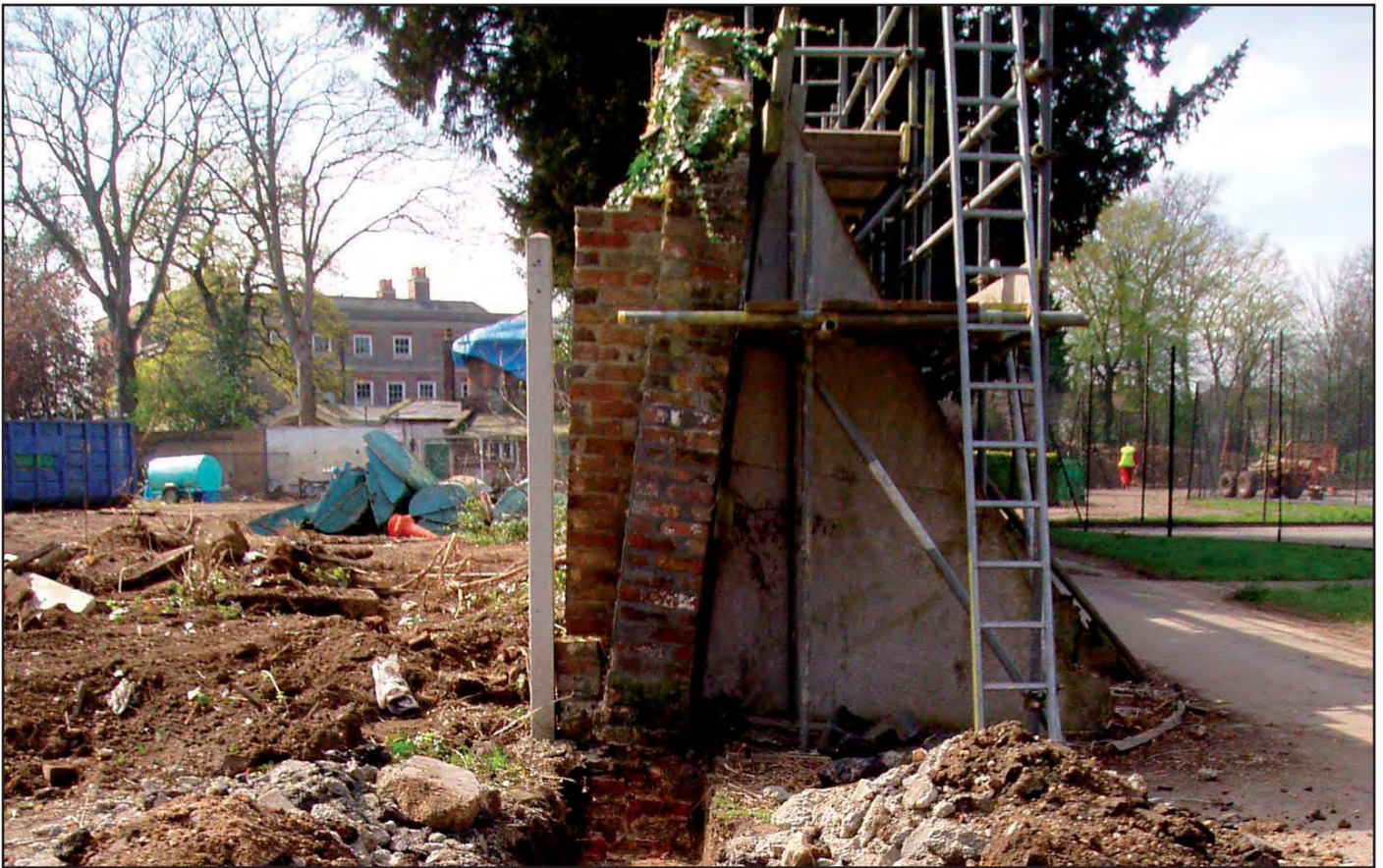
Plate 47: Footings from NE end wall of Wall 1 exposed during works
