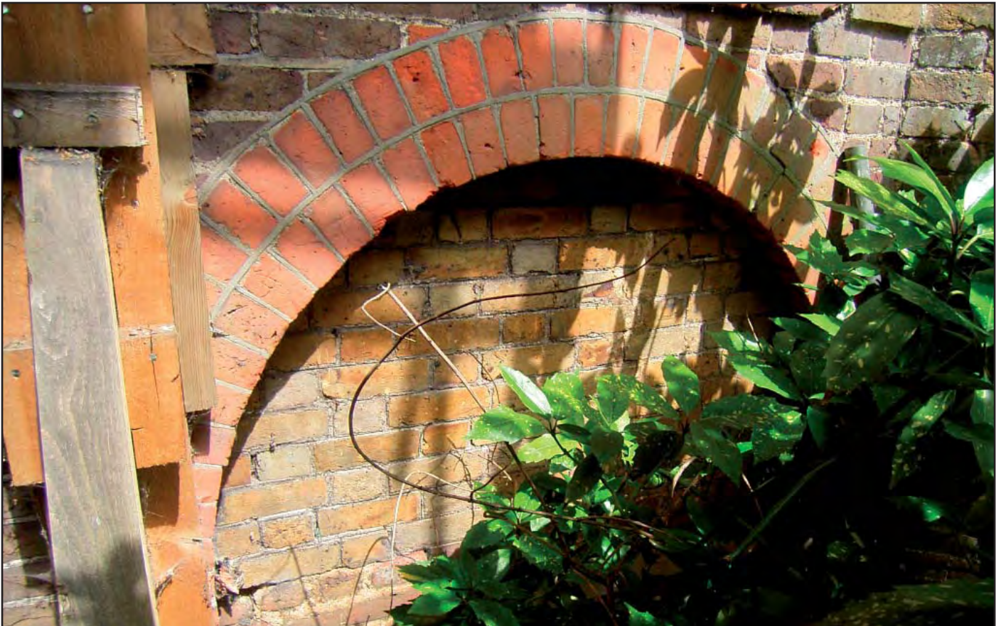
Plate 14: Blocked arch in SW elevation of Dovecote
