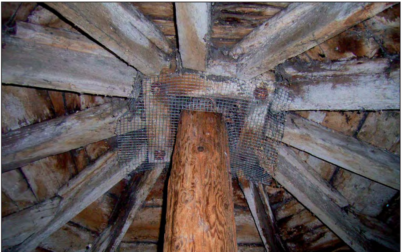
Plate 28: Apex of roof in Dovecote
