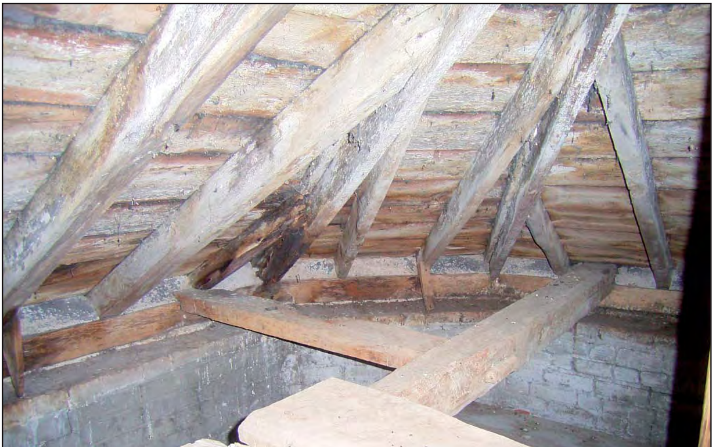
Plate 30: Roof detail in Dovecote
