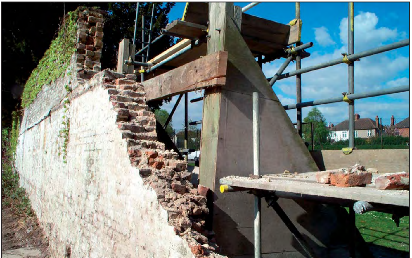
Plate 8: Wall 1 (NE end) during reconstruction
