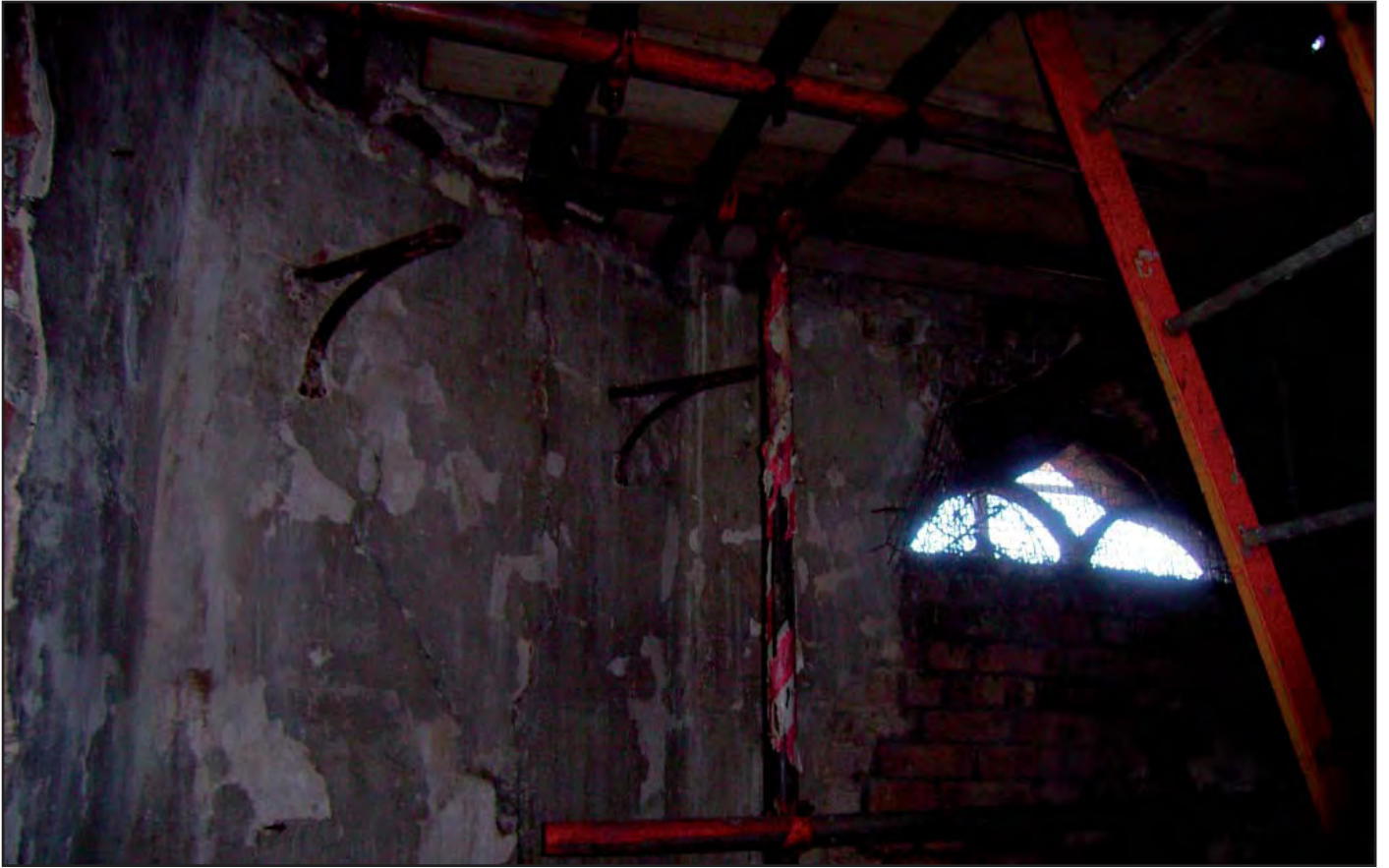
Plate 25: 1st floor of Dovecote
