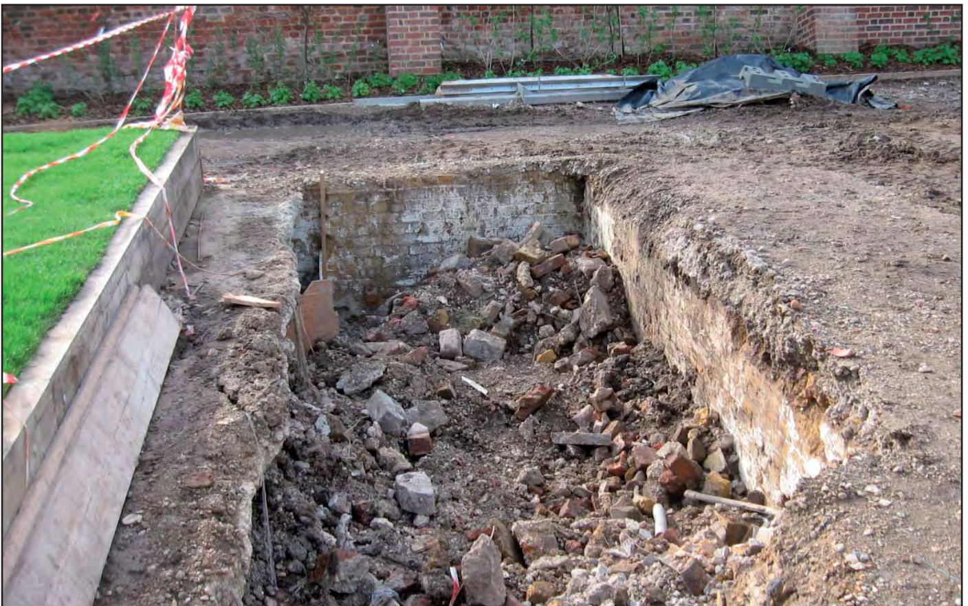
Plate 50: Brick (later 19th century) walls exposed in Tree Pit 4 in Kitchen Garden
