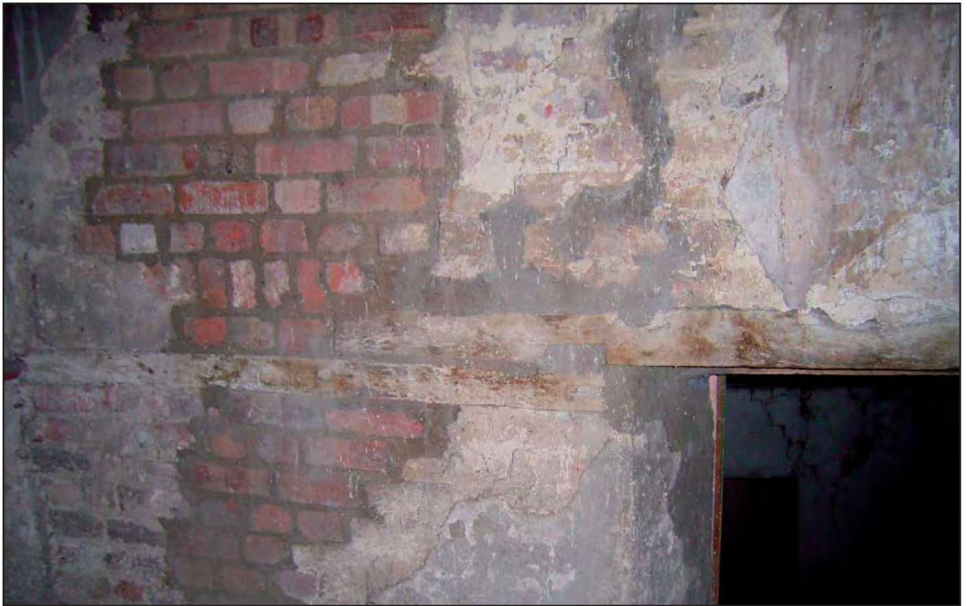
Plate 29: Repairs in internal walls of Dovecote
