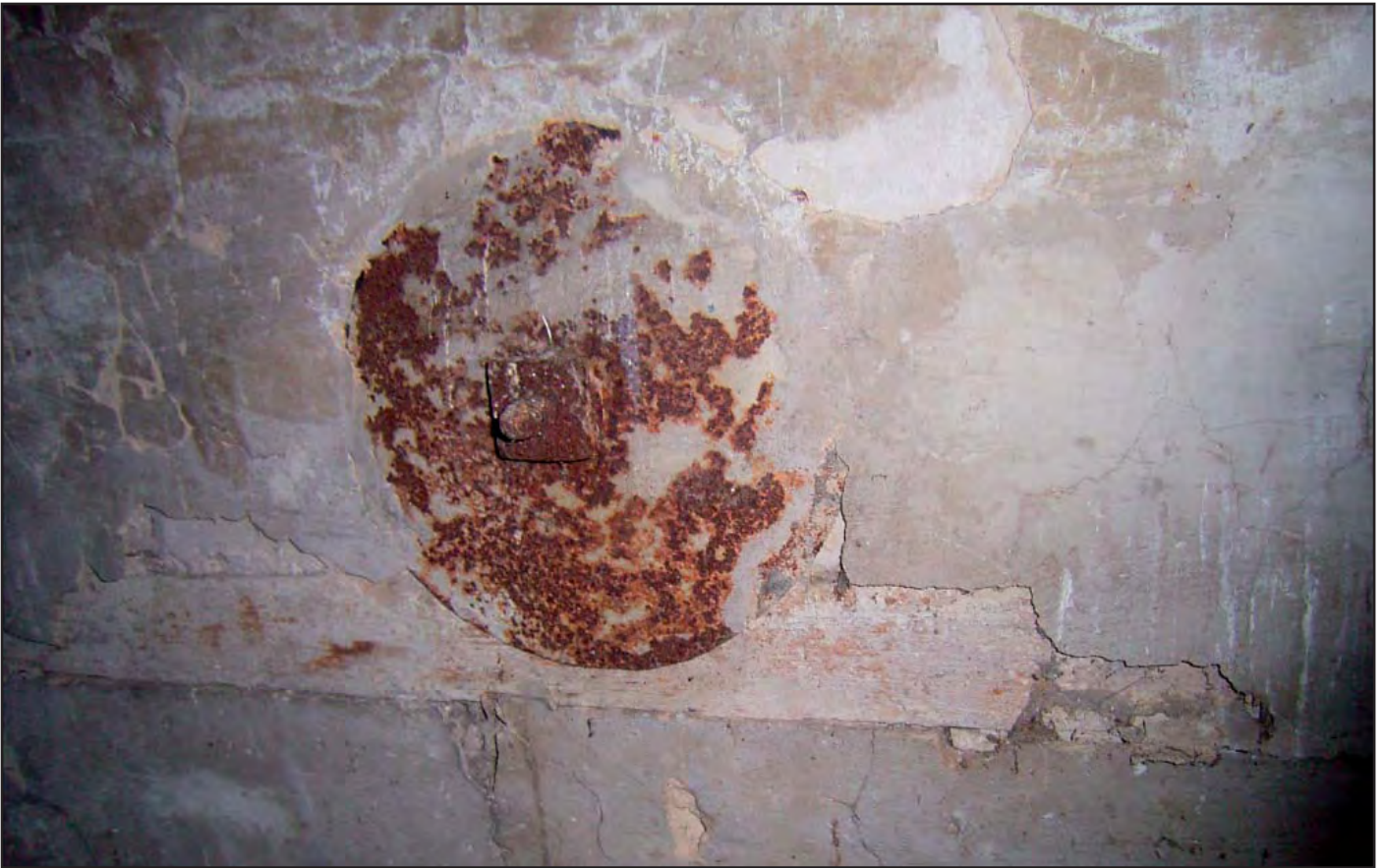
Plate 22: Tie bar plate in Dovecote
