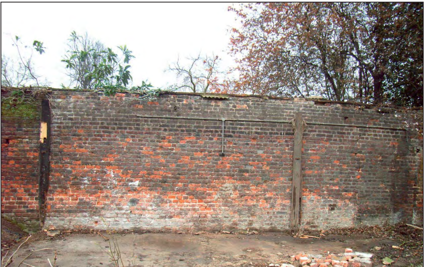
Plate 2: NW side of Wall 2a showing evidence of former lean-to's
