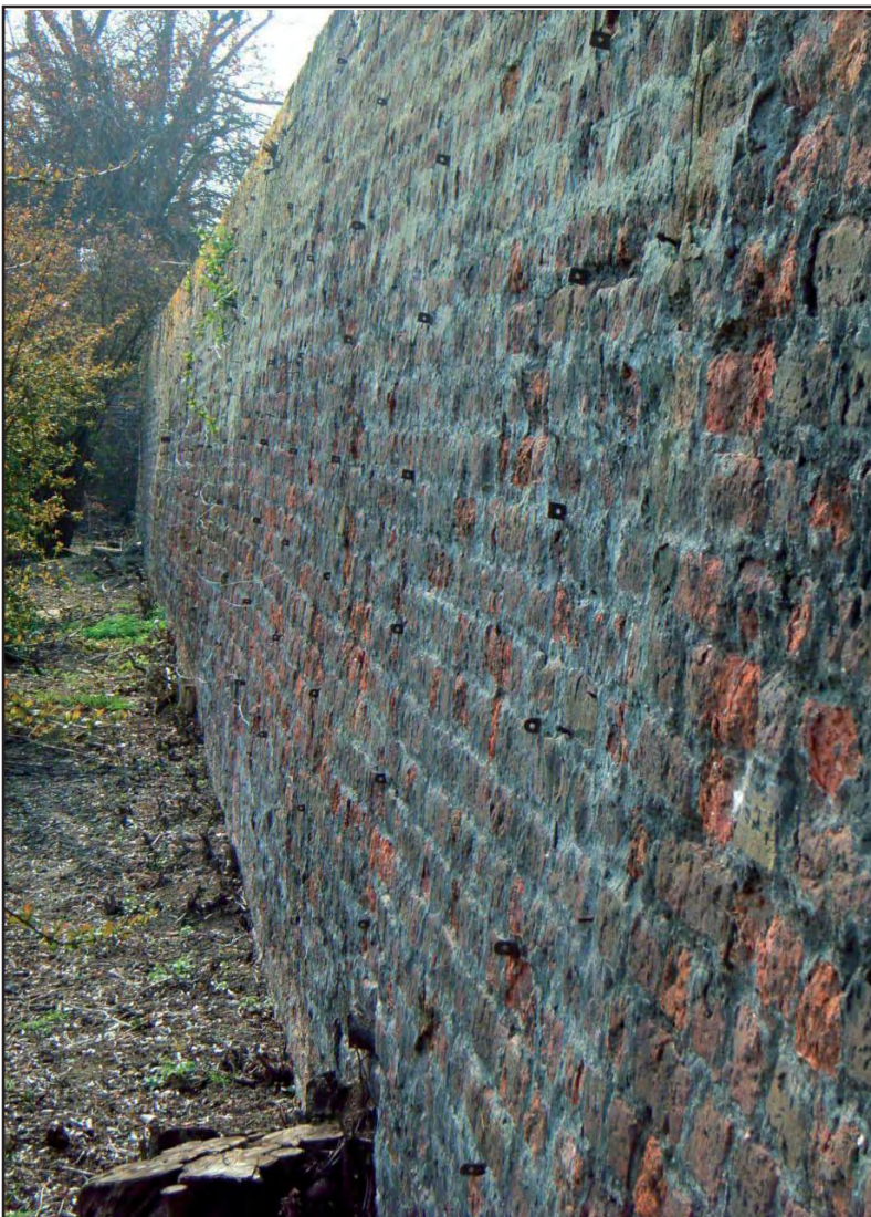
Plate 4: SE side of Wall 2 showing ash-rich repointing
