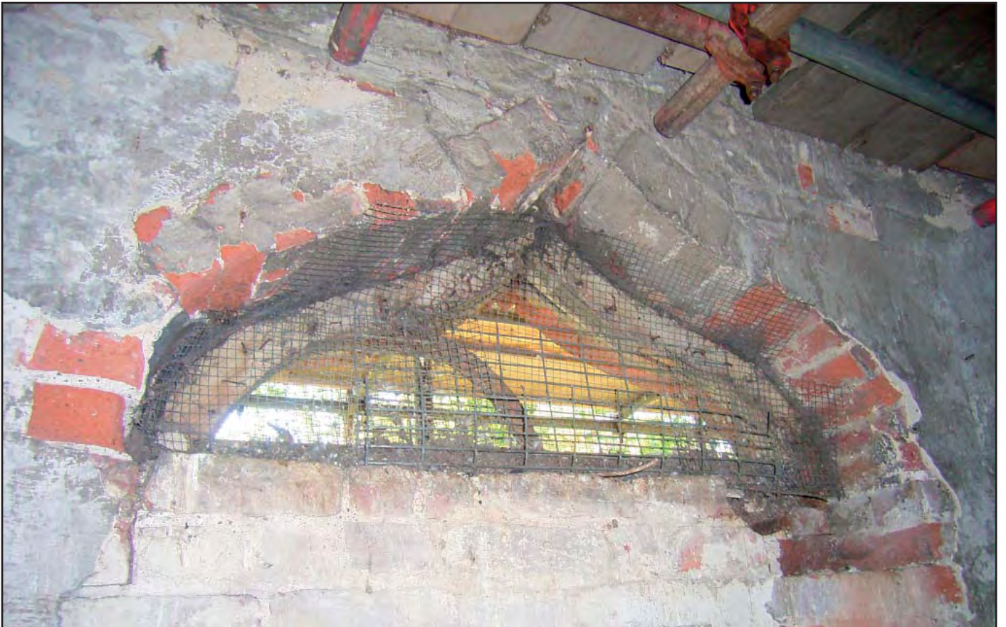
Plate 26: Window arch in Dovecote
