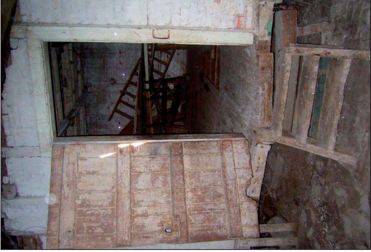
Plate 36: Access door to Granary
